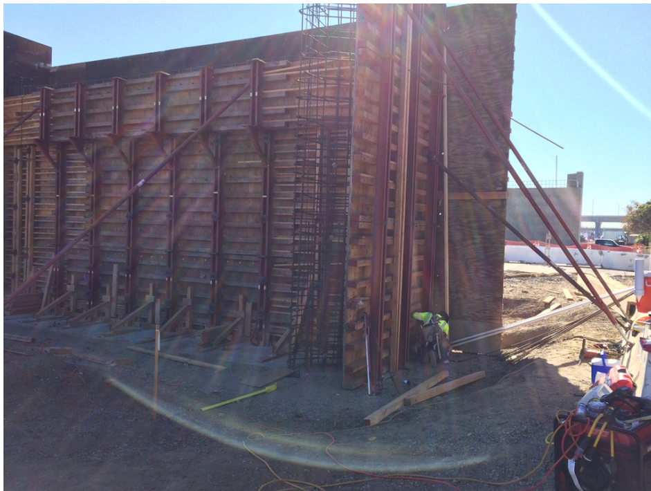
111 TH STREET BRIDGE - Abutment 2 formwork installation.
