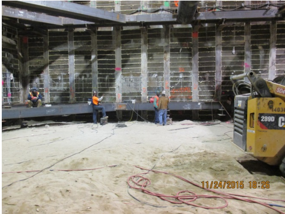
LEIMERT PARK STATION – Tier 2 wale welding operation.
