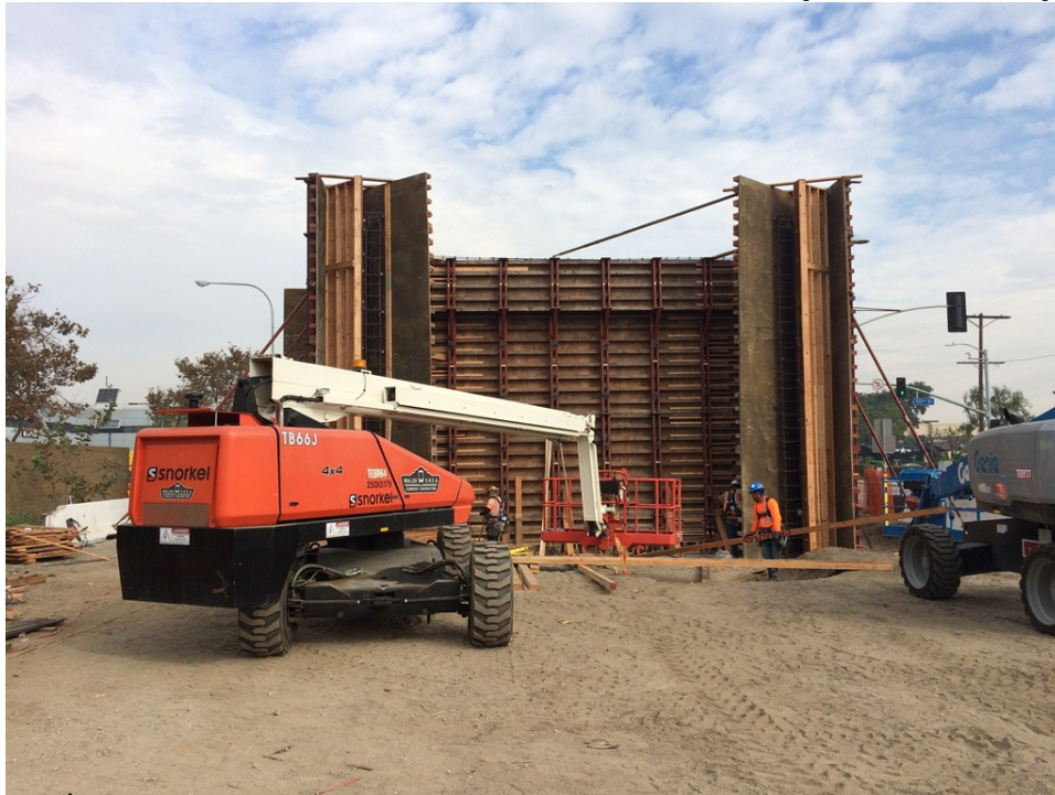
111 th UNDERPASS - Abutment 1 and return wall formwork and concrete placement.
