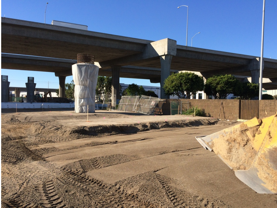
GREENLINE UNDERPASS - Subgrade compaction for falsework erection.
