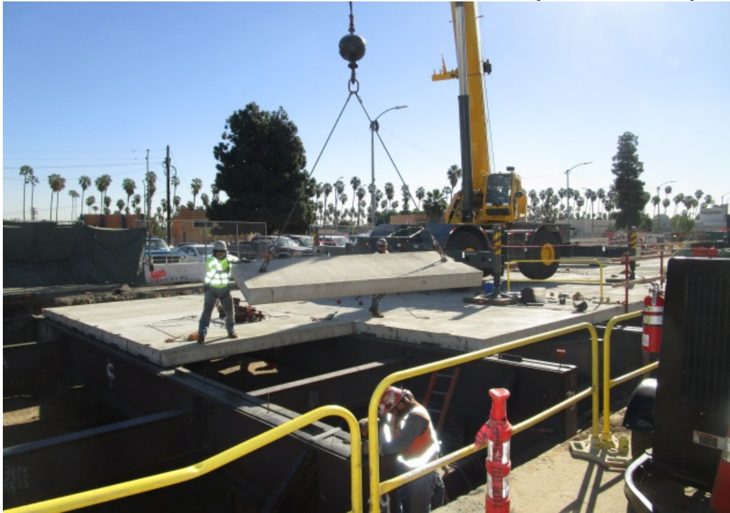
UG4 – Setting precast deck panels looking south.
