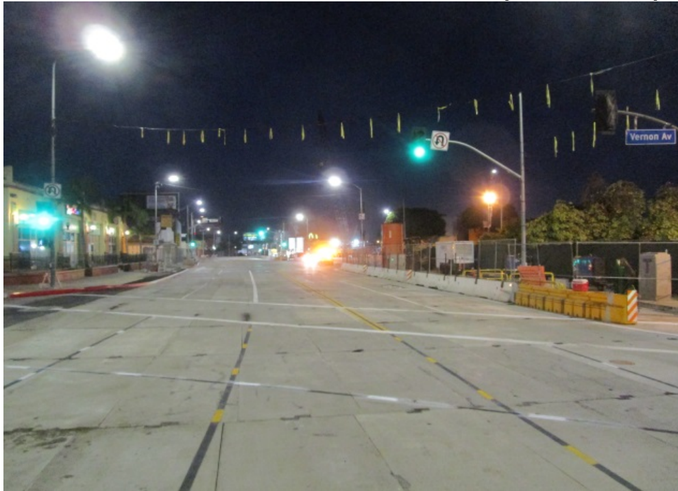
UG4 – Decking complete; looking north from Vernon.
