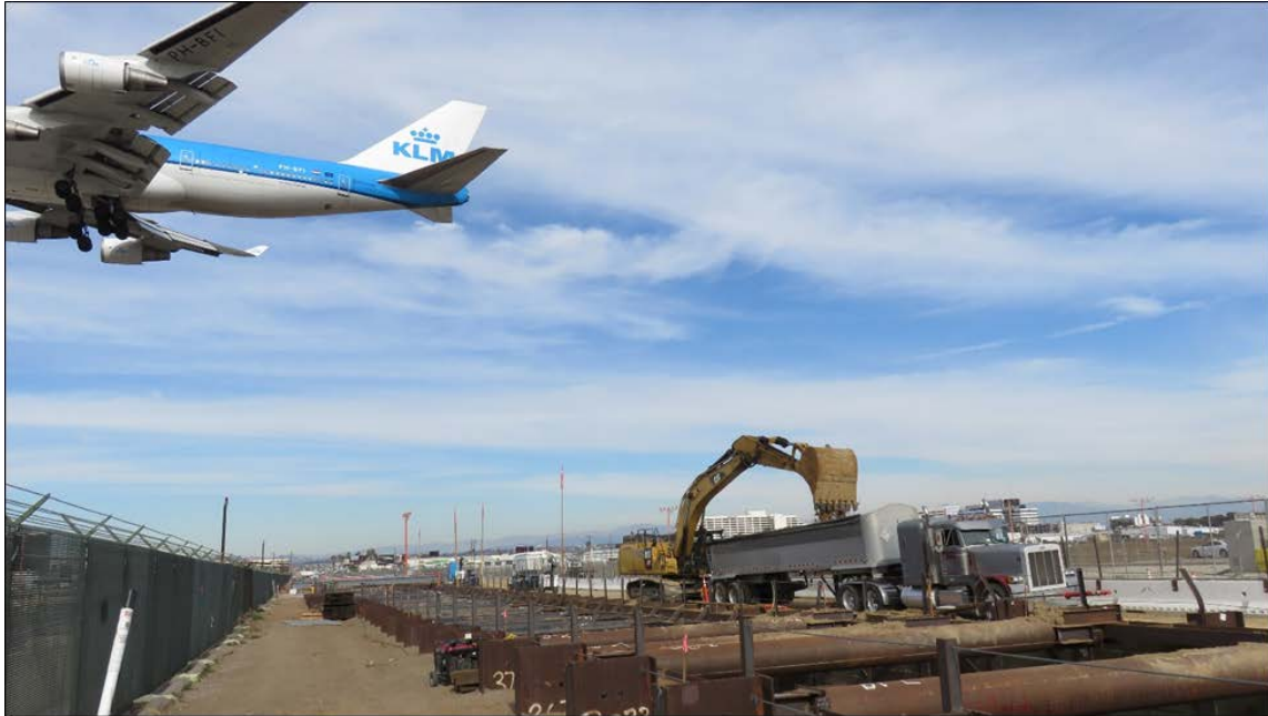
UG1 – On-going excavation.
