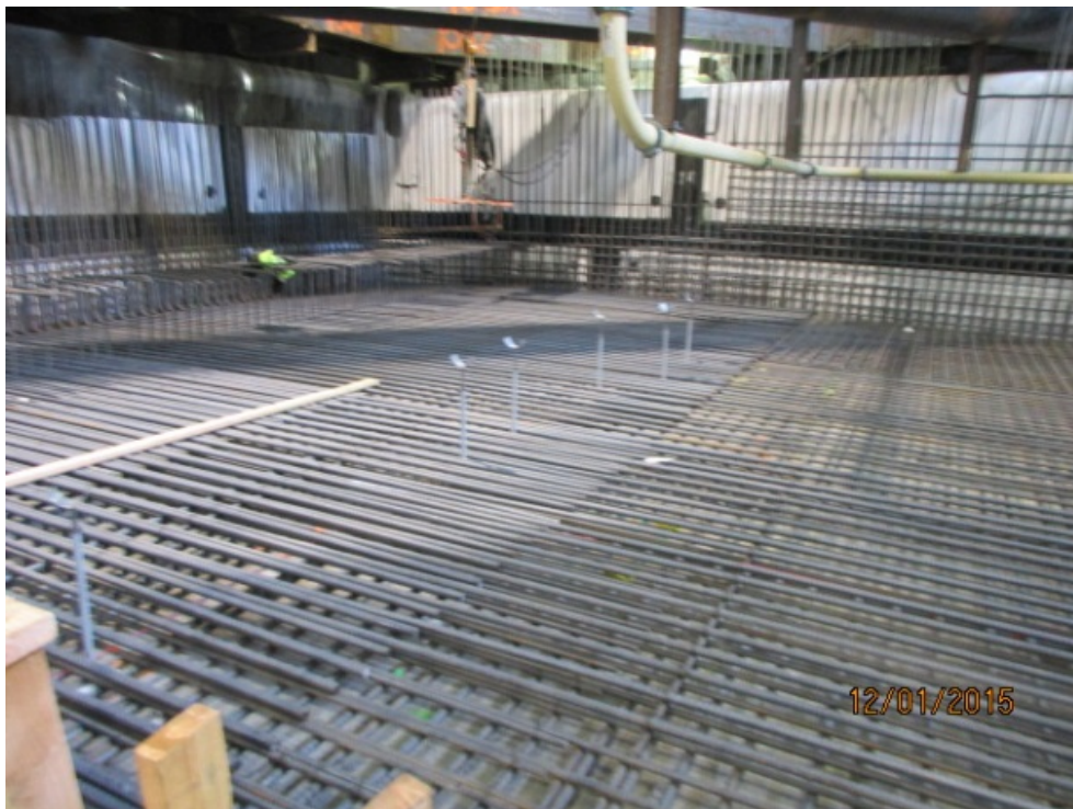
EXPO/CRENSHAW STATION – Installation of rebar for invert slab.
