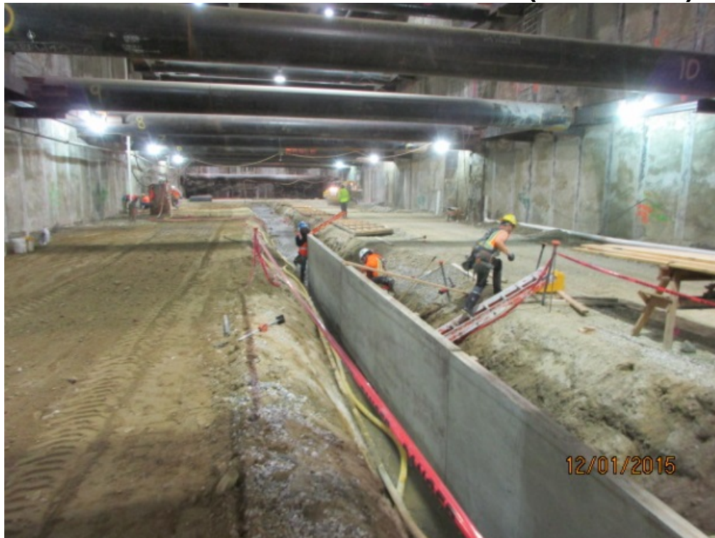
EXPO/CRENSHAW STATION – Installation of wall forms for center trench mud slab.
