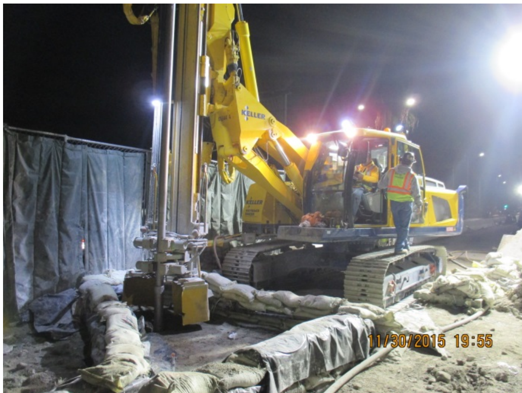
CROSS PASSAGE 2 – Jet grouting operation.
