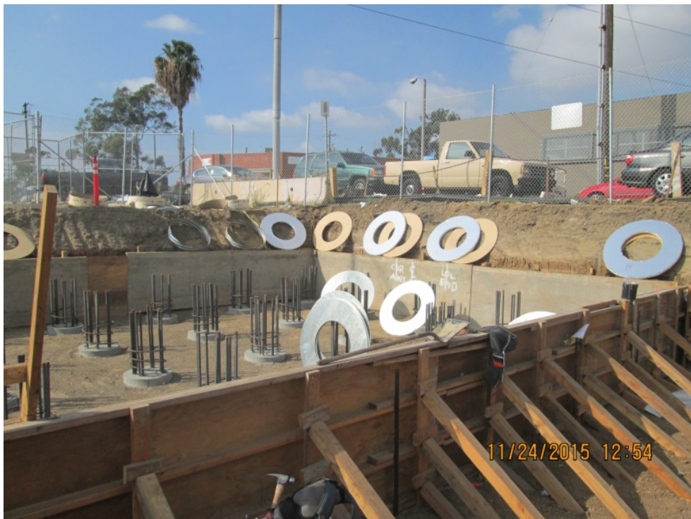
I-405 BRIDGE - Abutment 5 footing construction ongoing.
