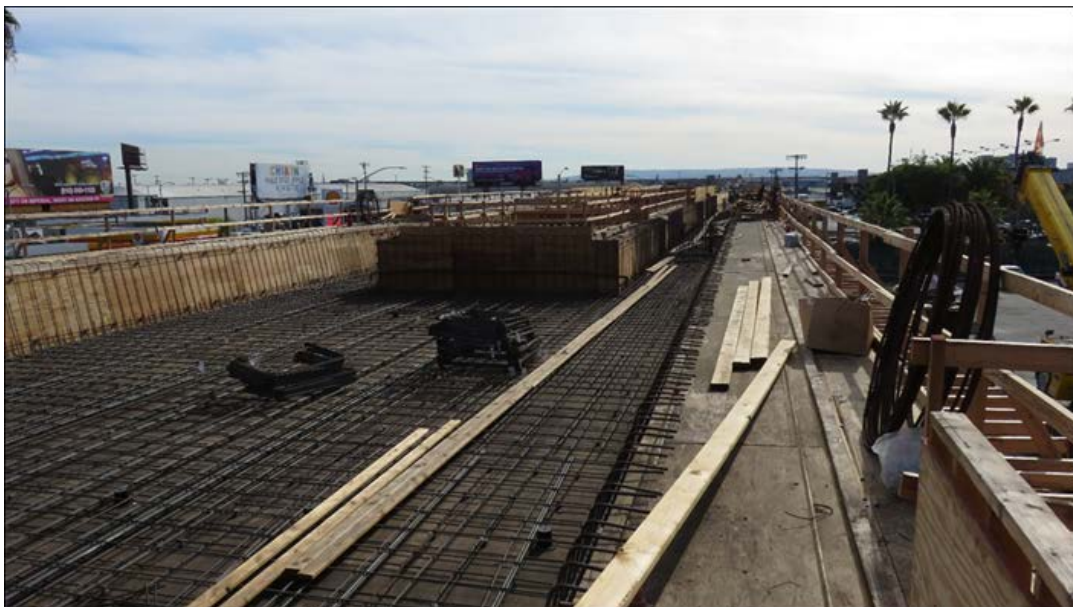
CENTURY BRIDGE – Super Structure Rebar.
