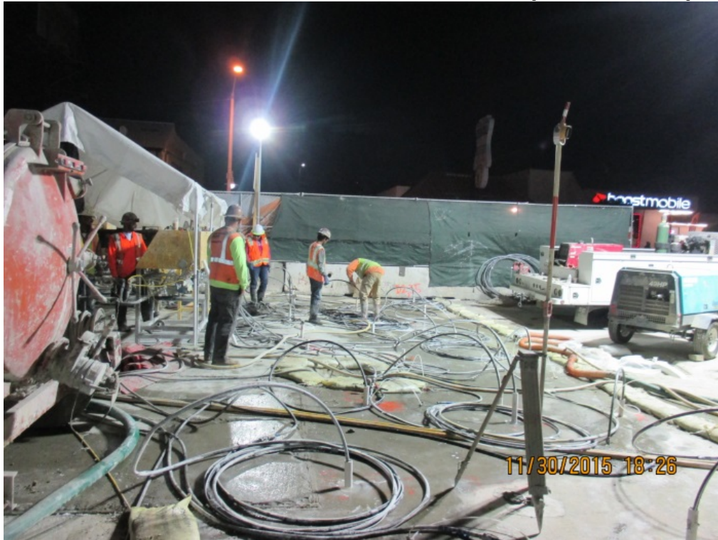
MARTIN LUTHER KING STATION – TBM Break-out chemical grout operations.
