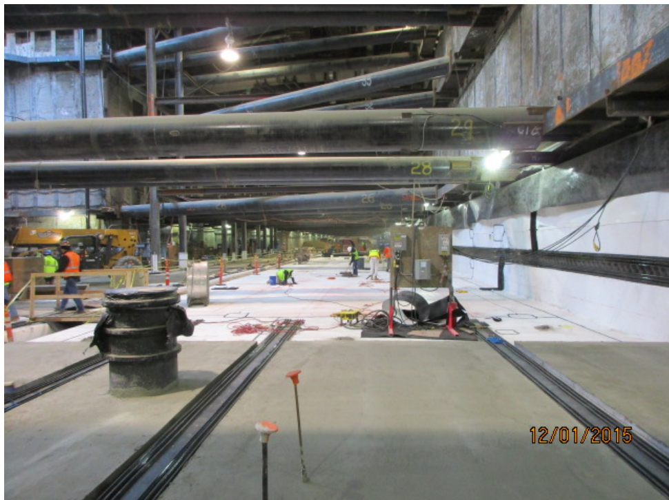
EXPO/CRENSHAW STATION – Welding waterbar to previously installed HCR membrane.
