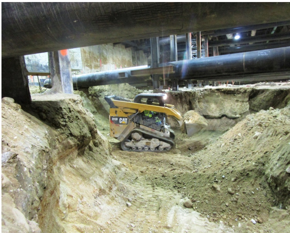
MARTIN LUTHER KING JR. STATION – Excavation operation toward Tier 3.
