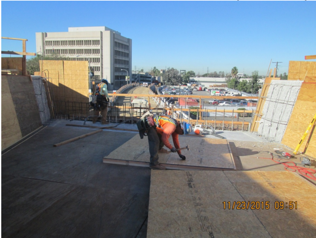
LA BREA BRIDGE - Back wall formwork.
