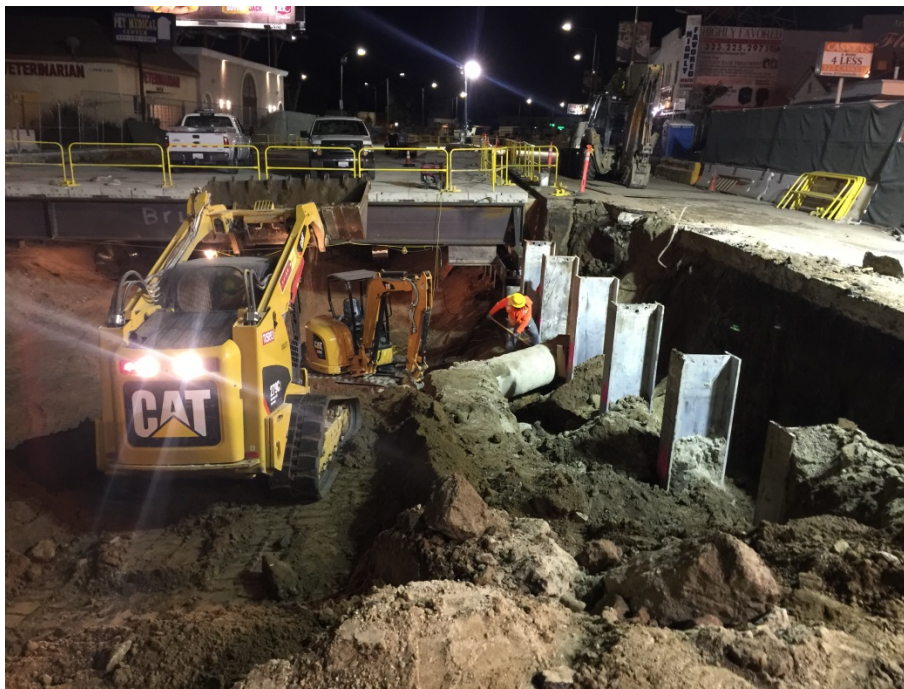
UG4 – Excavation operation around utilities.
