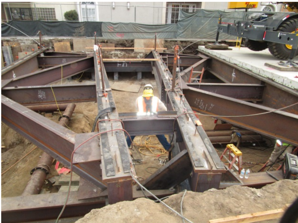
UG4 – Welding cross braces for the deck beams looking east.
