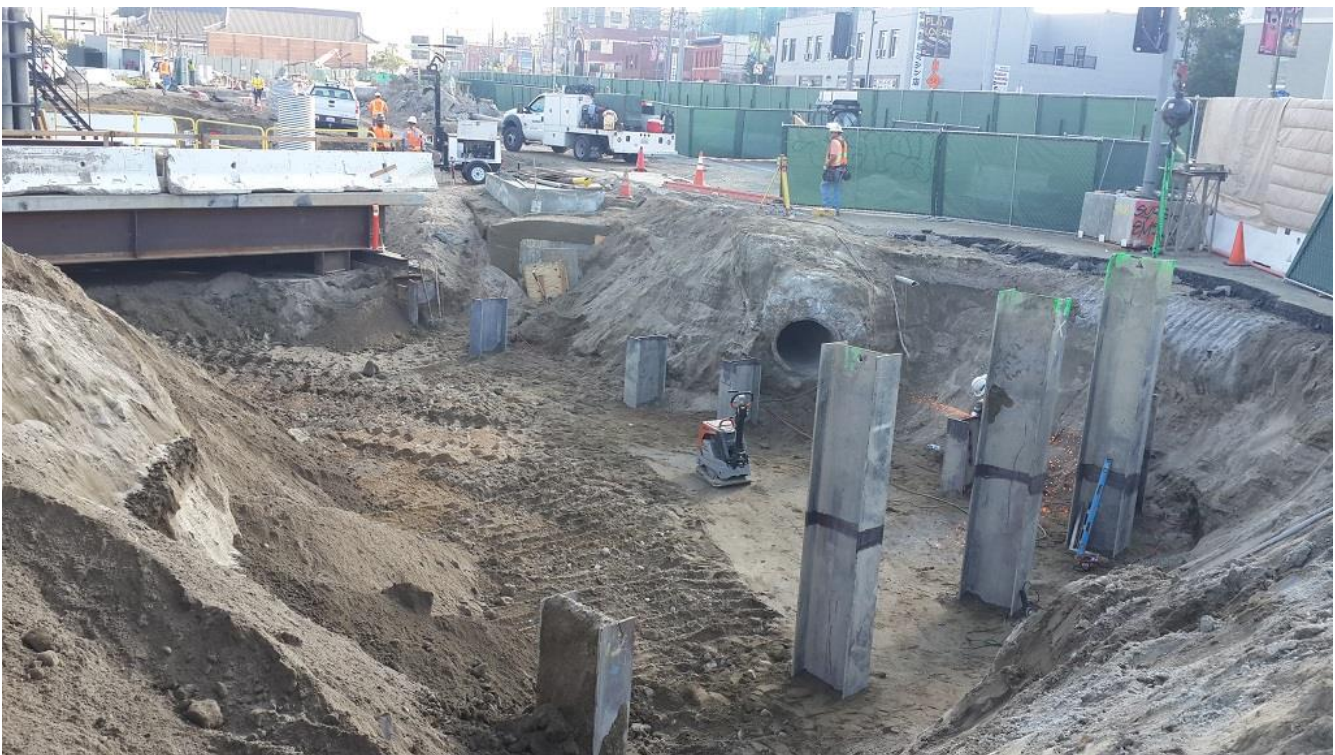
Excavation and pile installation at Mangrove Yard
