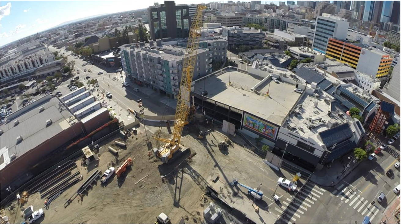
1 st /Central Construction Activities
