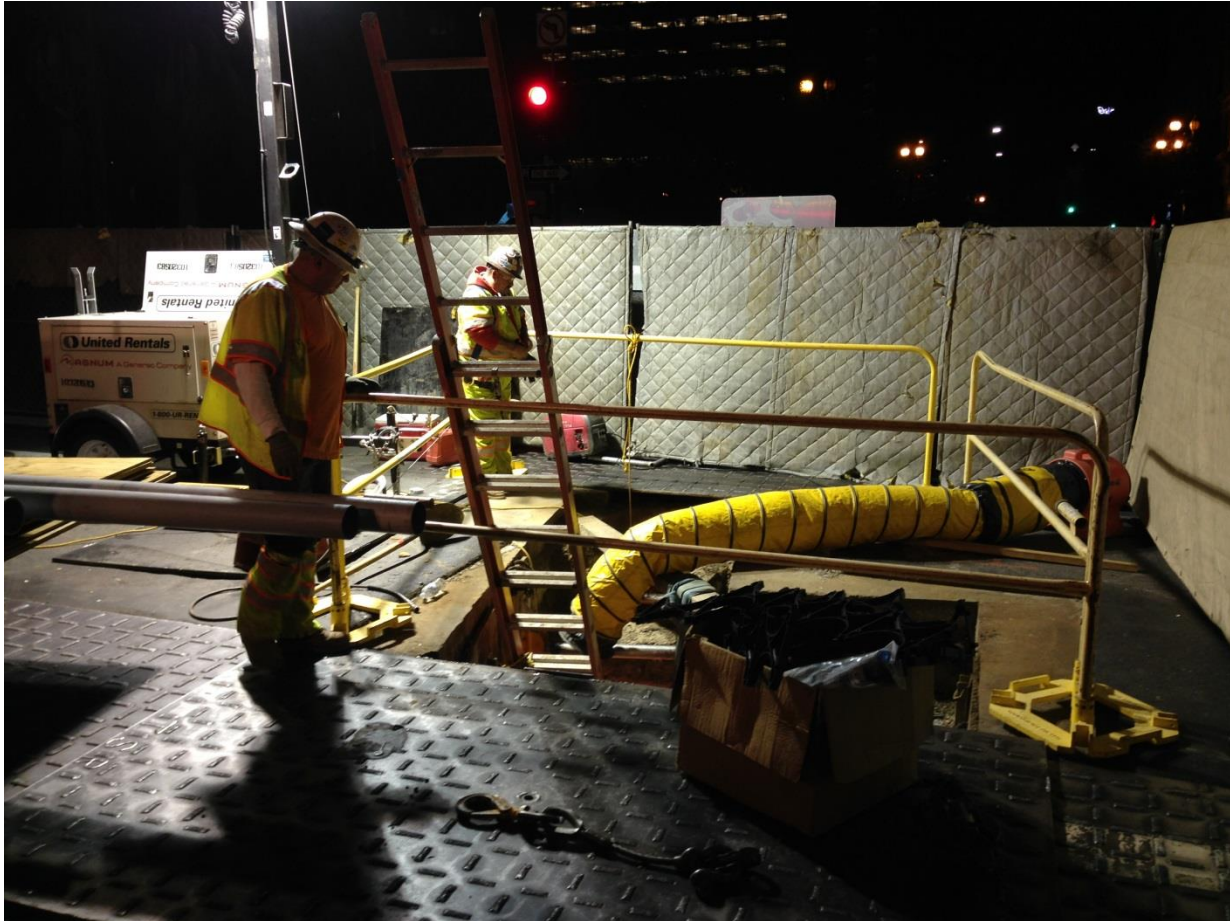
Nighttime electrical work at 2 nd /Spring
