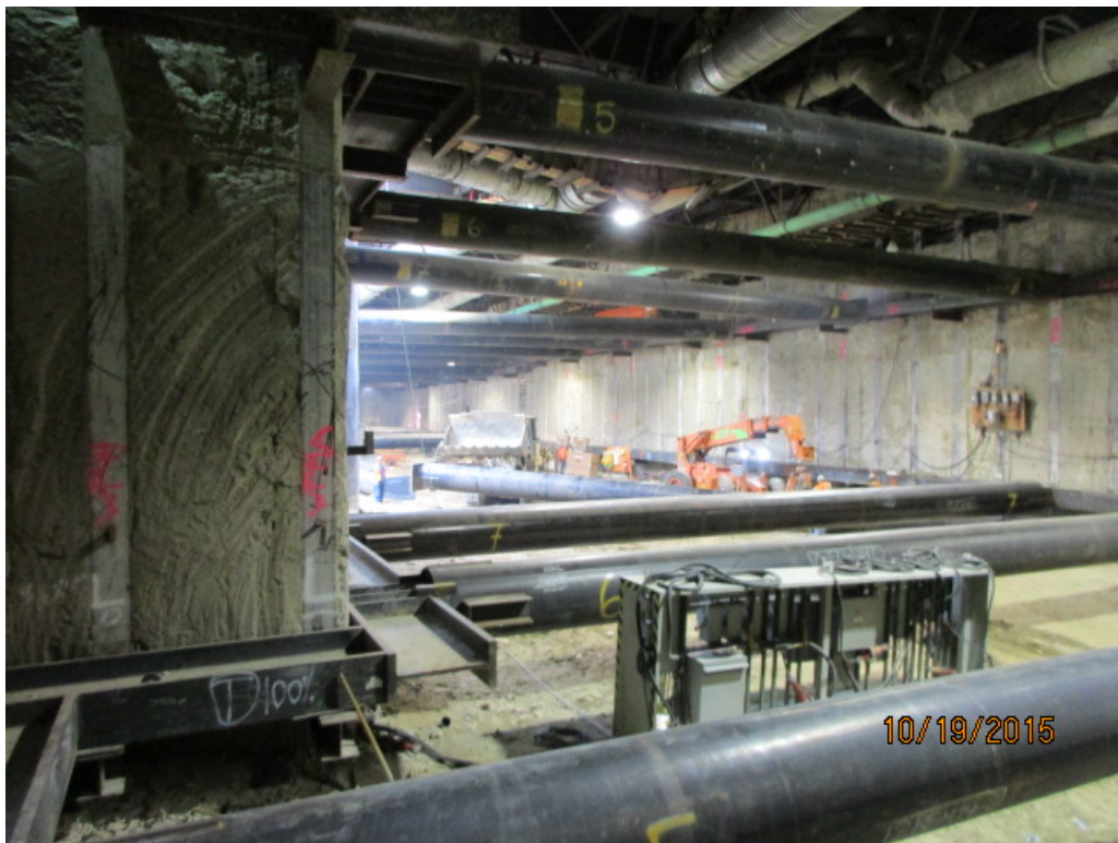
MARTIN LUTHER KING JR. STATION – Tier 2 SOE strut installation
