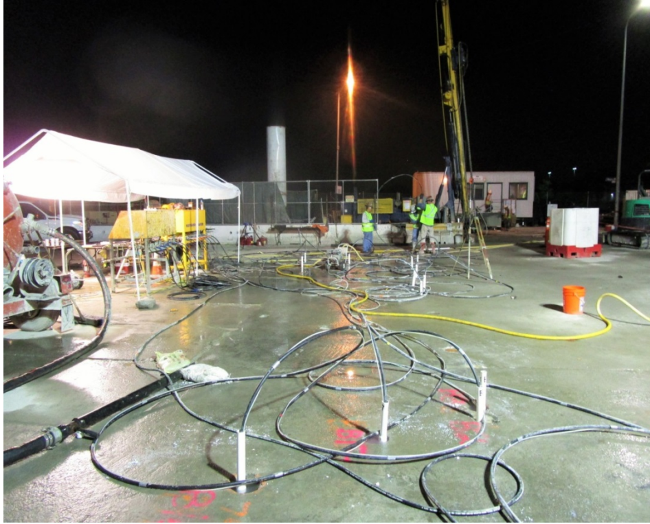
CRENSHAW/EXPOSITION STATION – TBM Break-out Chemical grouting operation
