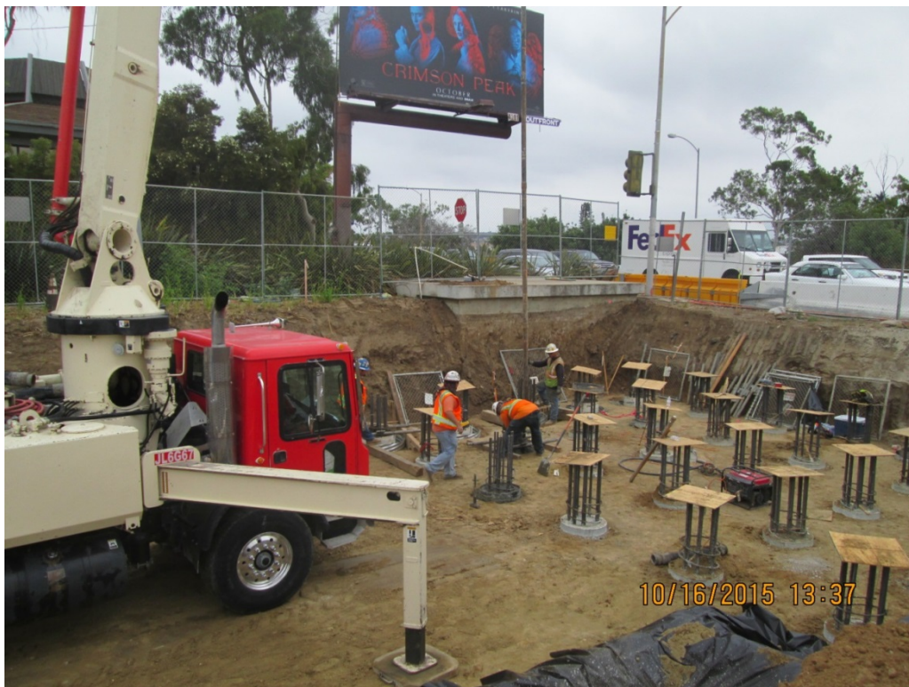
I-405 - Abutment 1 CIDH placement
