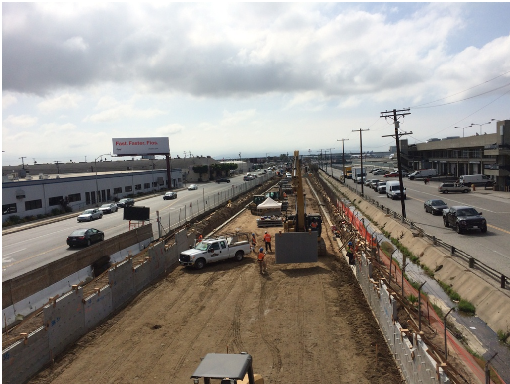
AVIATION/CENTURY - MSE (Wall 3 60L&R): Precast Panel erection
