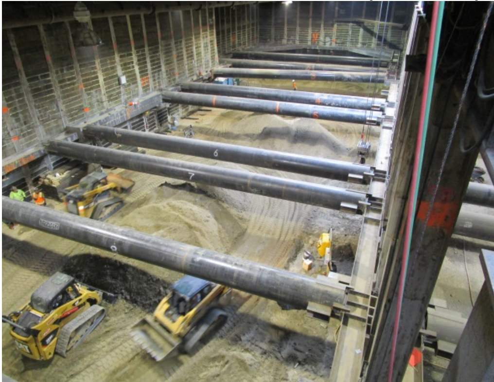
LEIMERT PARK STATION – Excavation operation looking north
