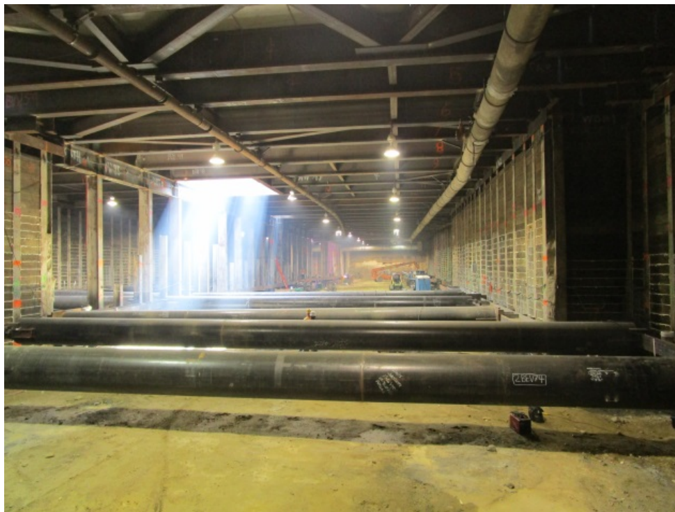
LEIMERT PARK STATION – Overall view looking south from north head wall
