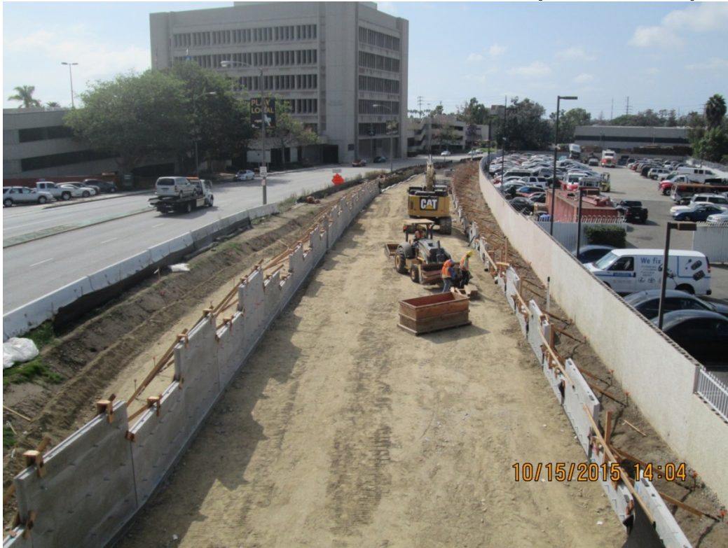
LA BREA BRIDGE - MSE panel erection
