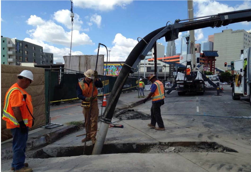
1 st /Alameda potholing for Deck Beams
