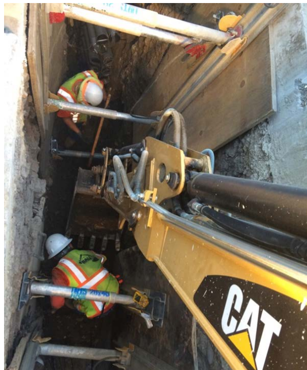
Trench Excavation at Broadway St.
