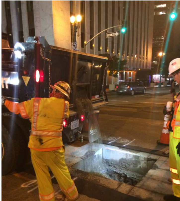
Backfilling pothole trench with pea gravel at Flower St.
