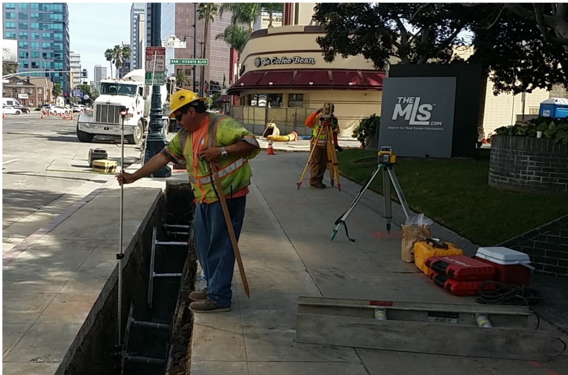
Surveyors Providing As-Built Data for SCE Ductbank Relocation
