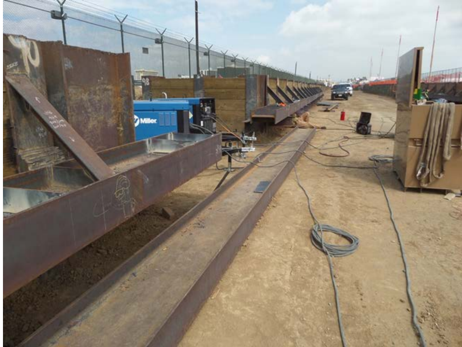
UG1: Welding walers along West pile line.
