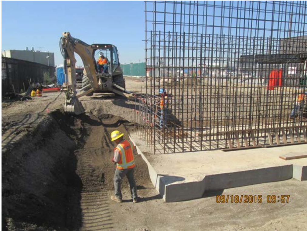
MANCHESTER – Abutment 1, structural backfill.
