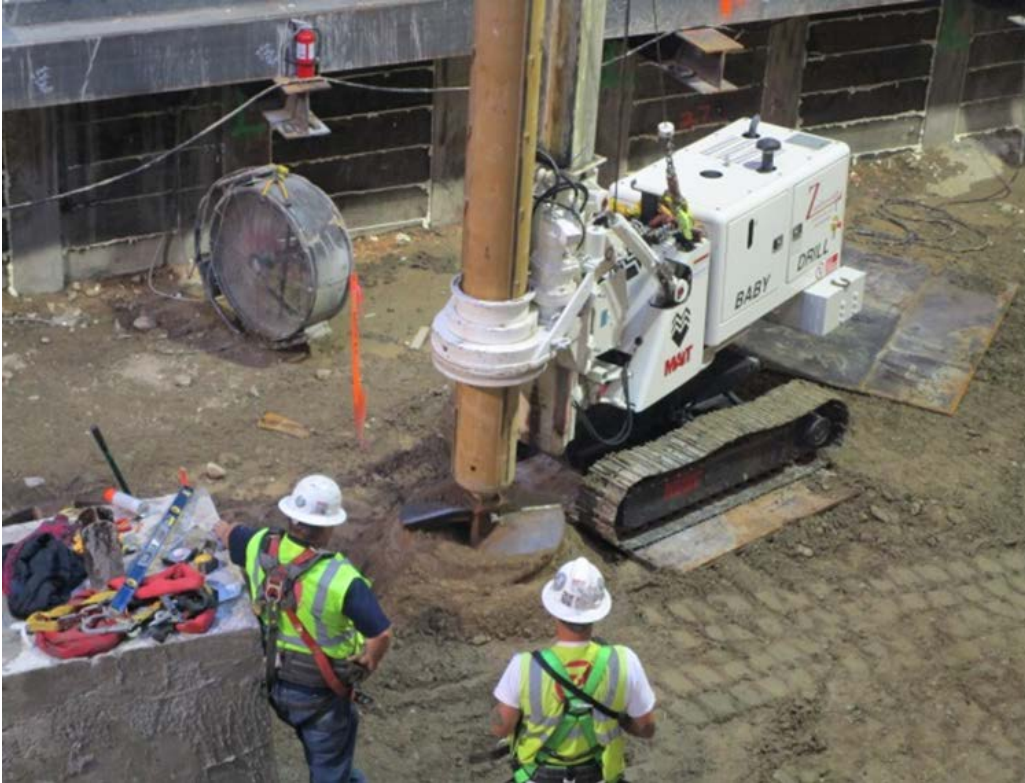
LEIMERT PARK Drilling for elevator Shaft #2.
