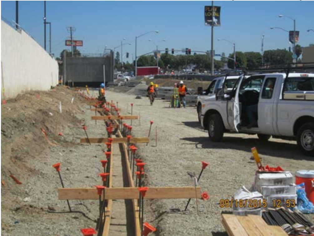
B1 GUIDEWAY - Cutting grade and leveling pad.
