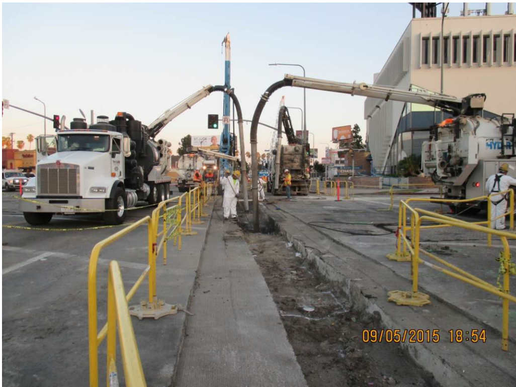
UG4 – Pot holing utility locations for pile layout.
