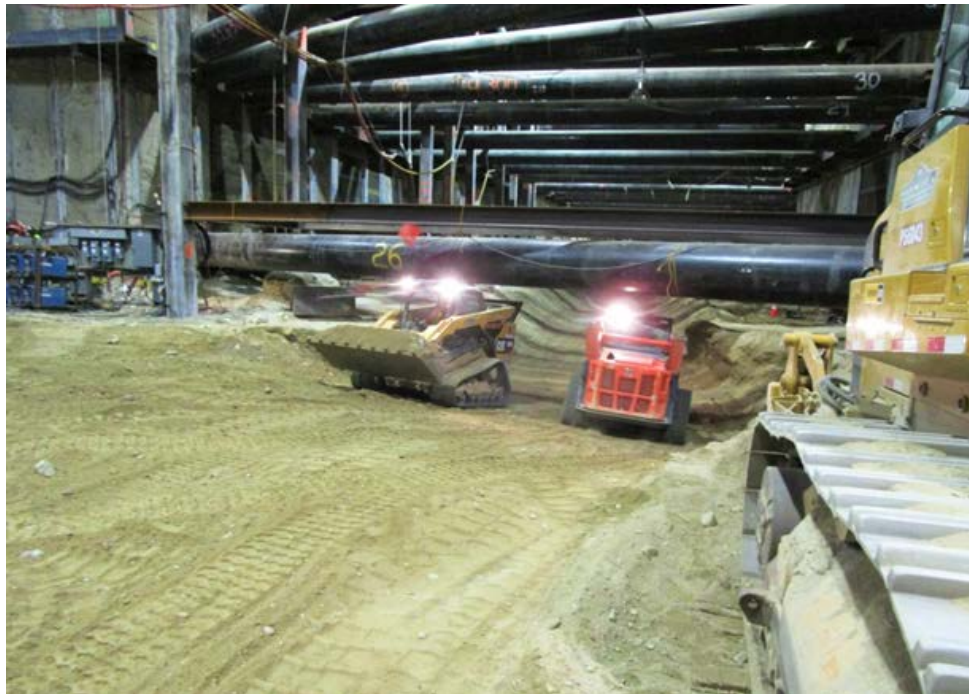
EXPOSITION/CRENSHAW – Excavating trough beneath Tier 3 pipe struts.
