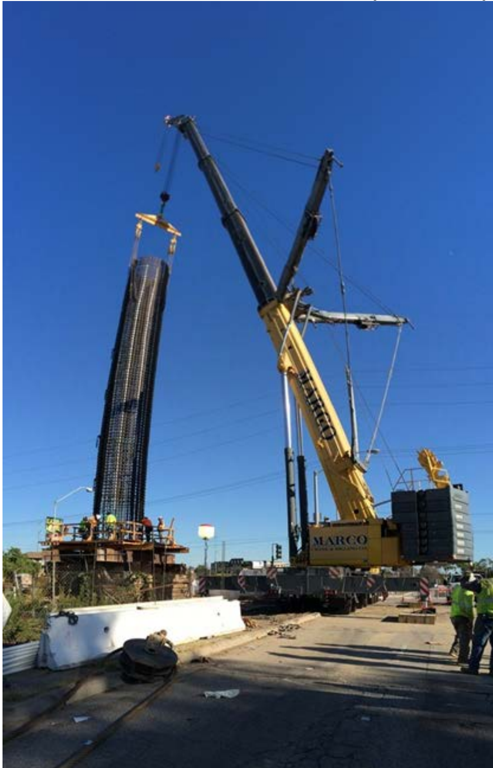
I-405 Bent 2 CIDH cage was set. Column cage being installed 09/24/15, followed by the concrete pour on 09/26/15.
