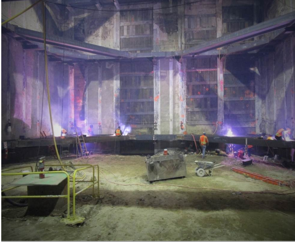
EXPOSITION/CRENSHAW – Tier-3 welding operation on south headwall.
