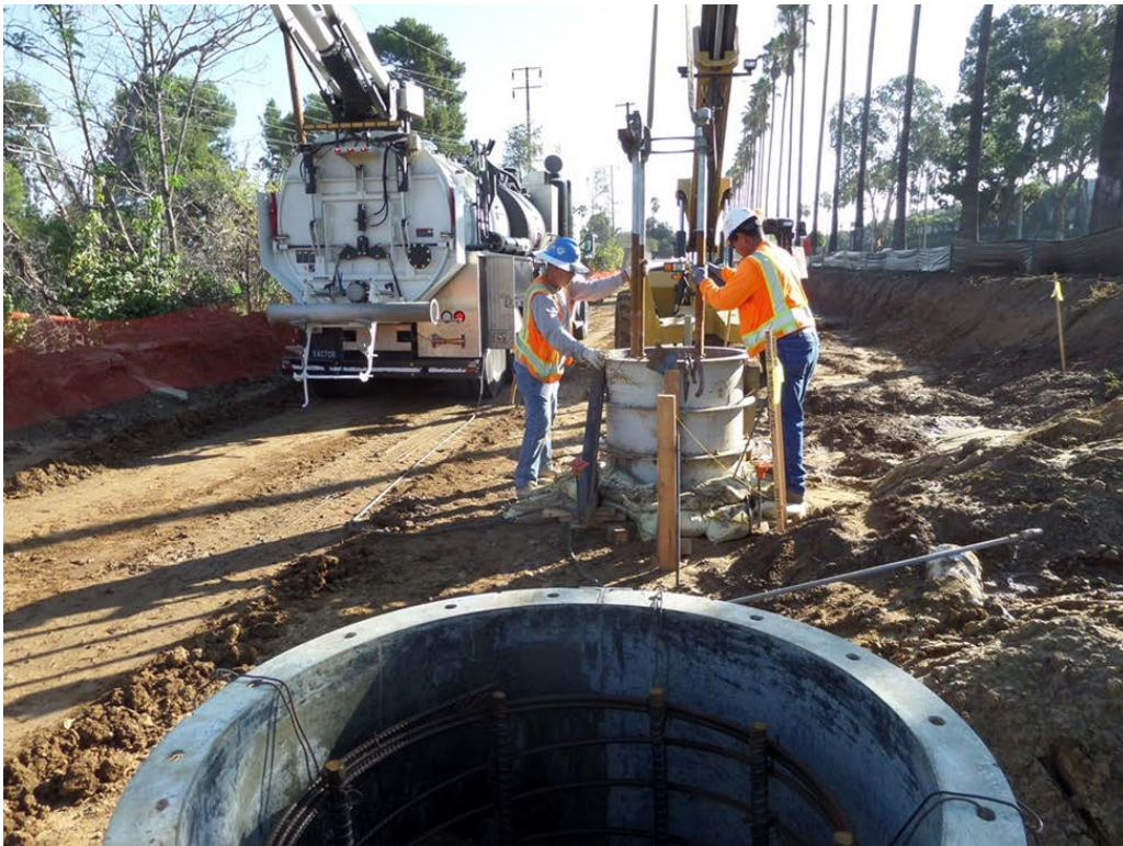
B1 GUIDEWAY – Continued OCS foundation work.
