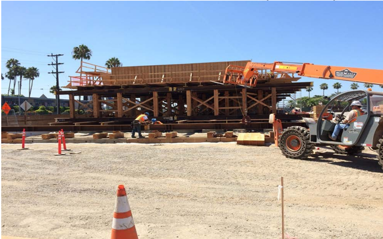
AVIATION/CENTURY : Bent 6 & 7; bent cap formwork construction. Abutment 1 footing; debris on subgrade, formwork and lagging removed.
