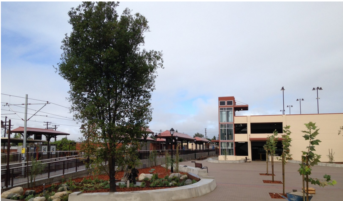
Monrovia Parking Structure Site Overview
