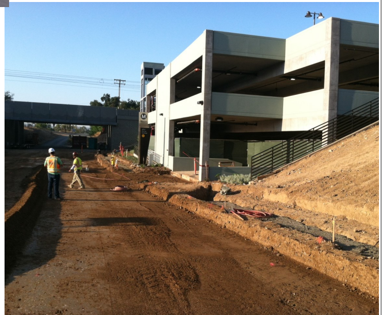
Azusa-Citrus Parking Structure Site Overview
