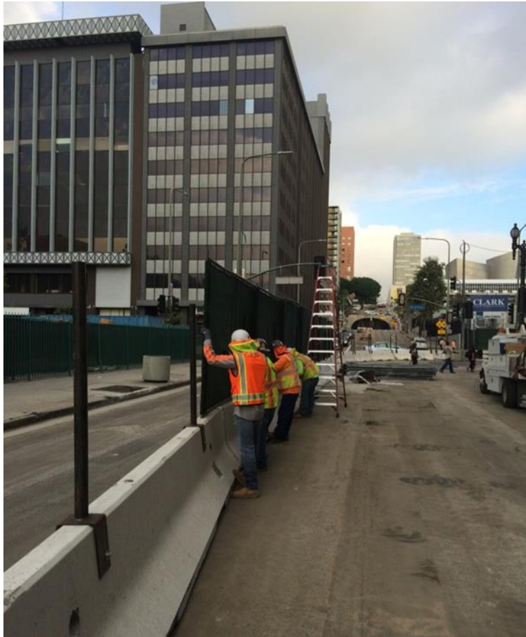
2 nd St. closure – Installing fence panels
