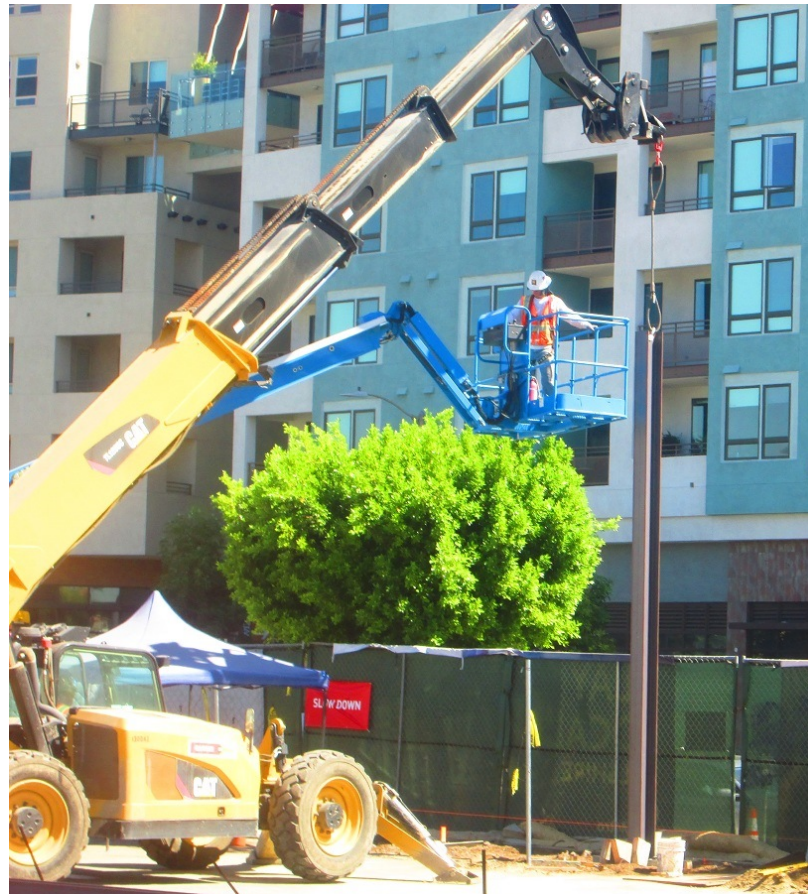
C1045 Contractor Installing Columns for the Soundwall at the South Wilshire/La Brea Construction Staging Site
