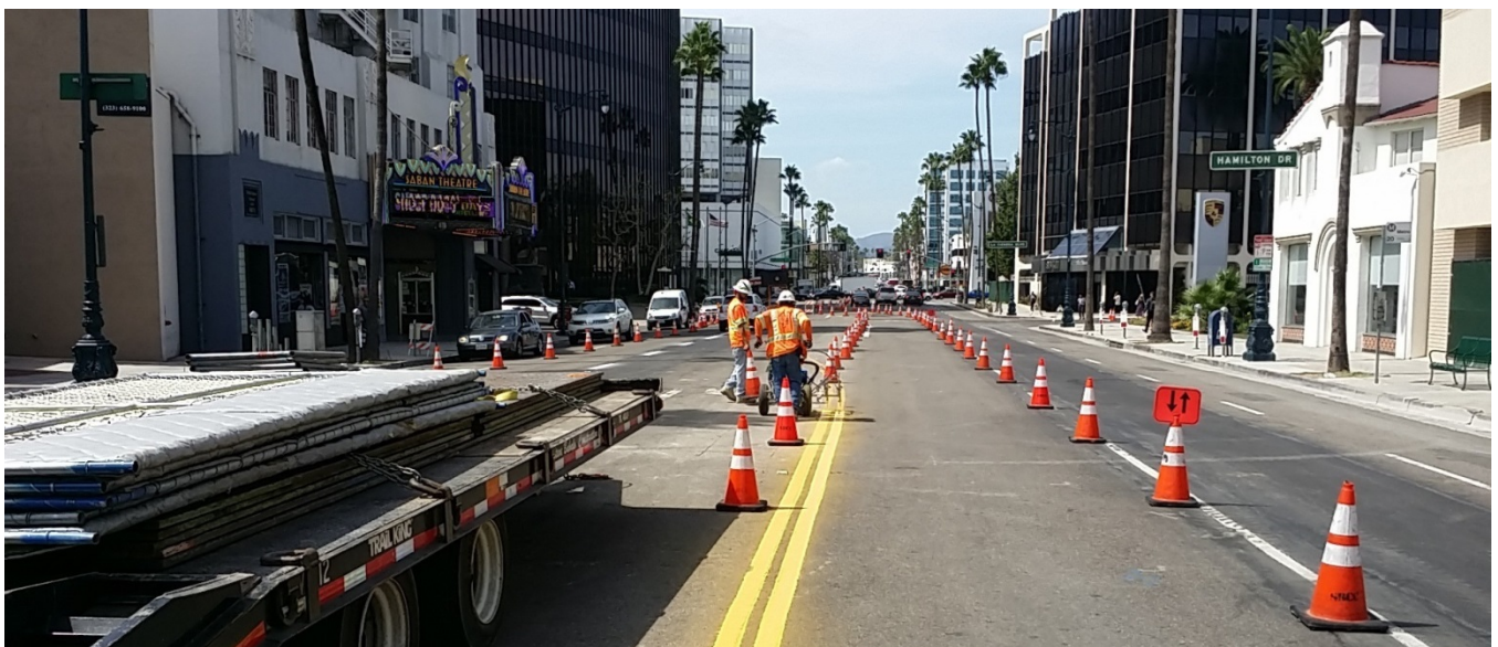
C1056 AUR Contractor Traffic Lane Striping on Wilshire Boulevard
