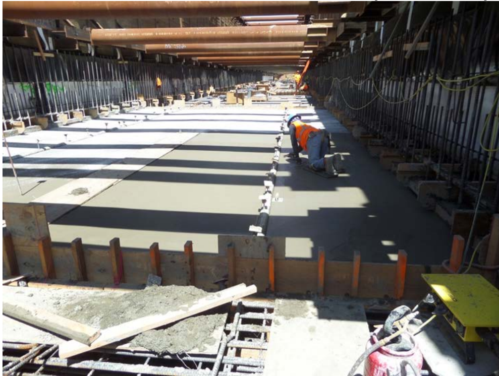
UNDERGROUND #1 – Invert concrete placement ongoing at south end.
