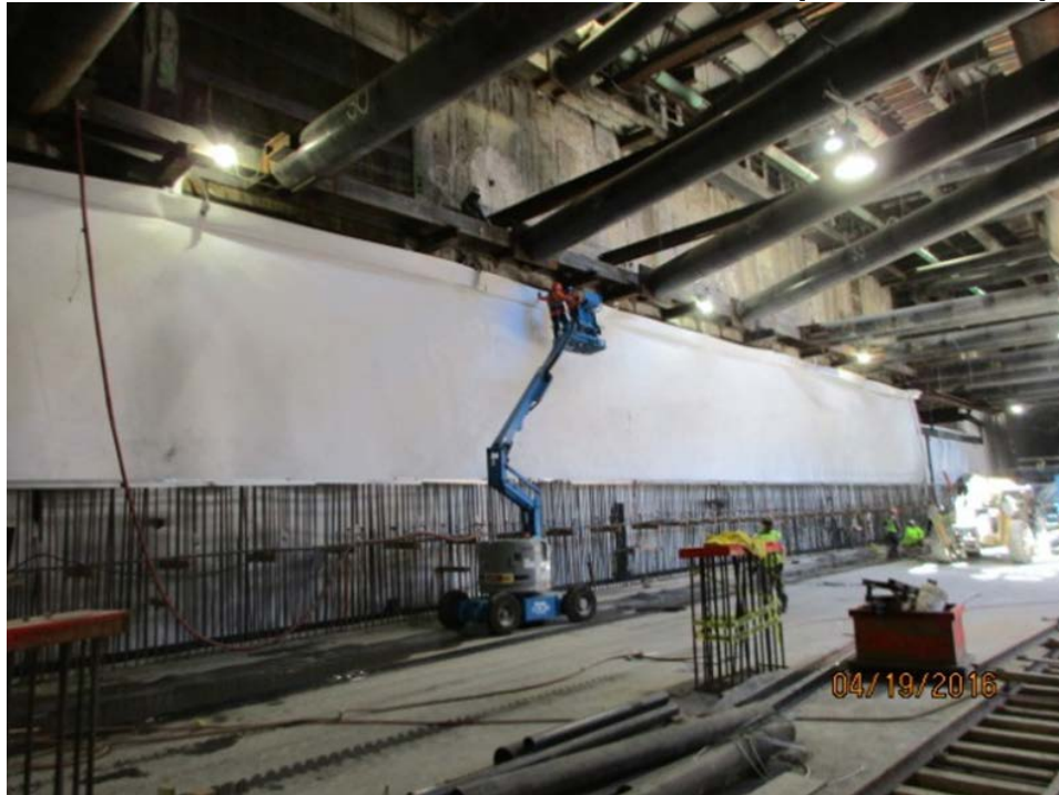
EXPOSITION/CRENSHAW STATION – Installation of waterproofing at west wall of station box.
