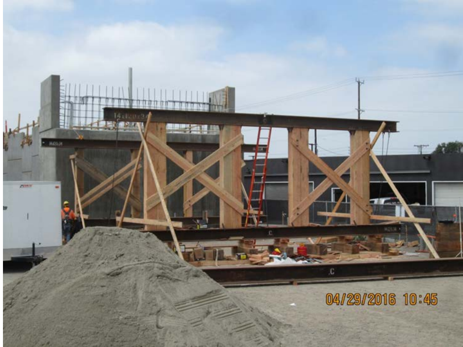
MANCHESTER BRIDGE – Falsework fabrication and erection begins.
