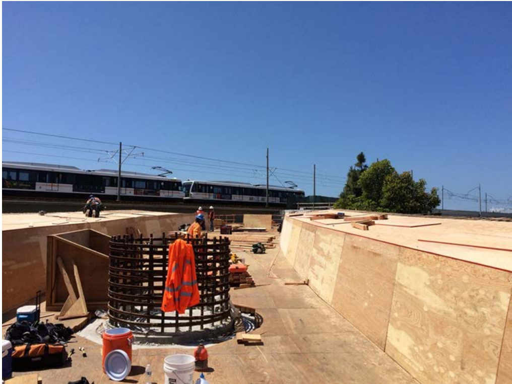
GREENLINE UNDERPASS – Exterior girder, overhang and soffit formwork placement ongoing.
