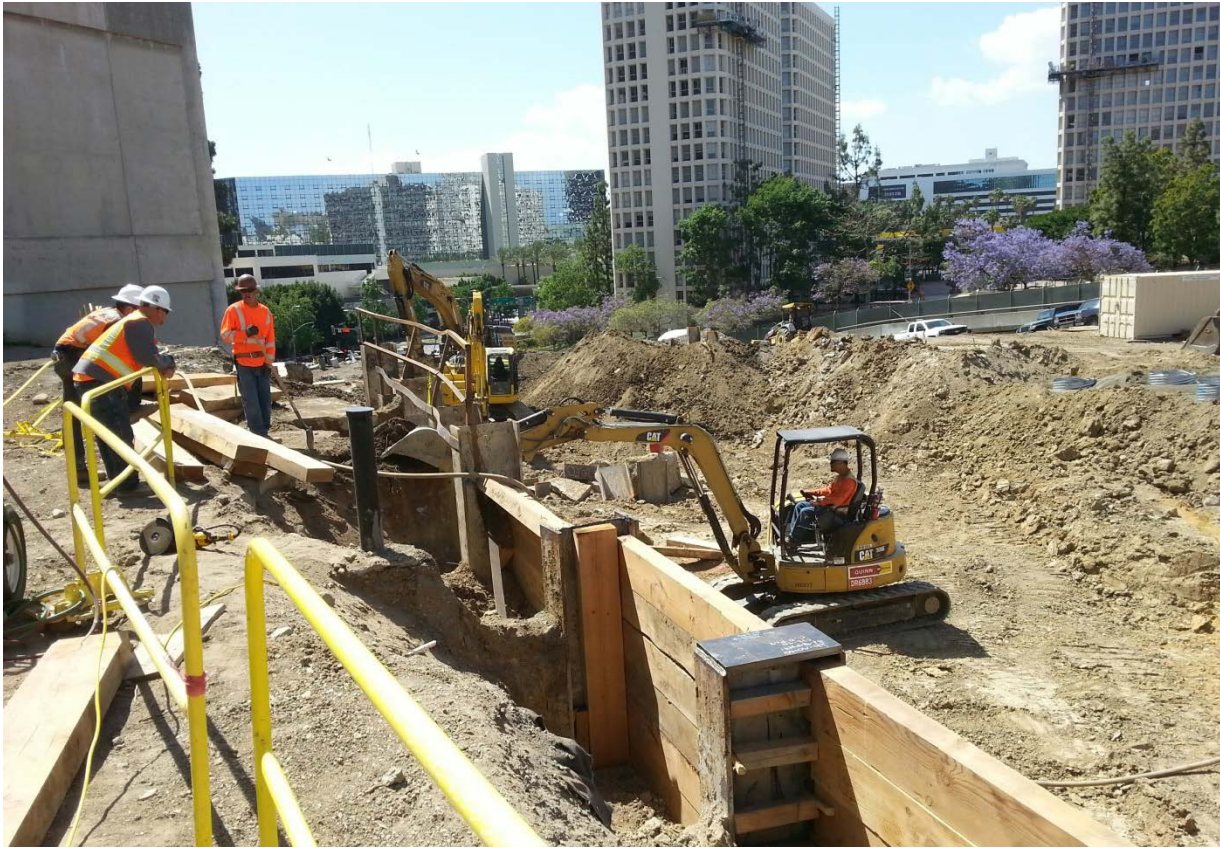
2 nd /Hope construction activities
