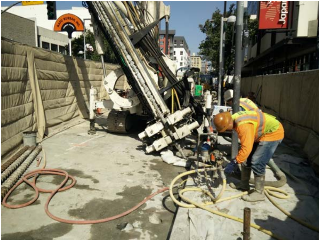
Permeation Grouting at 2 nd Street
