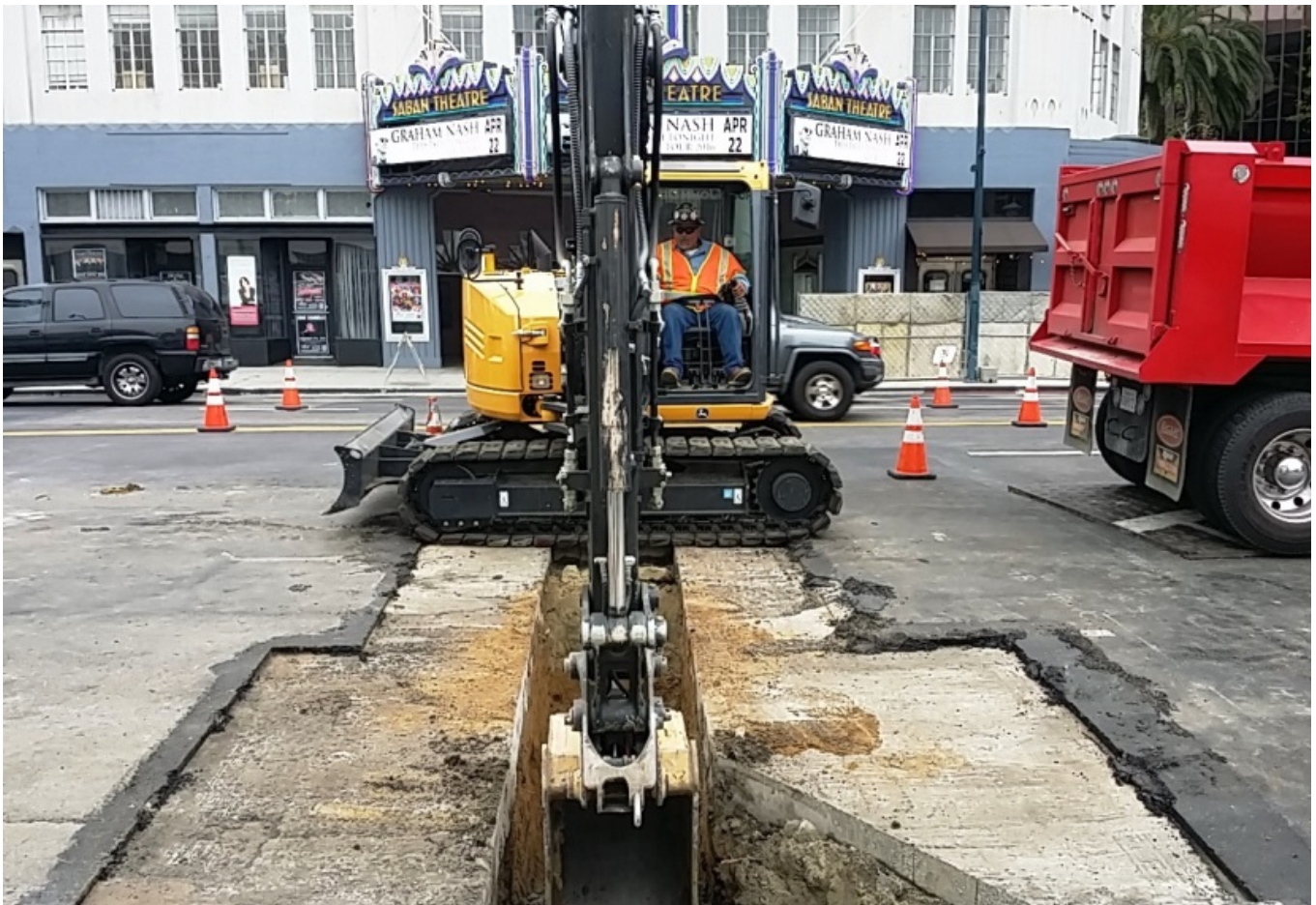
C1056 Contractor Excavating Sewer Lateral on Wilshire Boulevard
