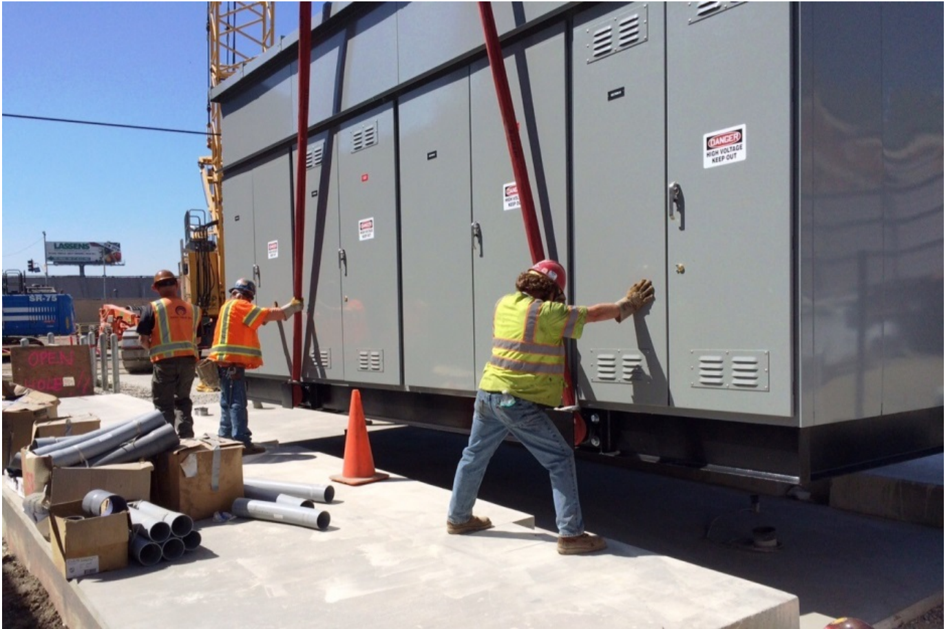
C1045 Contractor Installing Electrical Metering Switchgear for Tunnel Operations
