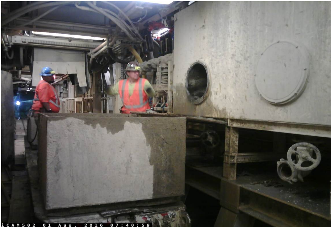
TUNNELING – Mucking out discharge tank.
