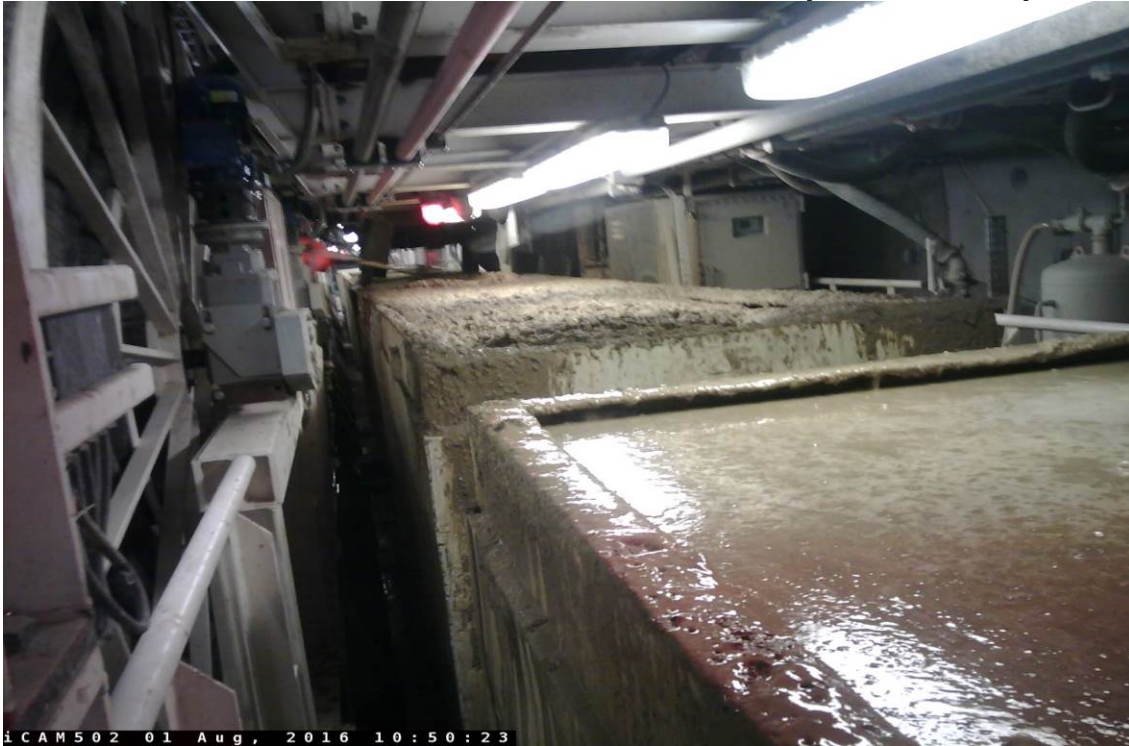
TUNNELING – Advancing TBM and hauling out muck cars.
