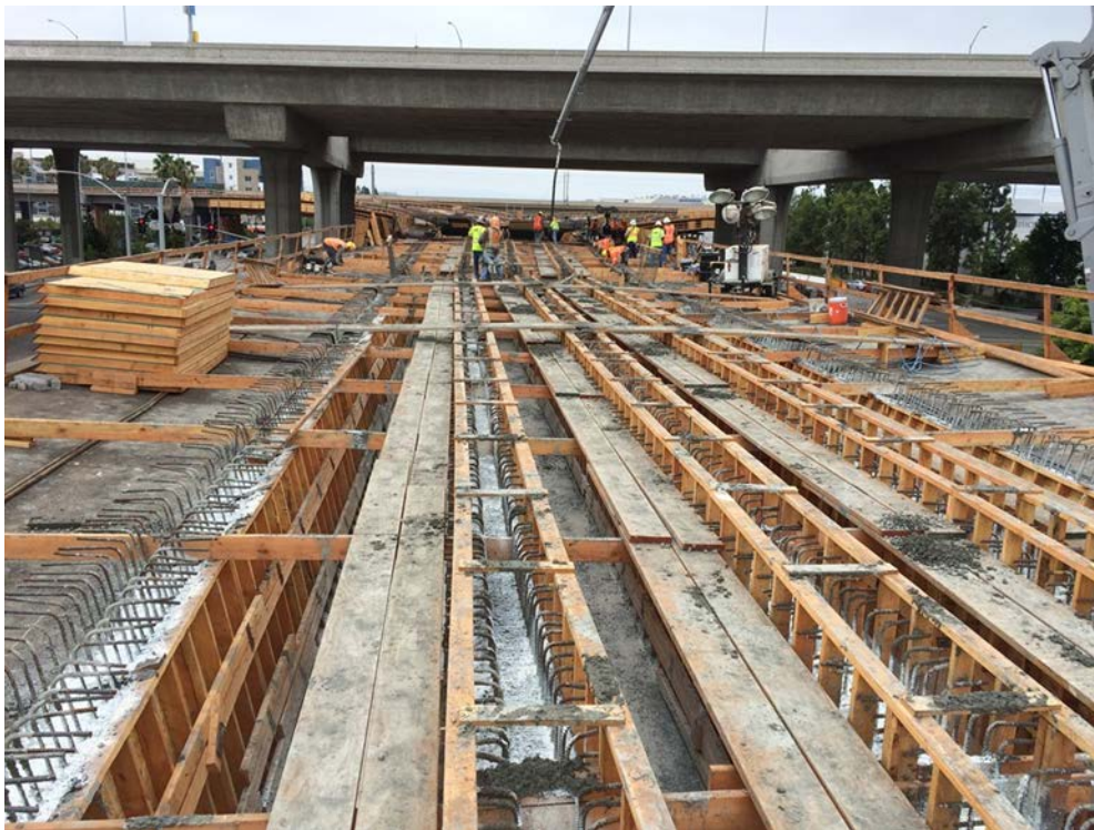
GREENLINE UNDERPASS – Frame 2 pour looking down at station.
