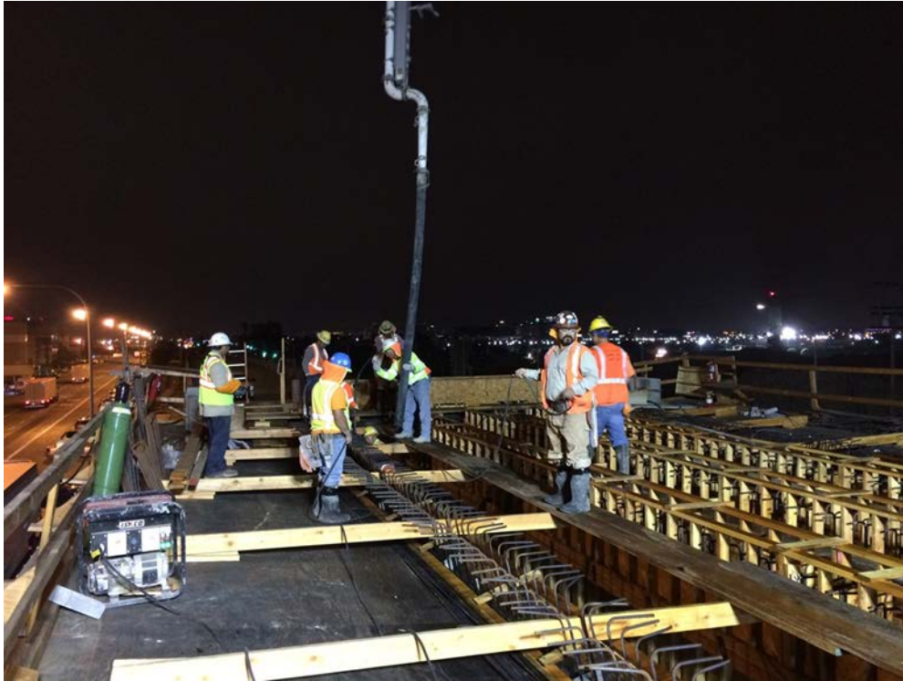
GREENLINE UNDERPASS - Frame 2 first pour of soffit and stems.
