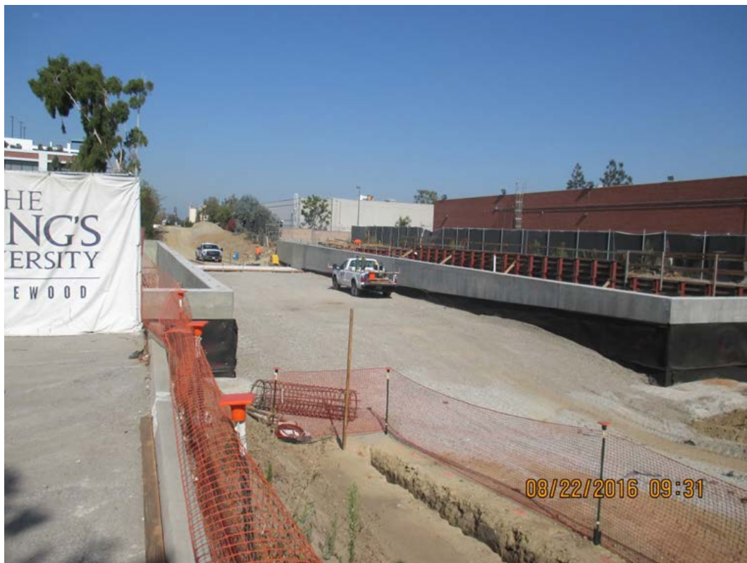
FAITHFUL CENTRAL BIBLE CHURCH PEDESTRIAN UNDERPASS – Backfilling and compaction testing between exterior ramps.
