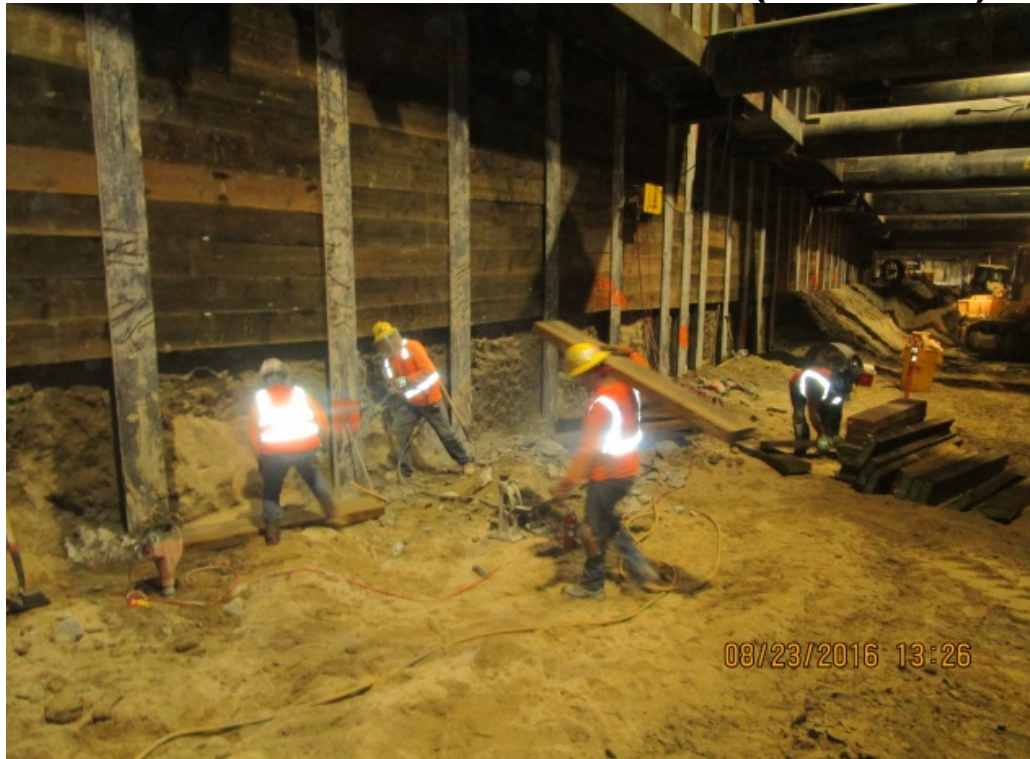
UG#4 – Excavation and lagging along west wall.
