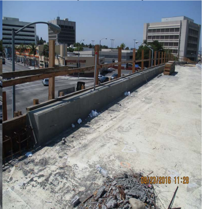
LA BREA BRIDGE – Worked on forming and concrete placement for the bridge deck parapet walls.
