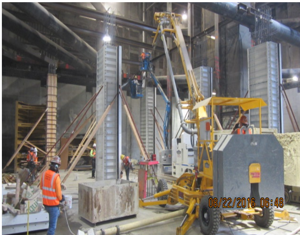
EXPOSITION/CRENSHAW STATION – Placement of lower invert columns at the north end of station box.
