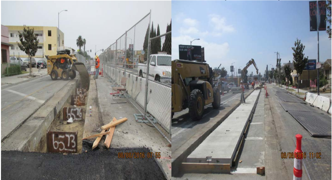
UG#3 – Backfilling and setting deck panels along the west pile line.
