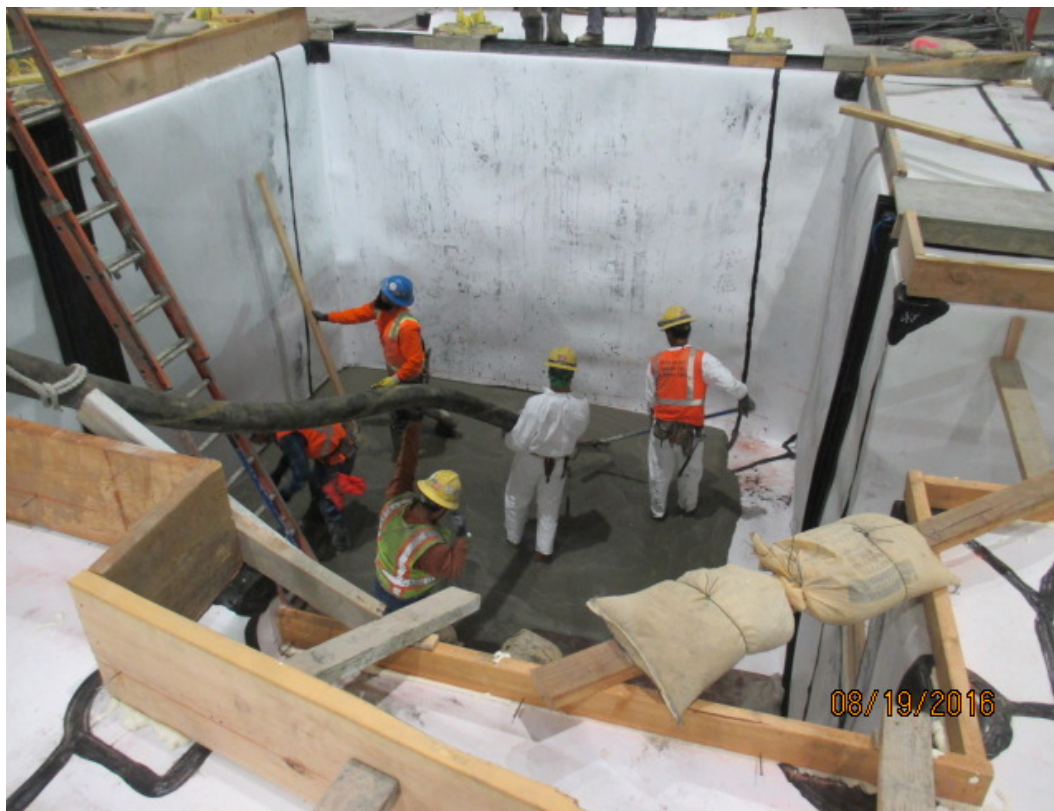
LEIMERT PARK STATION – Placement of protection slab at sump pit.
