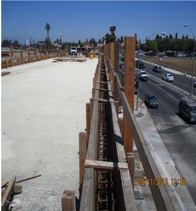
LA BREA BRIDGE – Worked on forming and concrete placement for the bridge deck parapet walls.
