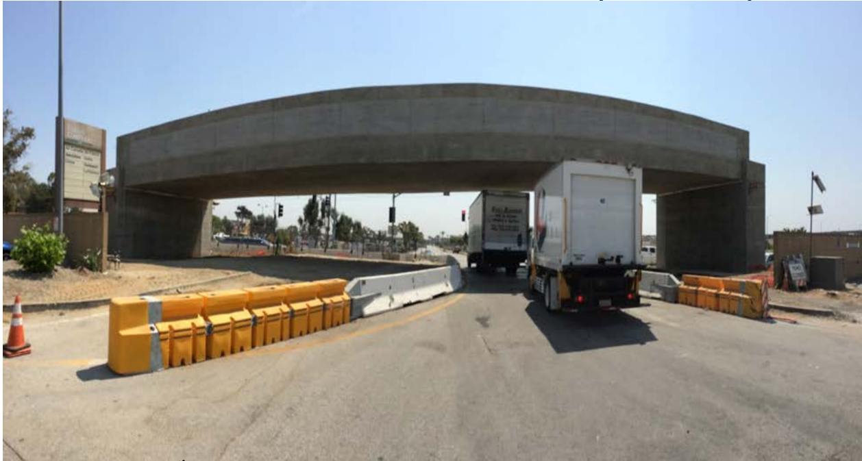
111 th STREET UNDERPASS - Panoramic view looking east.
