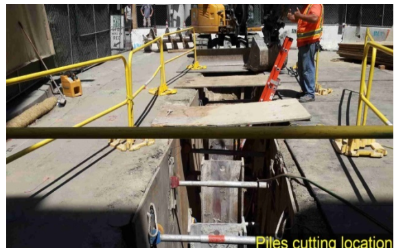
Pile related work on Flower Street
