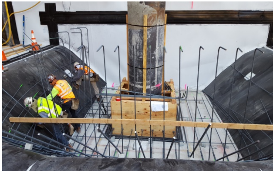
Installation of rebar for elevator shaft at 1 st /Central Station
