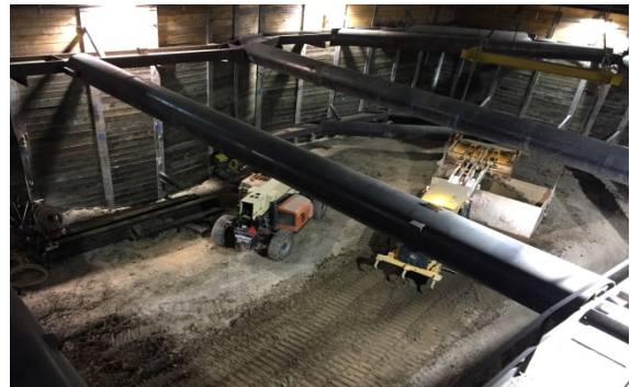
Excavation at 2 nd /Hope Station
