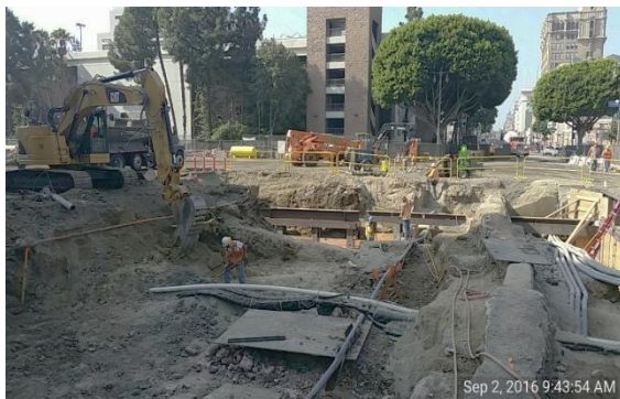
Deck beam installation at 2 nd /Broadway intersection
