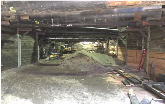
Excavation at Alameda Wye
