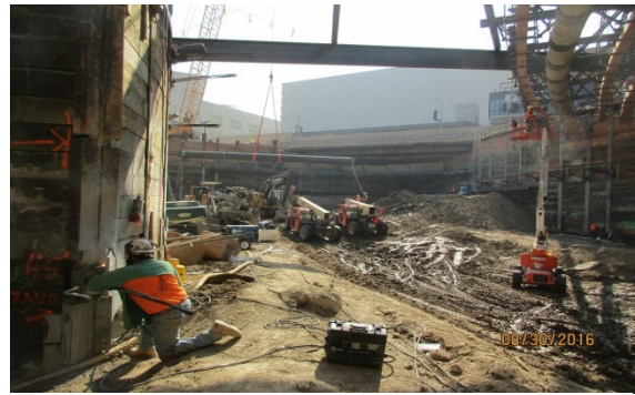
Tie-back related work at 2 nd /Hope Station
