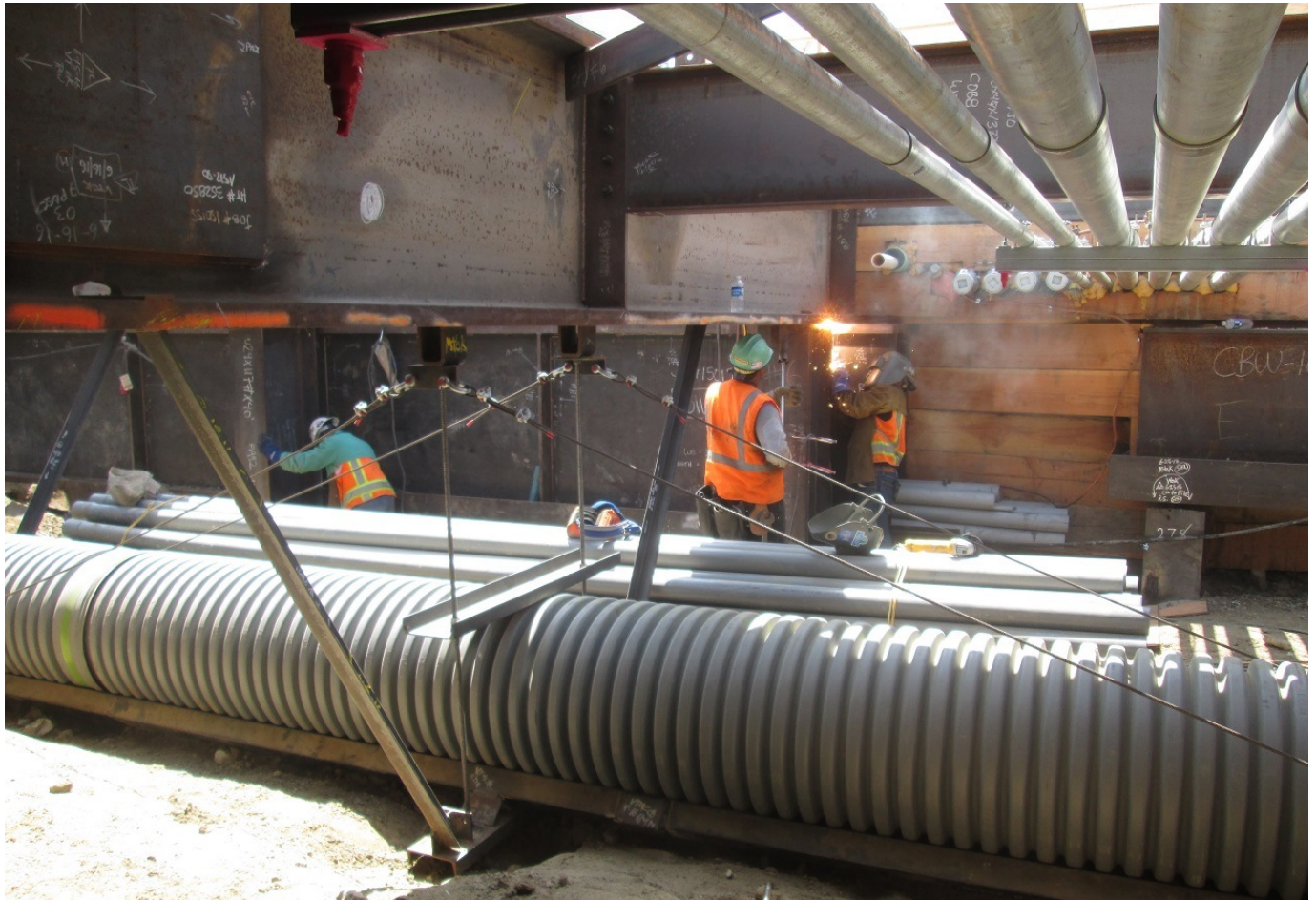
Utilities in Place under Wilshire/La Brea Station Decking
