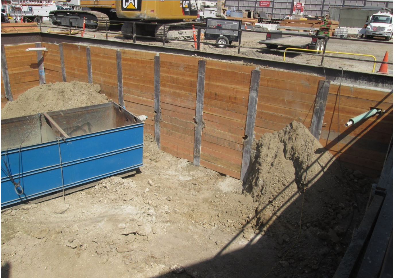
C1045 Contractor Excavation of North Muck Shaft at Wilshire/La Brea Station
