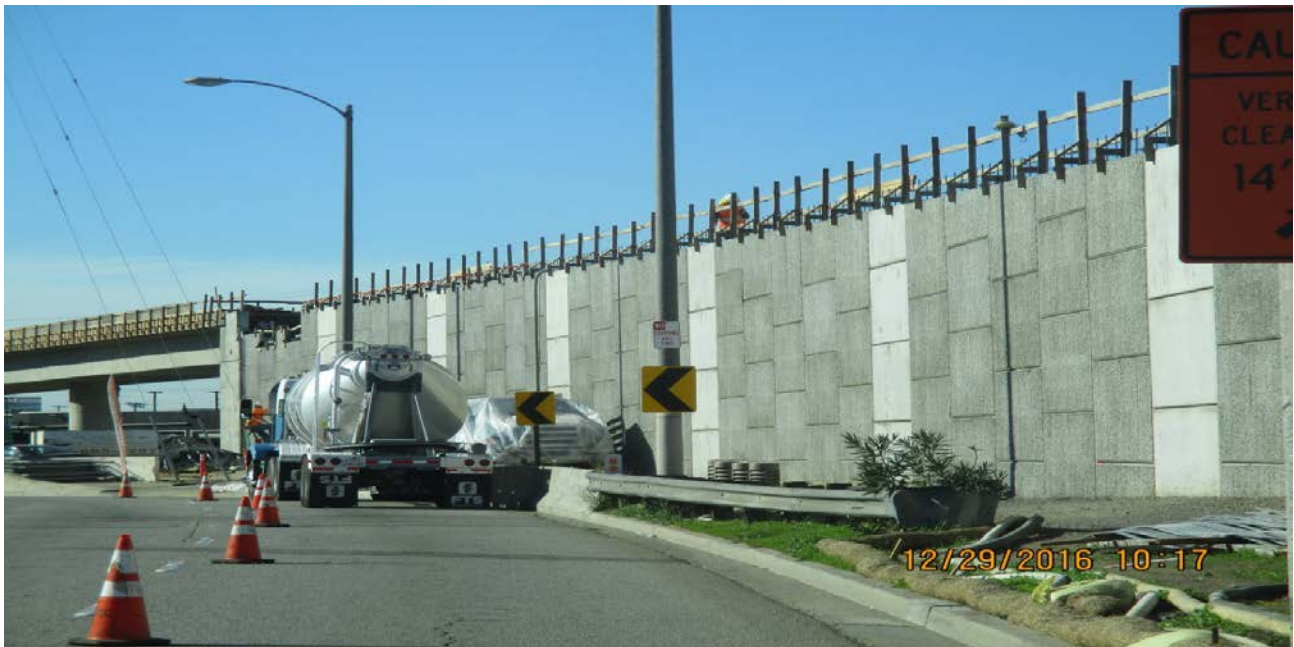
MSE 122 L & R (North of Manchester Blvd.) MSE 122 L&R facing down-station.
