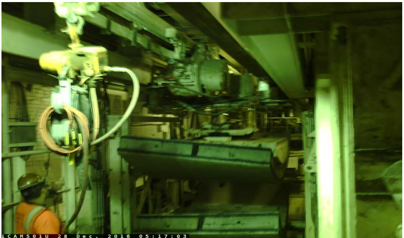
TUNNELING – Move tunnel segments to feeder for ring build.
