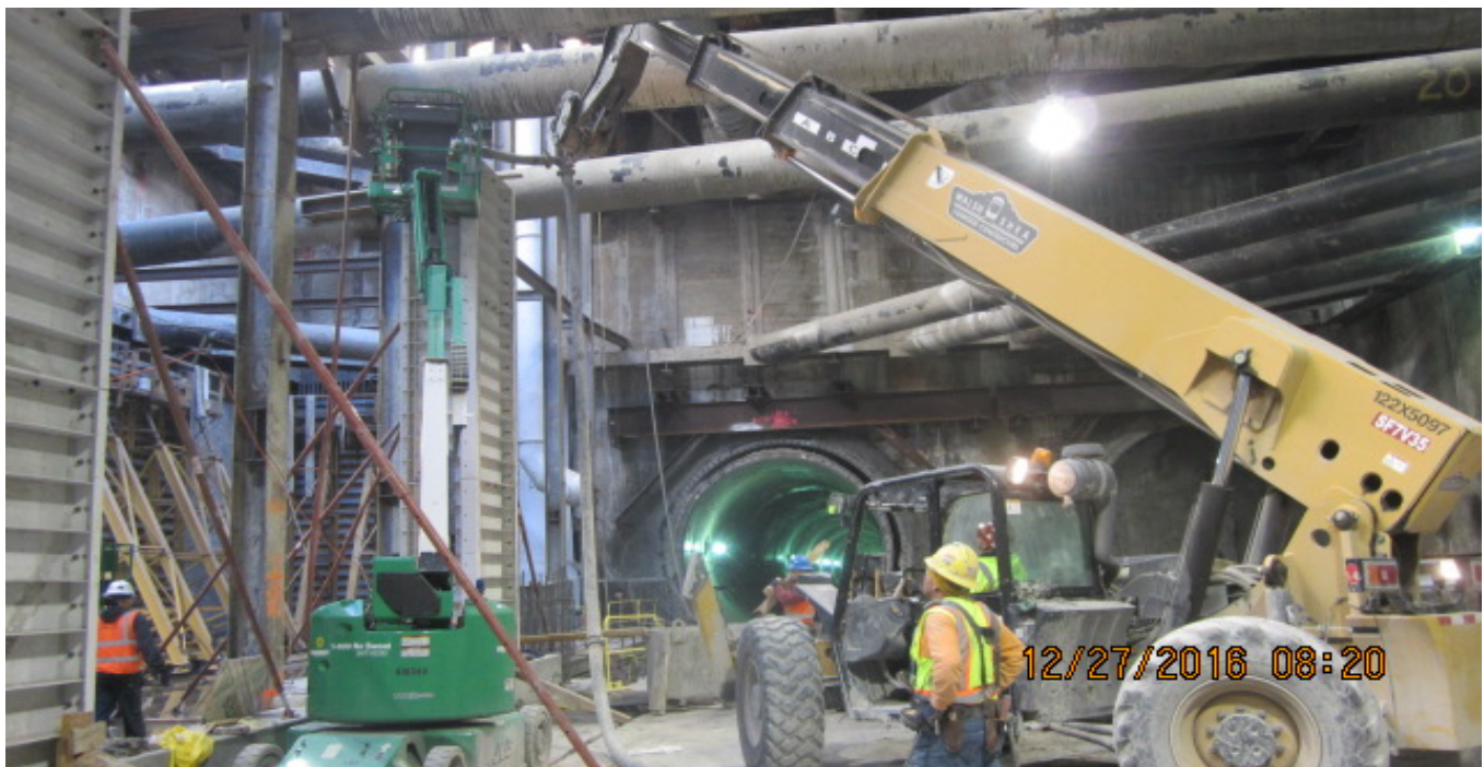
MARTIN LUTHER KING JR. STATION – Placement of invert columns.
