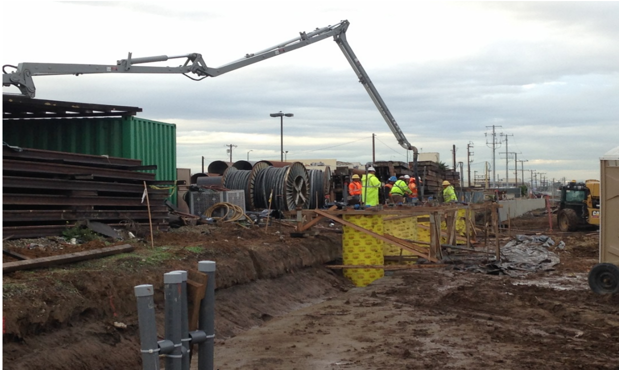
ACCOMODATIONS FOR 96 th STREET STATION – Ballast retainer wall construction ongoing.
