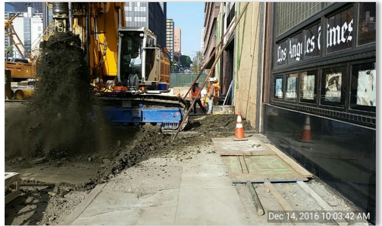
Piling on 2nd Street
