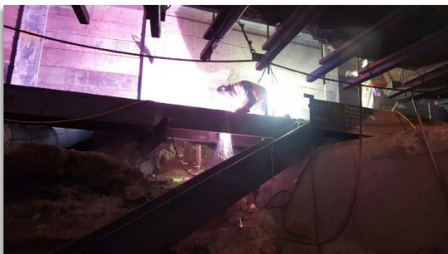
Welding of walers under Flower Street decking
