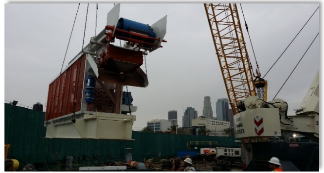
Muck conveyor system being lowered at 1st/Central Station
