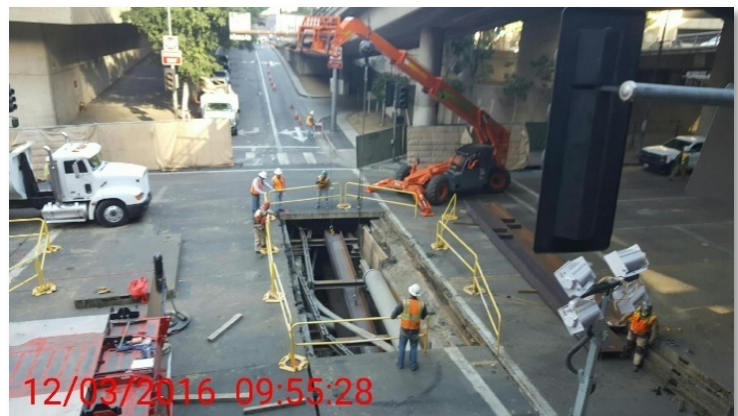
Lowering walers (support of excavation) at 4th/Flower
