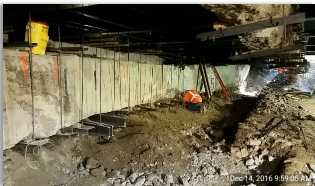
Utility hanging under 2nd Street decking
