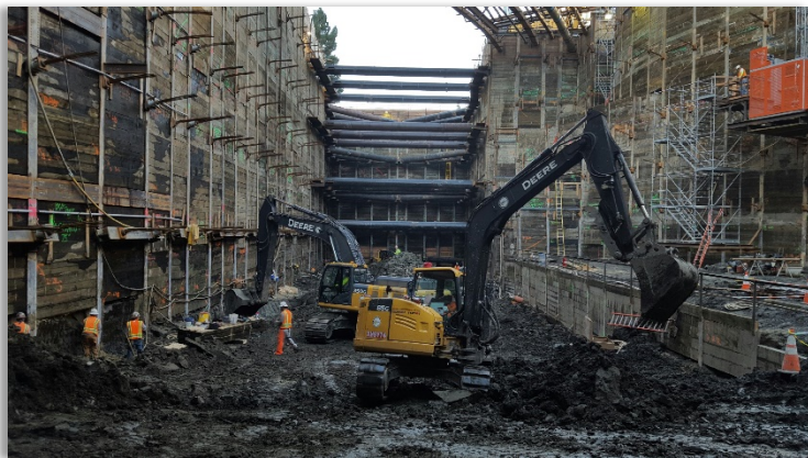
Excavation and lagging at the center of 2nd/Hope Station
