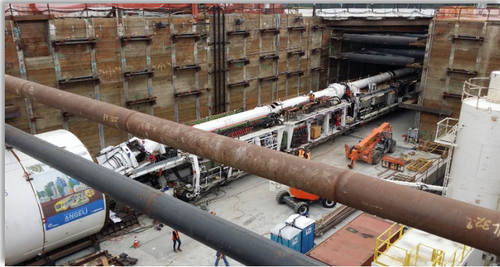
TBM assembly underway at 1st/Central Station
