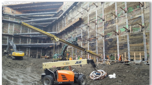
Drilling for tie-backs at 2nd/Hope Station
