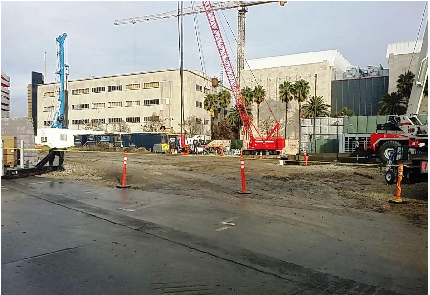
View of South Wilshire/Fairfax Construction Staging Yard
