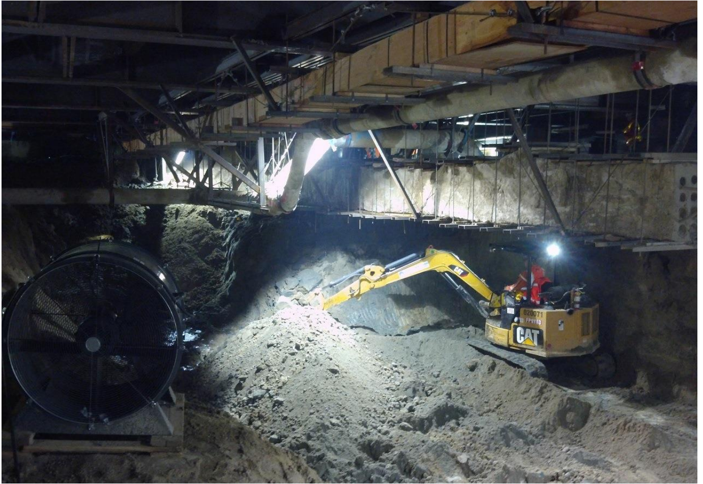
Wilshire/La Brea Station Excavation under Decking
