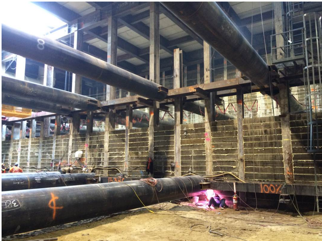
LEIMERT PARK STATION – Tier-2 strut installation looking east
