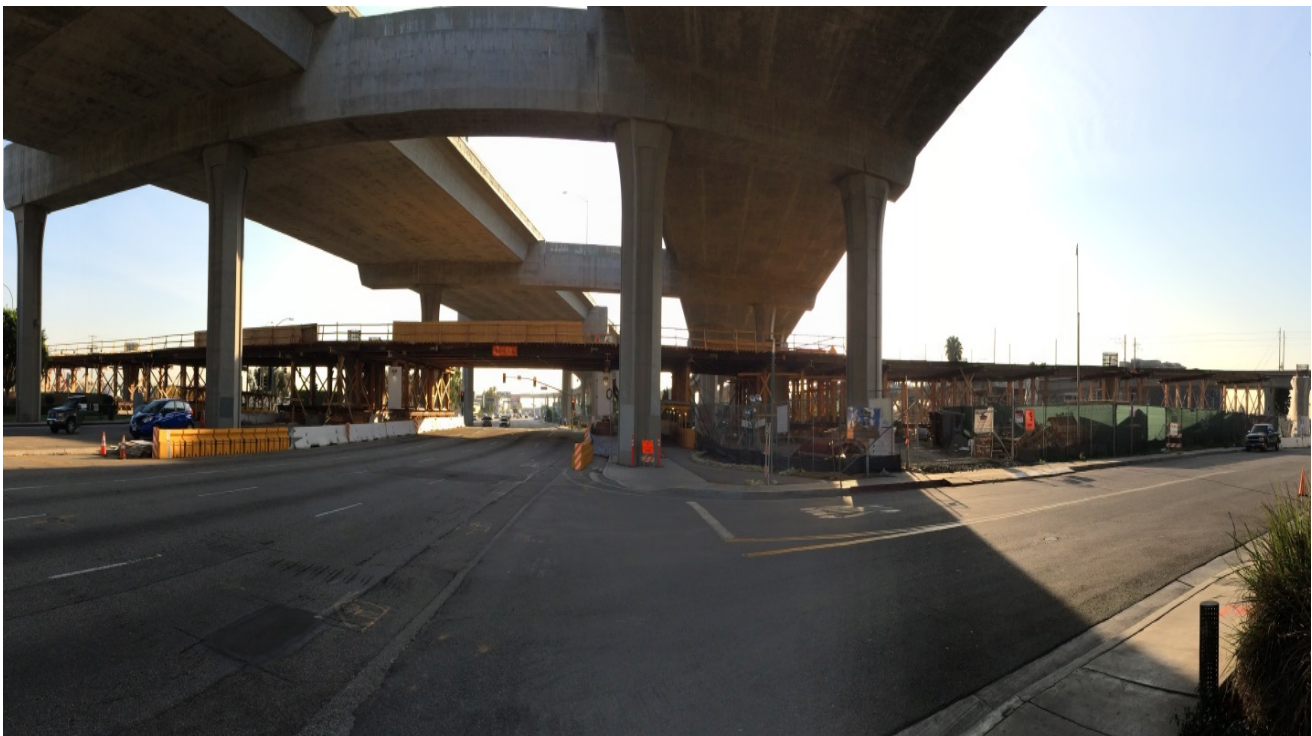
GREENLINE UNDERPASS – Falsework and rolling soffit continue
