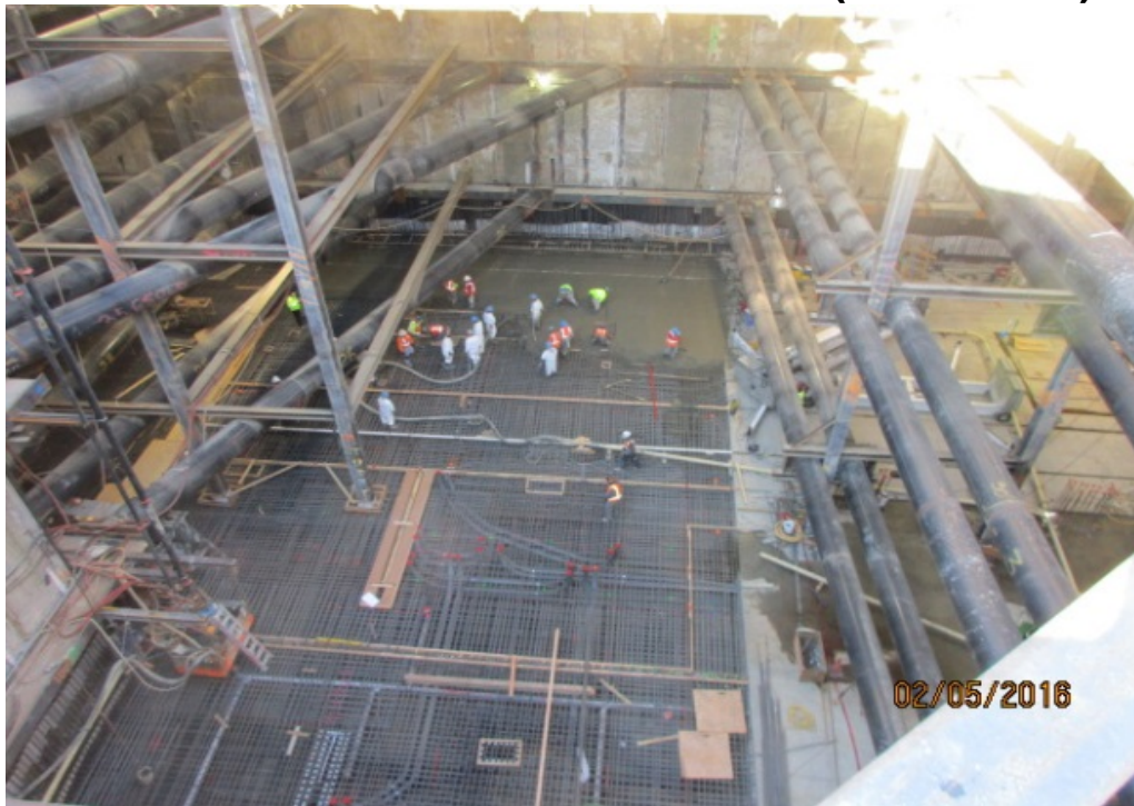
EXPOSITION/CRENSHAW STATION – Rebar installation and preparation for invert concrete placement
