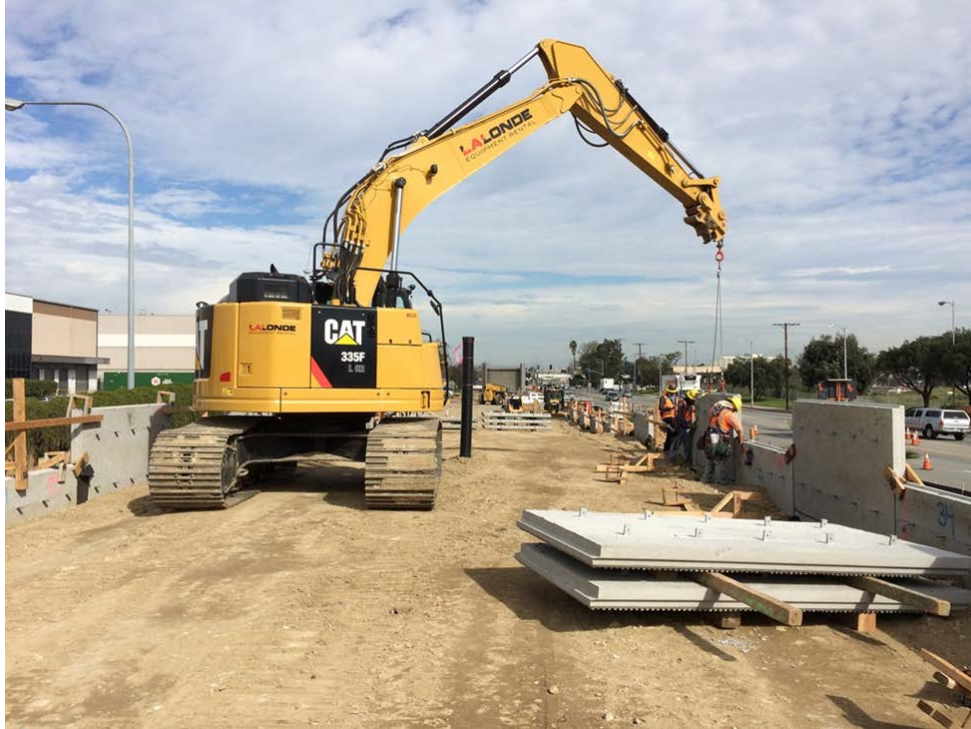
MECHANICALLY STABILIZED EMBANKMENT (MSE) Wall 17L&R - Precast panel erection
