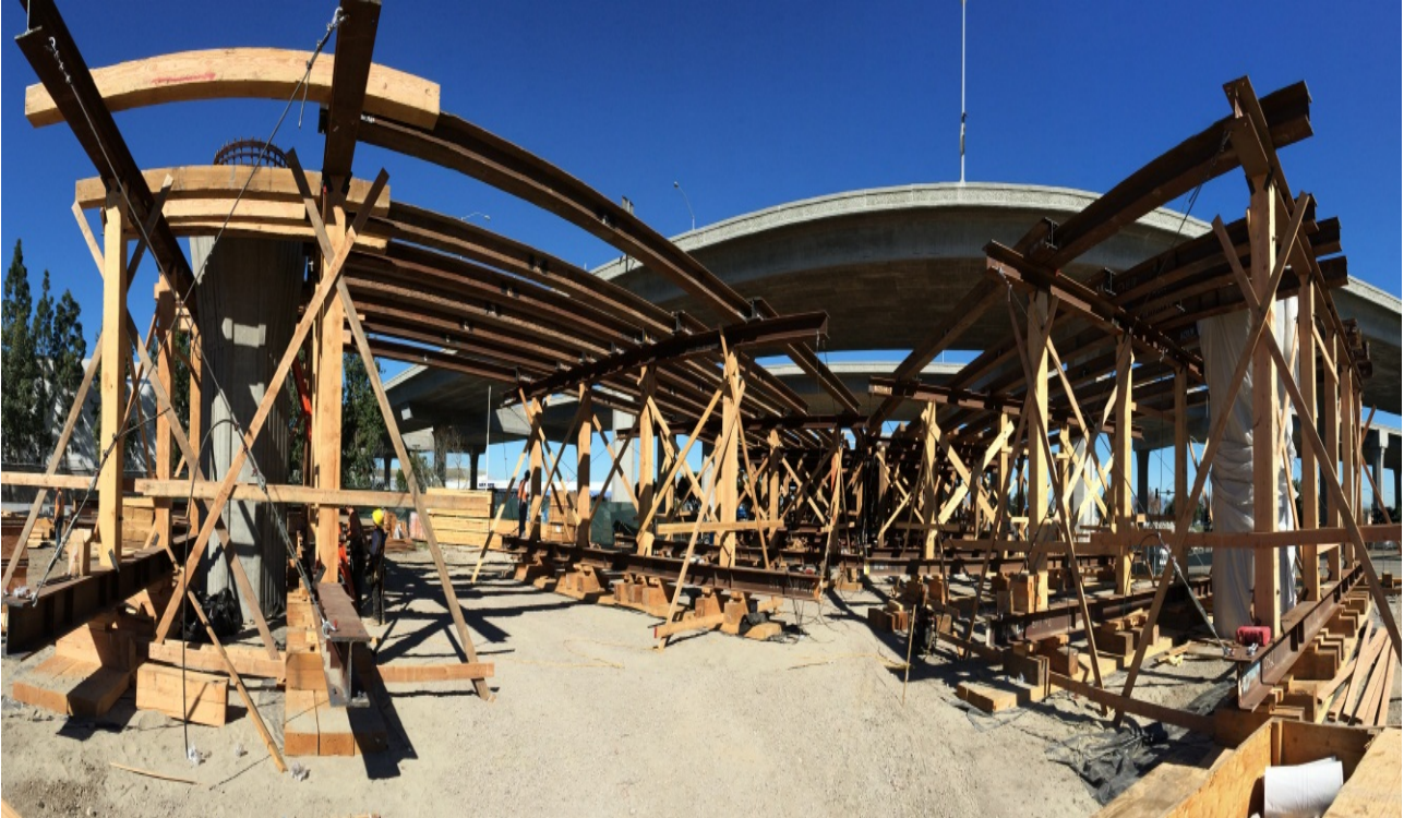
GREENLINE UNDERPASS – Falsework and rolling soffit continue
