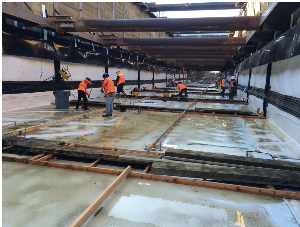
UG1 – Installing waterproof membrane
