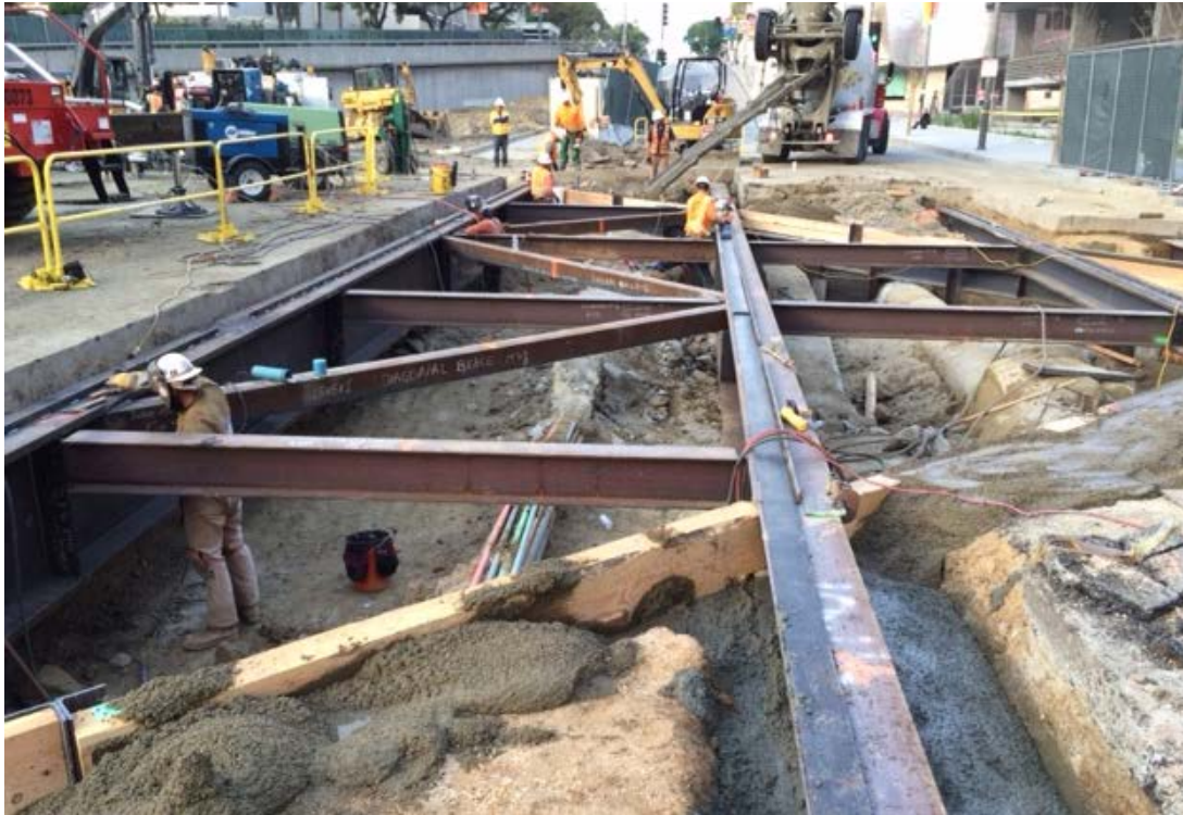
Deck installation at 2 nd /Hope
