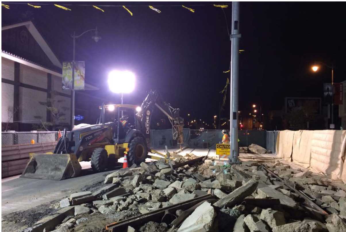
Buddhist Temple Tie-in demolishing at Mangrove Yard
