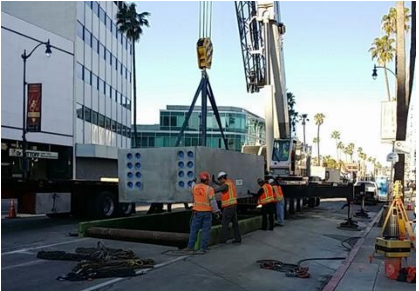
Installation of SCE Electrical Vault West of La Cienega Boulevard
