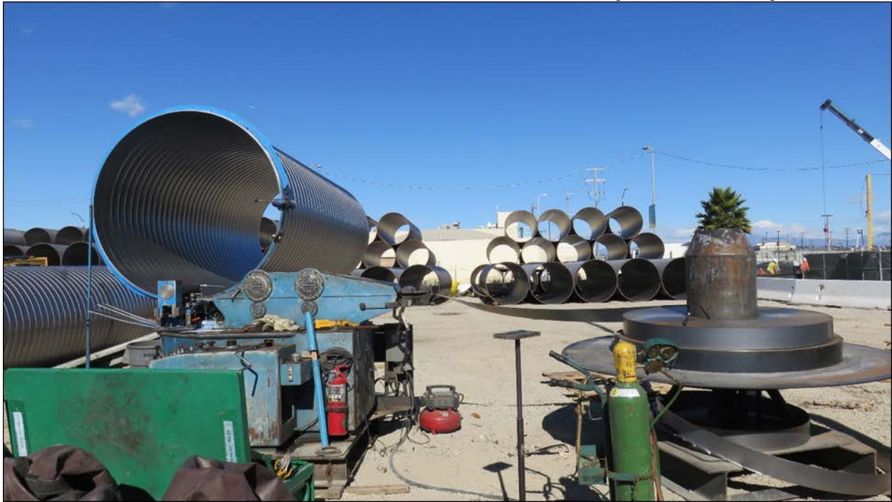
Tunnel ventilation fabrication at Bellanca Yard.
