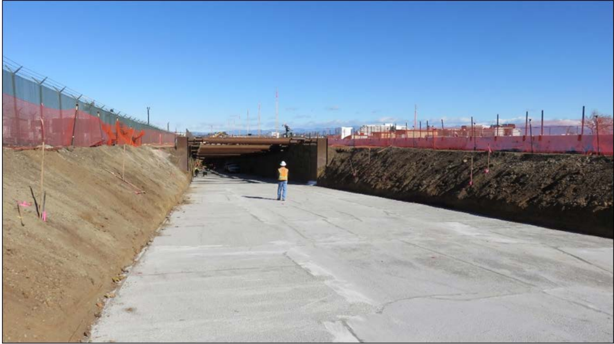
Mud Slab on the South Side of UG1.
