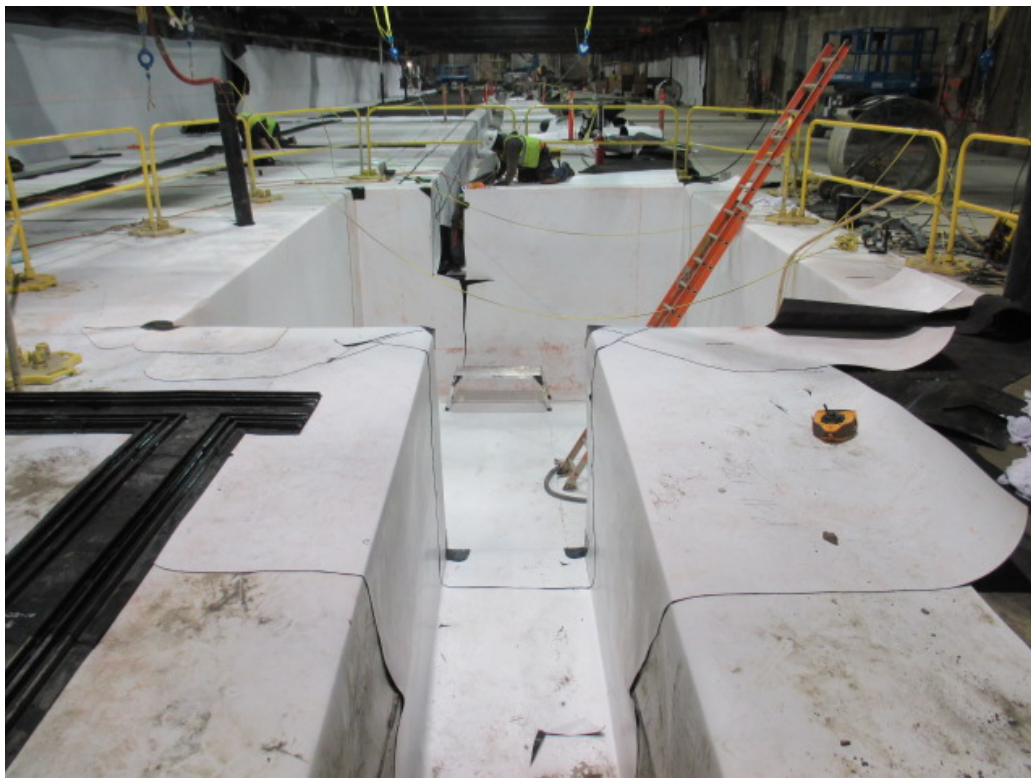
EXPOSITION/CRENSHAW STATION – Installation of waterproofing in the sump pit
