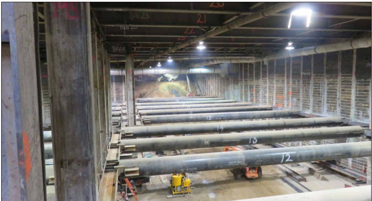
LEIMERT PARK STATION - Looking south with UG4 in the background.
