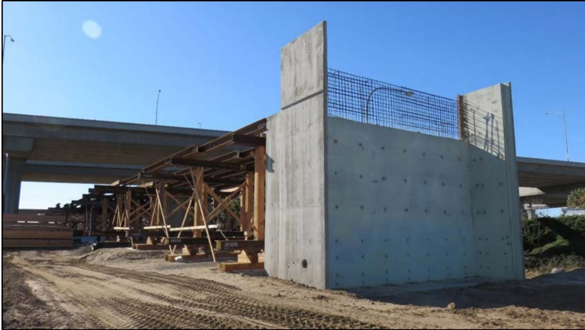
Completed (North) Abutment and Falsework.
