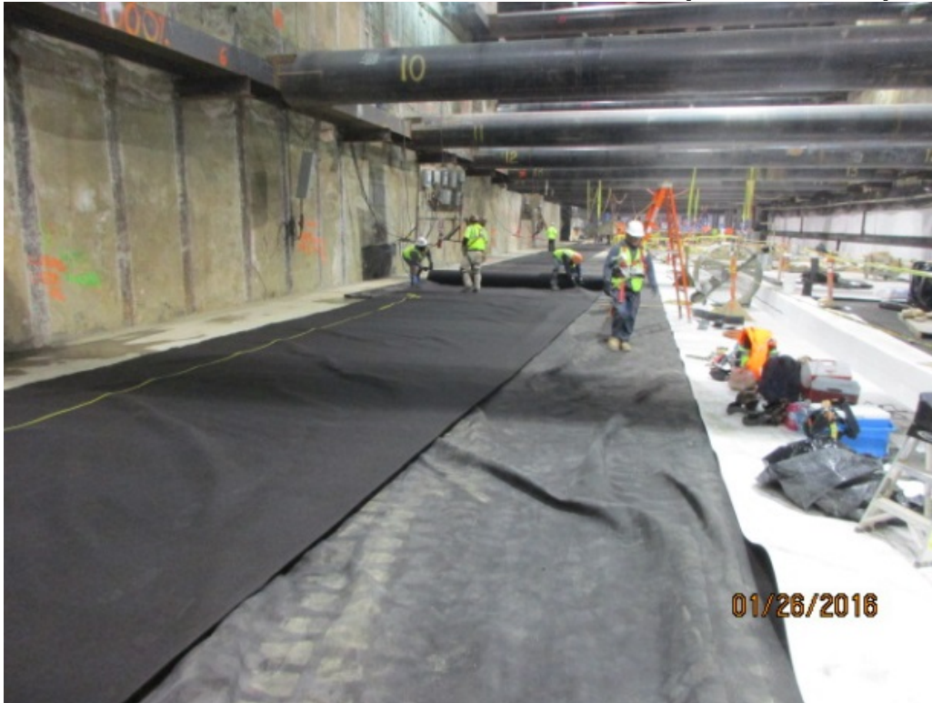
EXPOSITION/CRENSHAW STATION – Installation of waterproofing components
