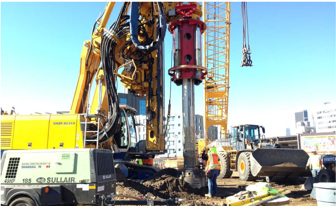
Pile installation at 1 st /Central Station
