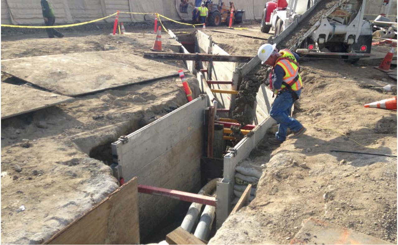
Backfill ductbank at 1 st /Hewitt
