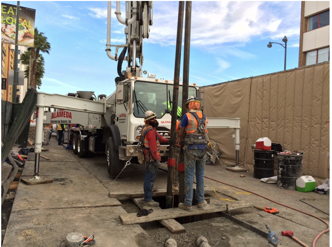
C1045 Contractor Slurry Backfill for Pile #106 at Wilshire/La Brea Station
