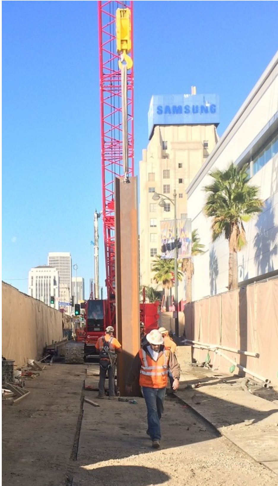
C1045 Contractor Installing Pile #106 at Wilshire/La Brea Station
