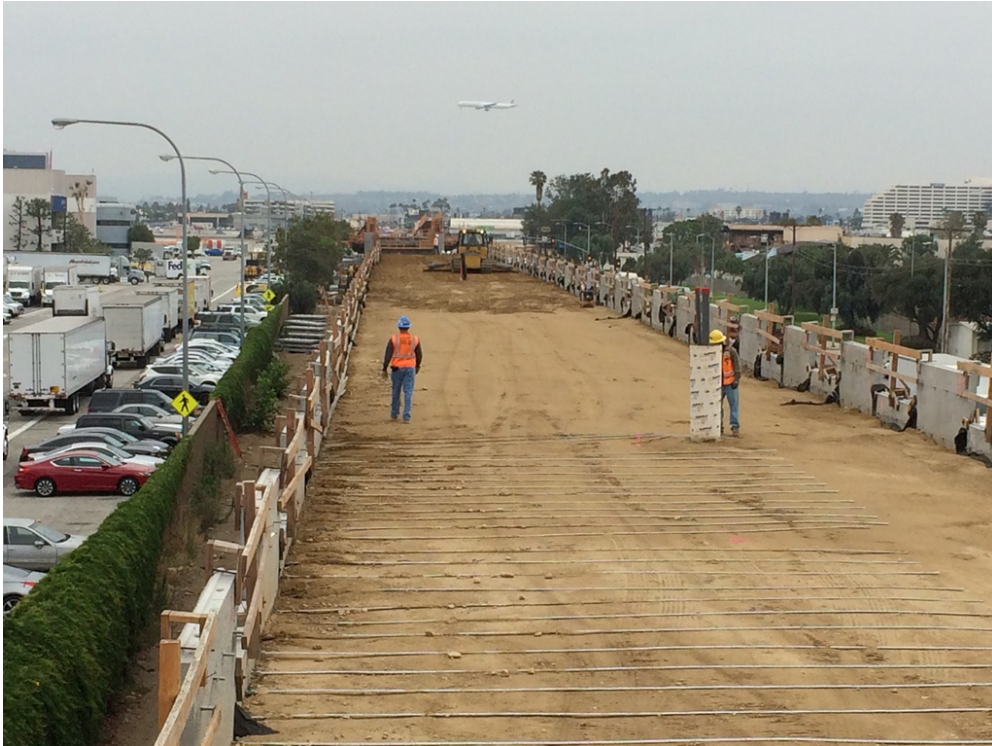
MSE Wall 17L&R (North of Imperial Highway): Crews worked on galvanized strap placement, embankment backfill and compaction.
