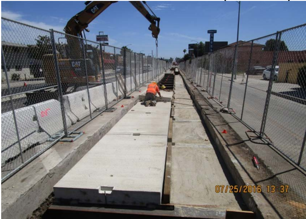
UG#3 – Installation of west side deck panels.
