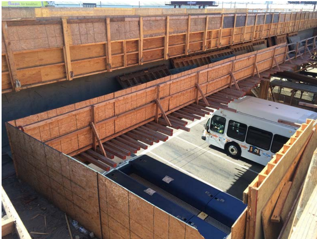
AVIATION/CENTURY BRIDGE – Exterior girder formwork removed in Frame 1A.
