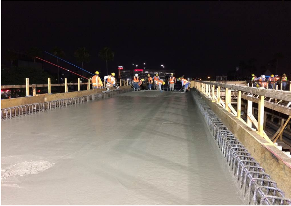
AVIATION/CENTURY BRIDGE – Frame 1A deck concrete placement.
