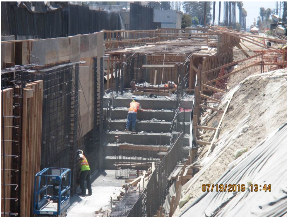
FAIRVIEW HEIGHTS STATION - Crews continued installing rebar and formwork for Southern retaining wall for the subterranean TC&C room.
