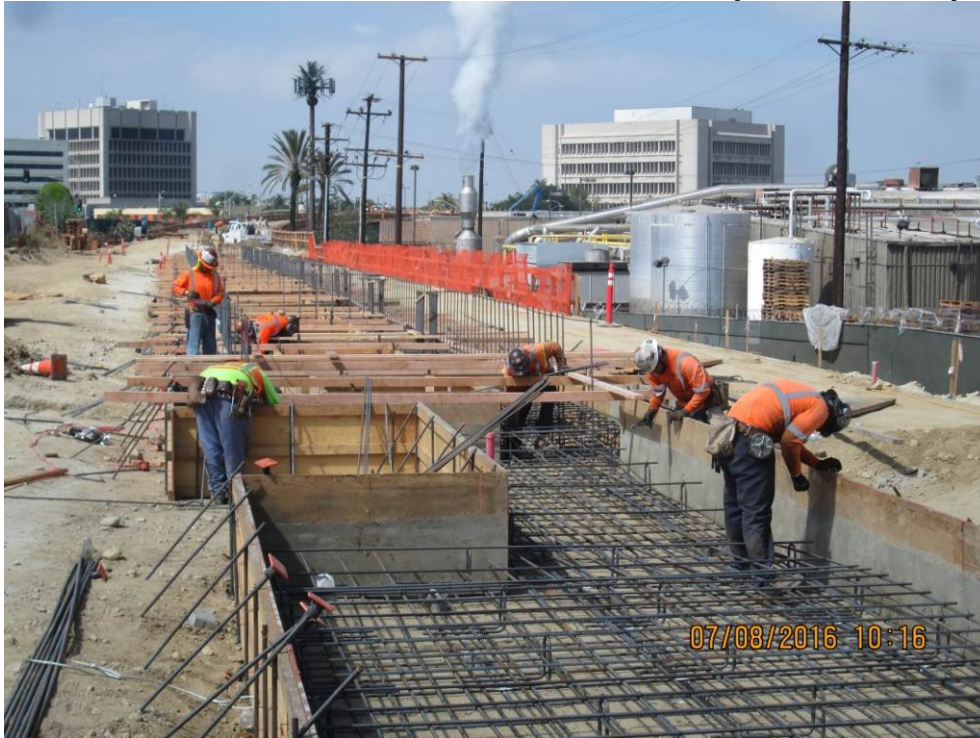
DOWNTOWN INGLEWOOD STATION - Crews worked on installing formwork and rebar for the station's footing and grade beams.
