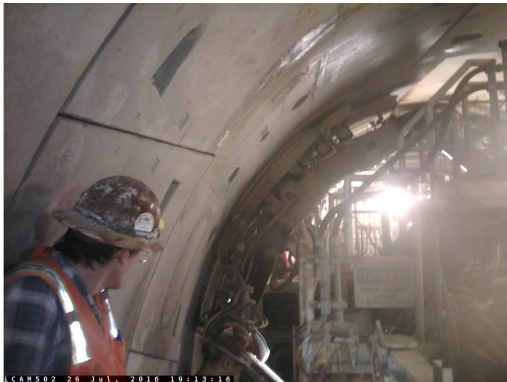
TUNNELING – Setting ring #519.
