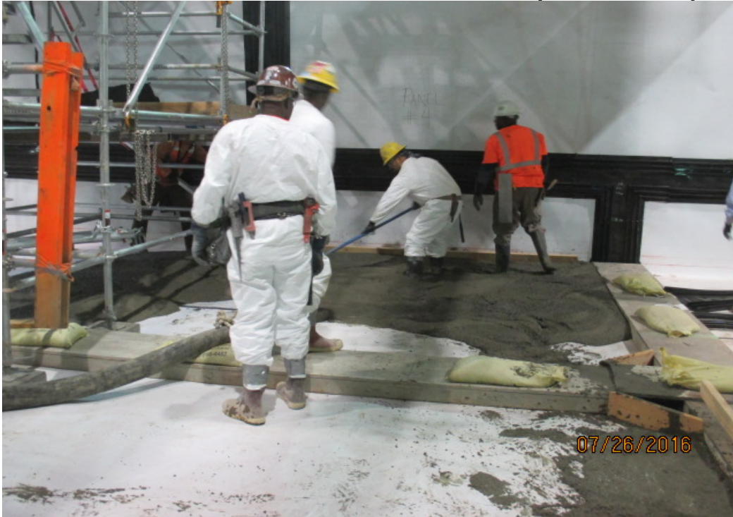
LEIMERT PARK STATION - Placement of protection slab at east side of station box.
