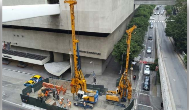
Piling setup at 4 th /Flower
