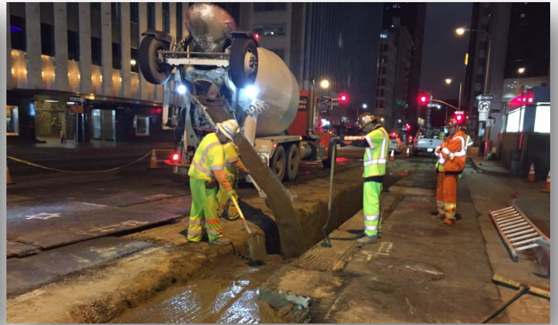
Slurry backfill over welded steel pipe on Flower Street
