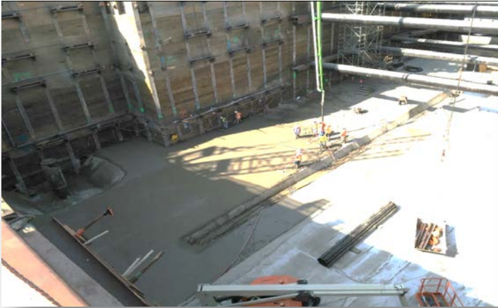
Pouring mud mat at 1 st /Central Station
