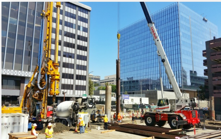
Piling at 2 nd /Broadway Intersection
