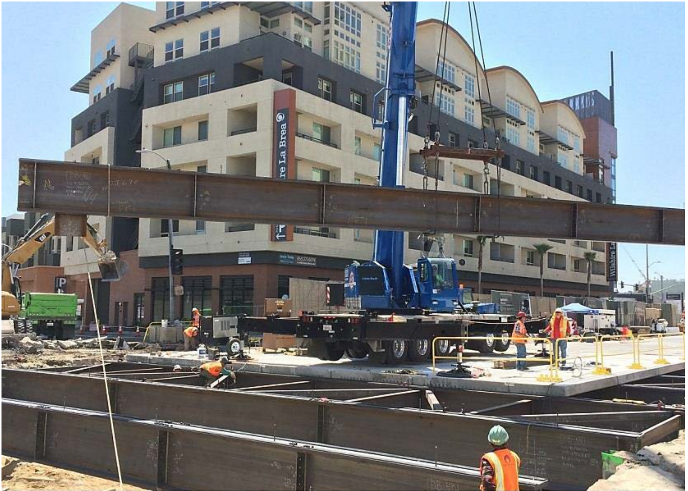
C1045 Contractor Installing Deck Beam at Wilshire/La Brea Station
