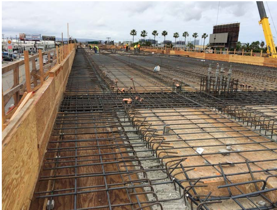
AVIATION/CENTURY BRIDGE – Frame 1 deck rebar installation.
