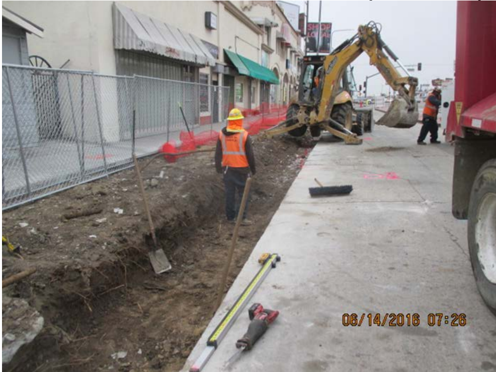
PARK MESA HEIGHTS – Excavating for curb and gutter.
