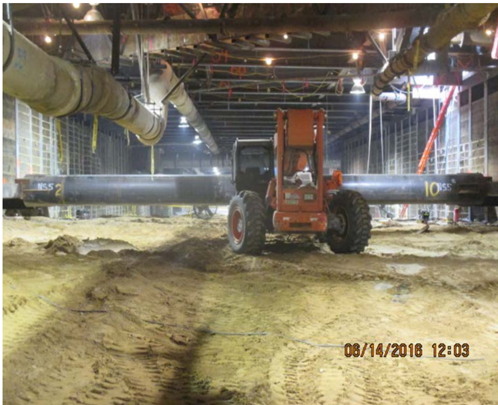
UG#4 – Staging struts.
