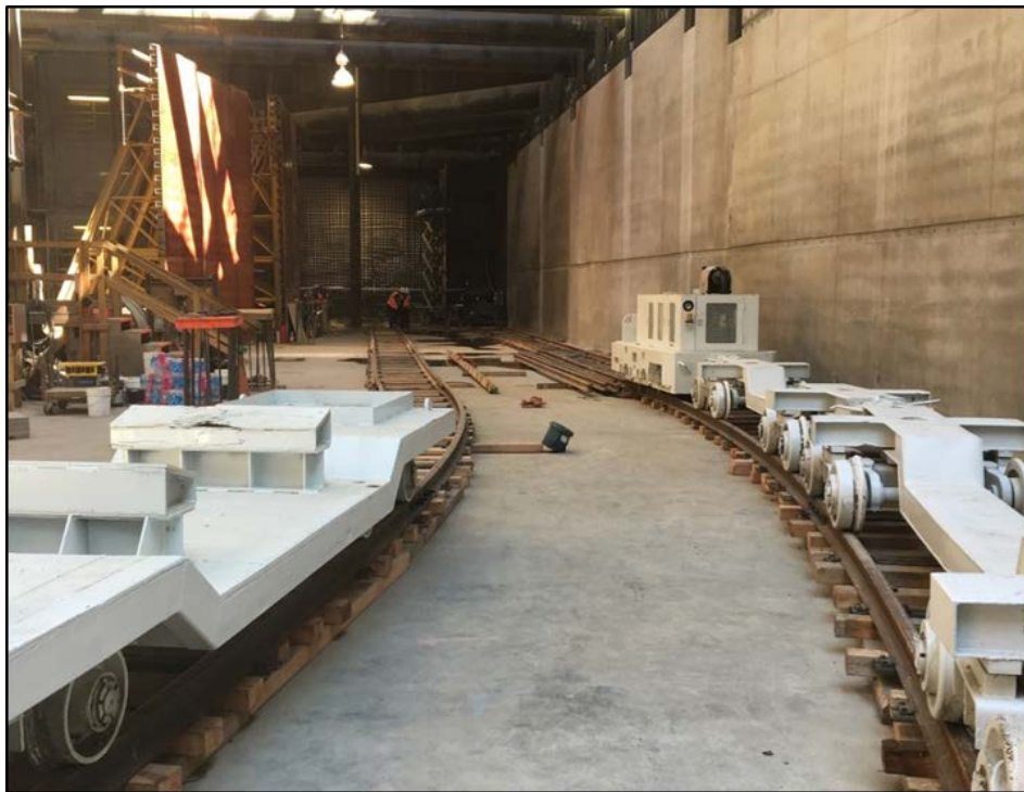
TUNNELING – Muck cars and segment cars on tracks.
