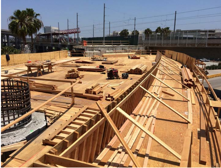
GREENLINE UNDERPASS – Soffit, exterior girder and overhang formwork placement ongoing.
