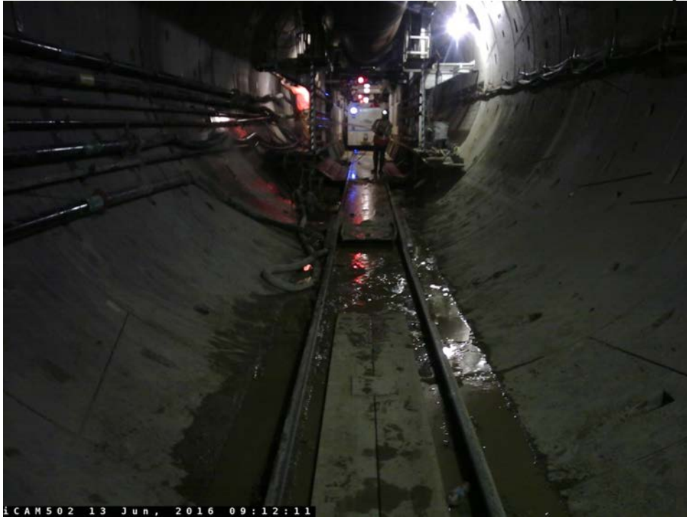
TUNNELING – Looking south into the southbound tunnel.
