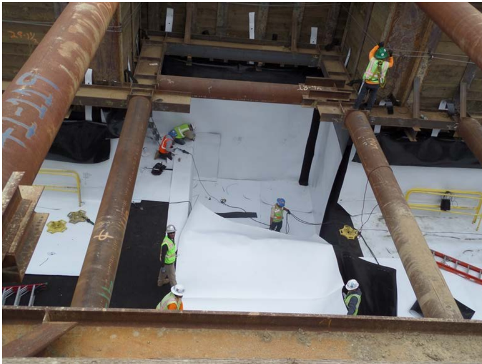
UG#1 – Waterproofing (HDPE) installation at Sump Pump #2.
