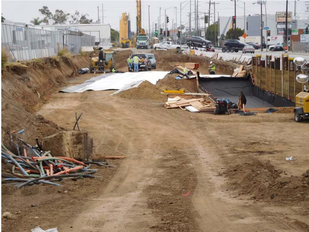
WESTCHESTER STATION – Mass excavation and fine grading for the station footing.
