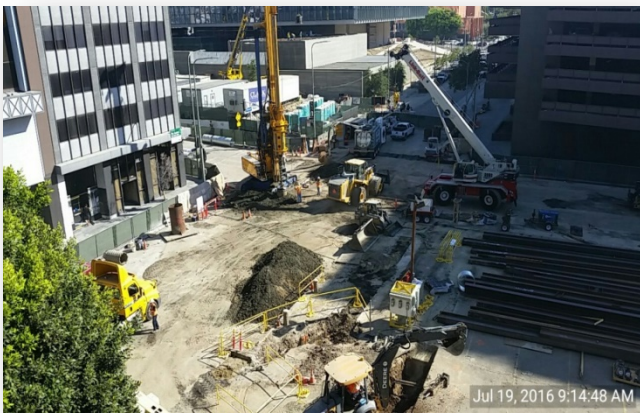
Piling at 2nd/Broadway Hammer Head
