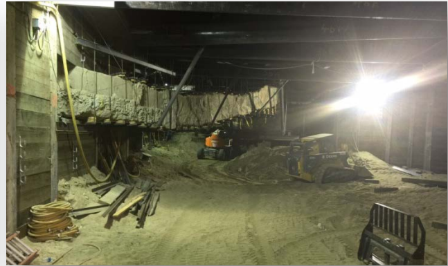
Utilities Under Wye Decking
