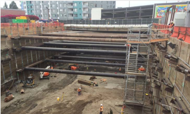
1st/Central Station Excavation
