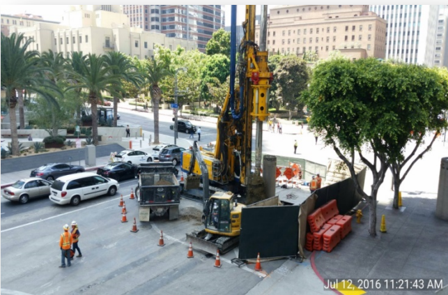
Piling on west side 5th/Flower Street
