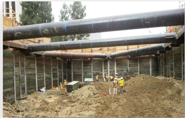
Walers and Struts Installation, Level 1 West Side of Hope Station
