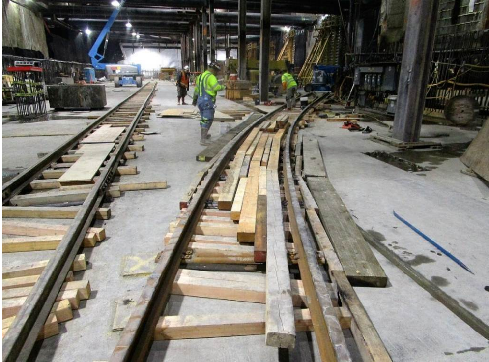
EXPOSITION STATION – Tunnel construction shaft area rail installation
