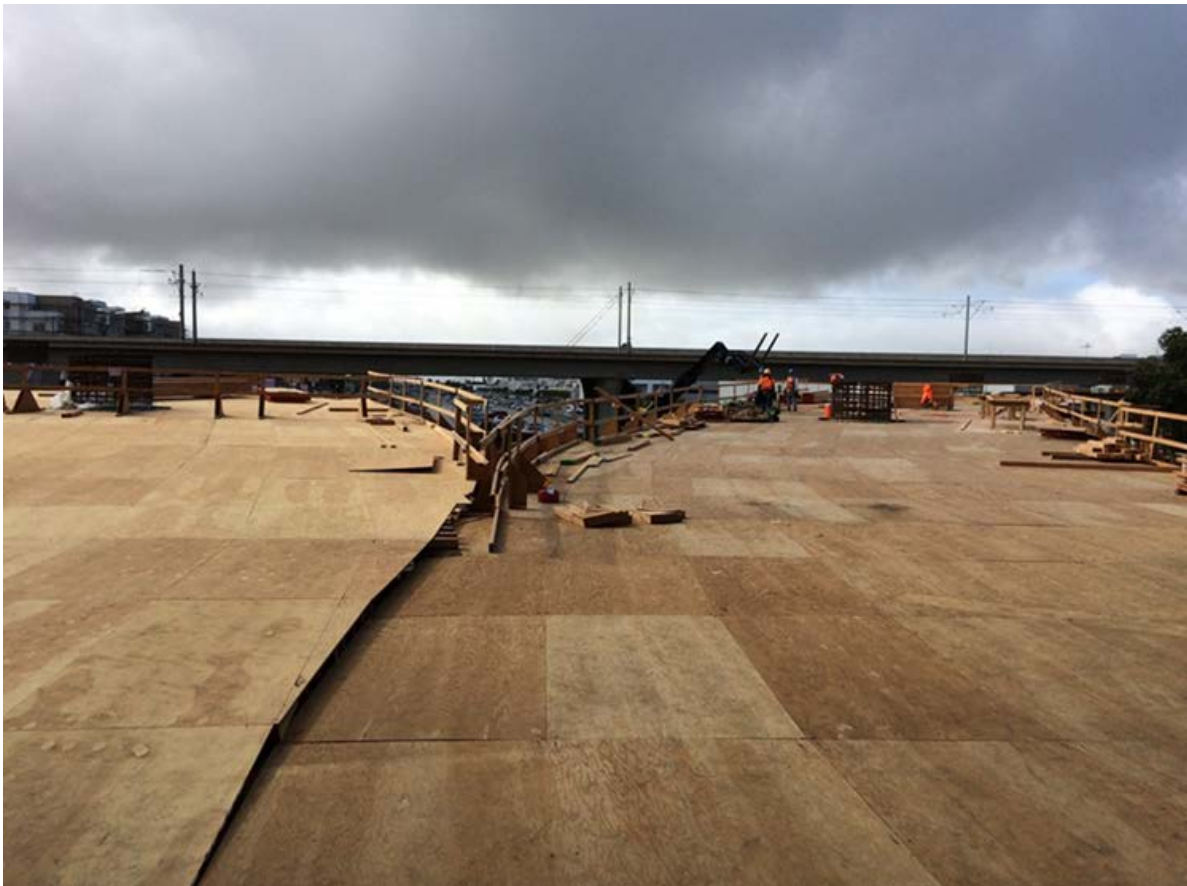
GREEN LINE UNDERPASS (AG-1) Falsework erection and rolling soffit continue
