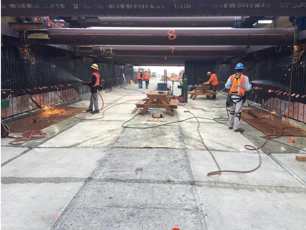
UG1 - Work is progressing.
