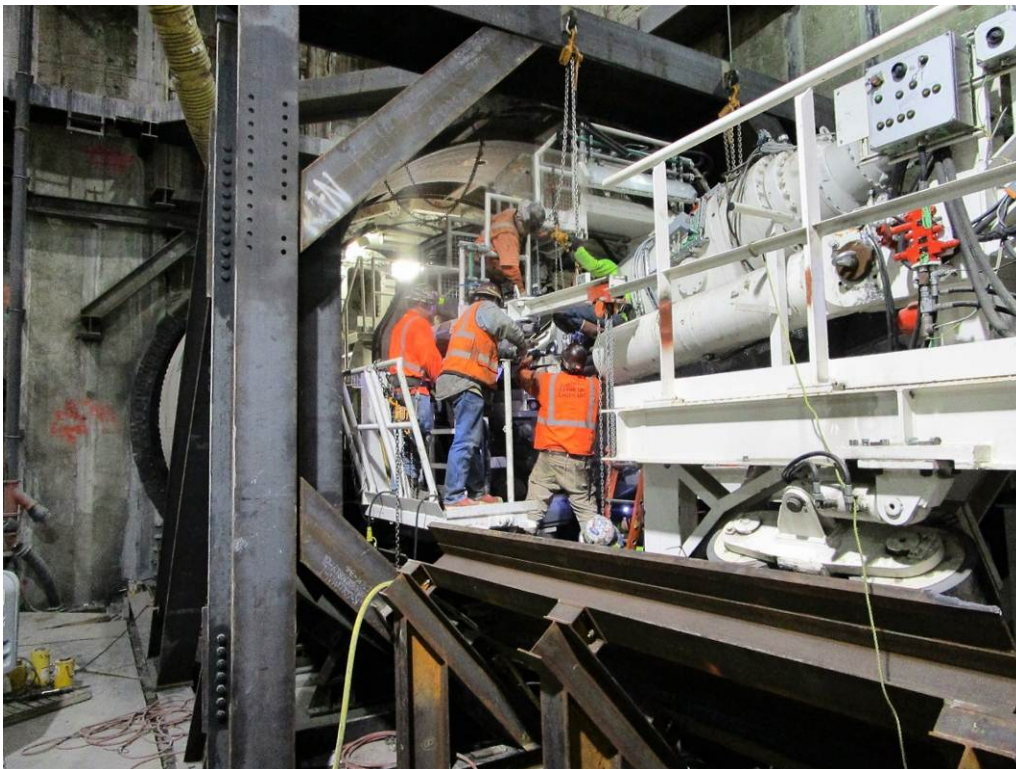
EXPOSITION STATION – Connecting trailing gear tow cylinders to the TBM
