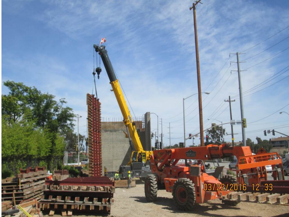
(AG-5) I-405 BRIDGE - Abutment 1 form-cured and stripped.
