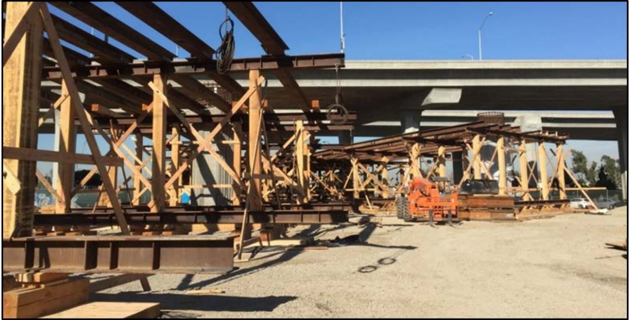
GREEN LINE BRIDGE - Falsework passing below I-105
