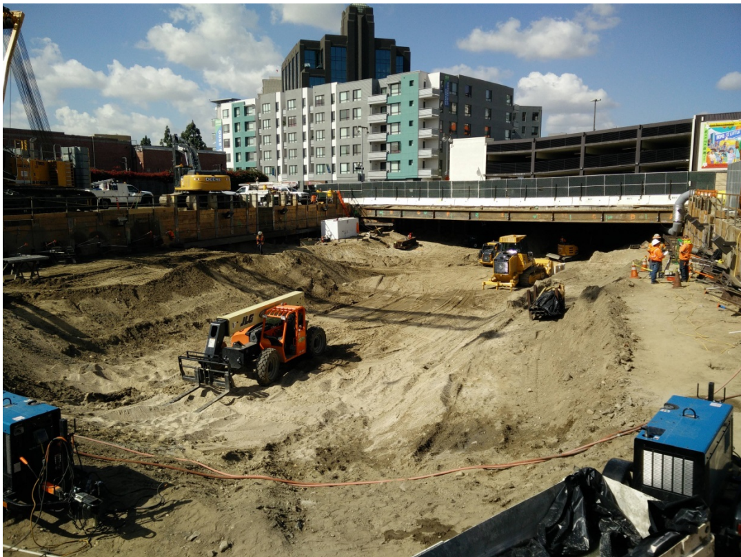
1 st /Central Station construction activities
