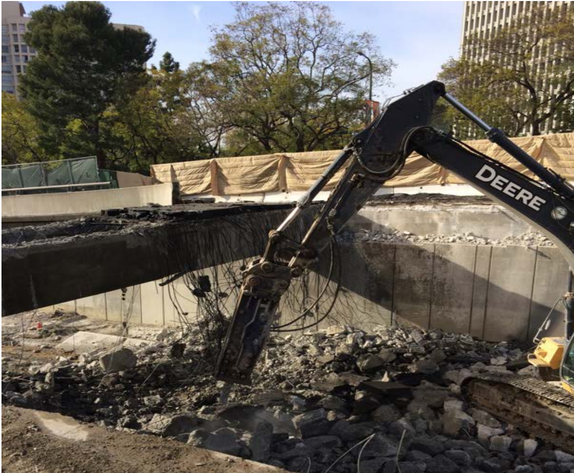
Bridge demolition at 2 nd /Hope
