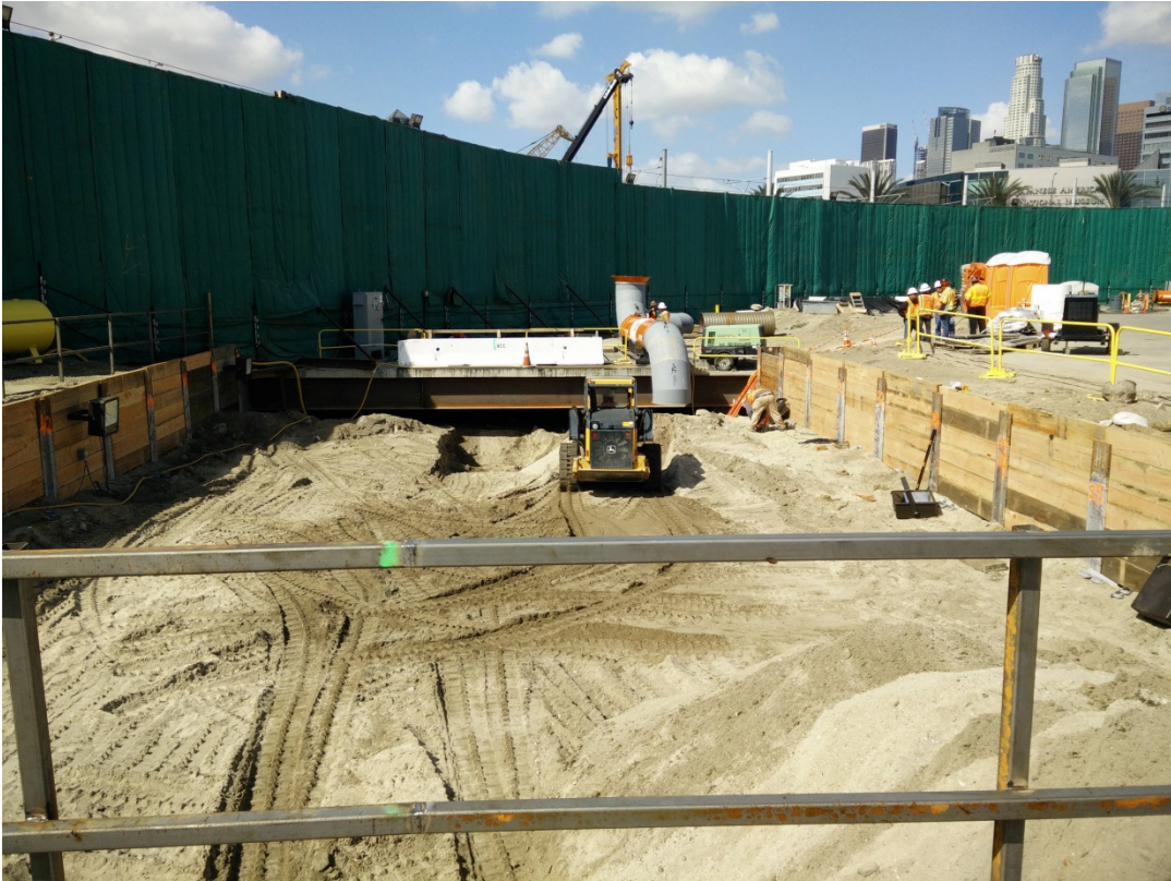
TBM Pit/Wye Excavation
