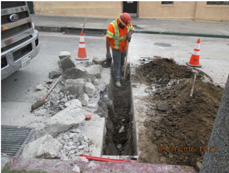
PARK MESA HEIGHTS – New electrical utility placement.
