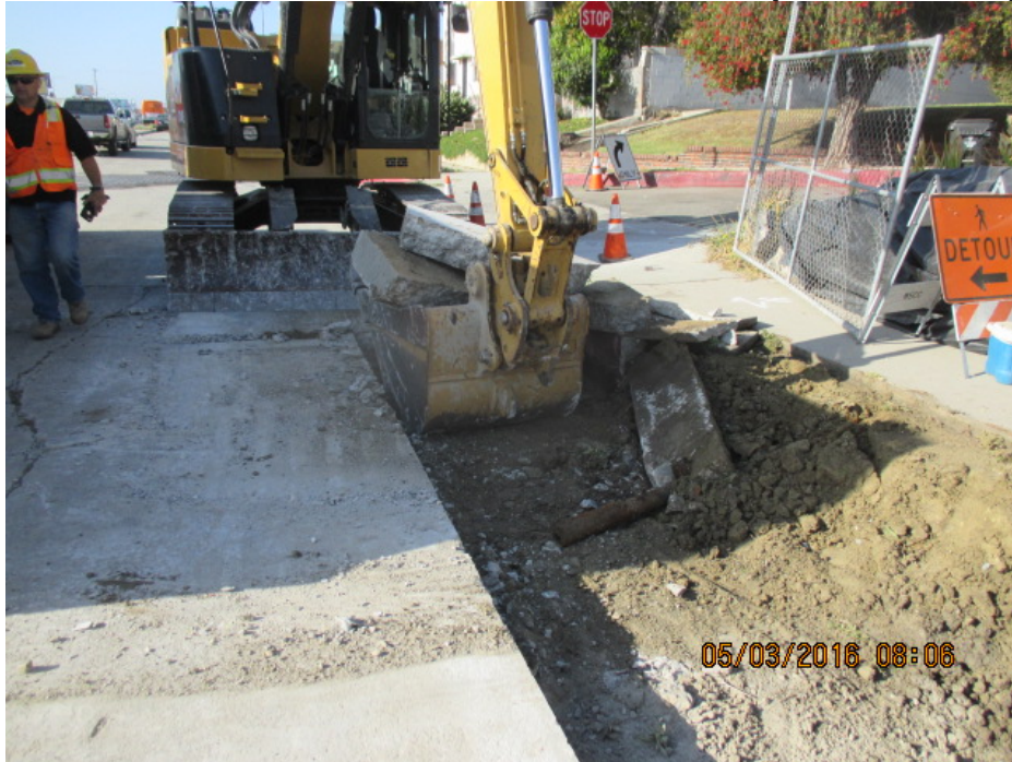
PARK MESA HEIGHTS – Demolition of curb, sidewalk, and street.
