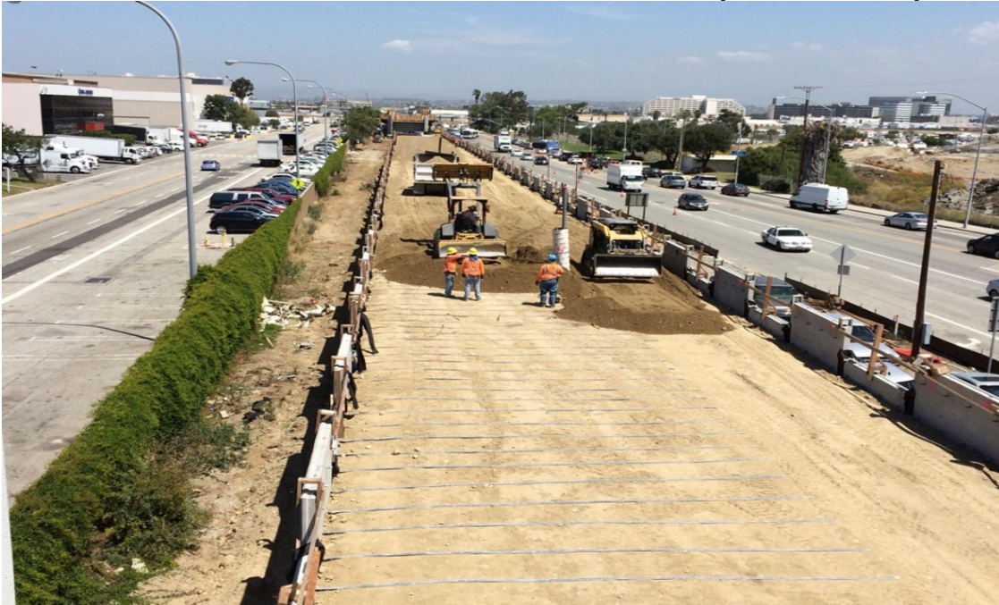
MSE WALL 17L&R (North of Imperial Highway): Subgrade preparation, leveling pad placement, precast panel erection, galvanized strap placement, embankment backfill and compaction testing ongoing.
