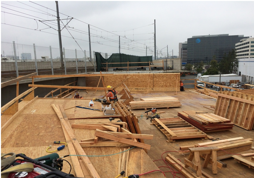
GREENLINE UNDERPASS – Falsework erection complete; formwork placement, soffit exterior girder and overhang formwork placement continues.
