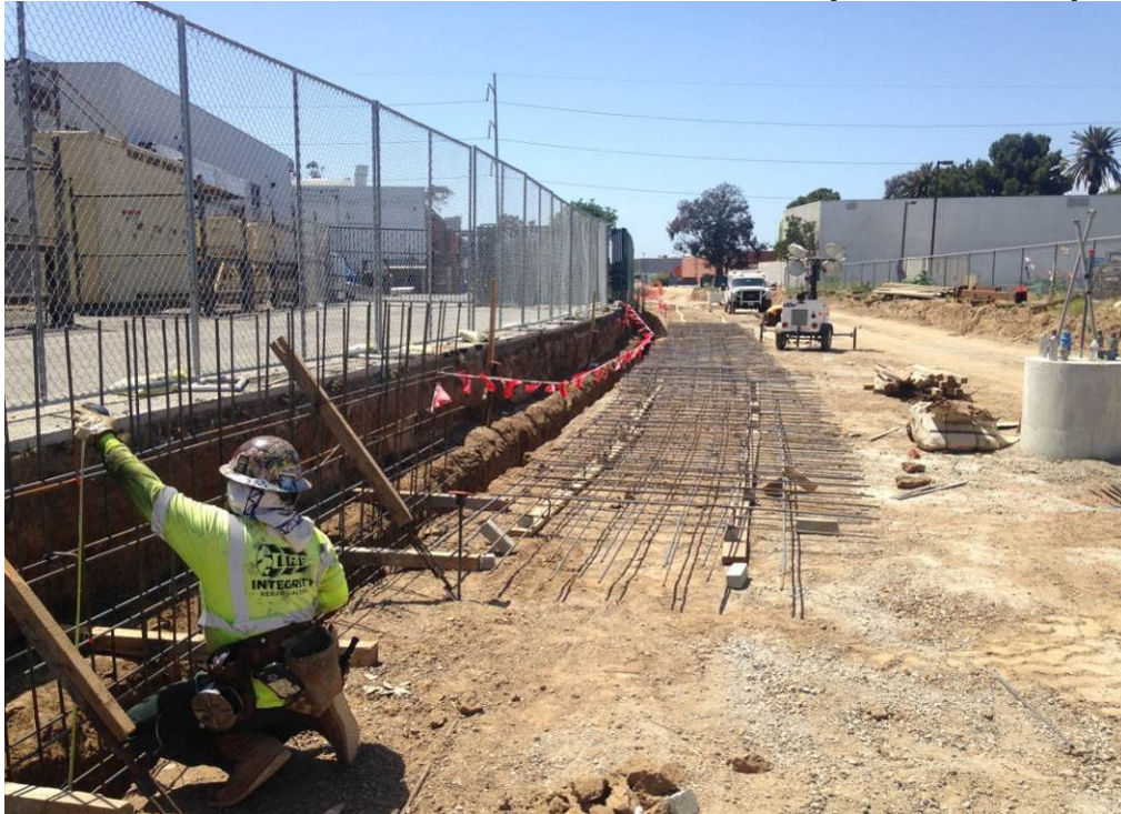
SEGMENT A – Ballast retainer wall construction ongoing.
