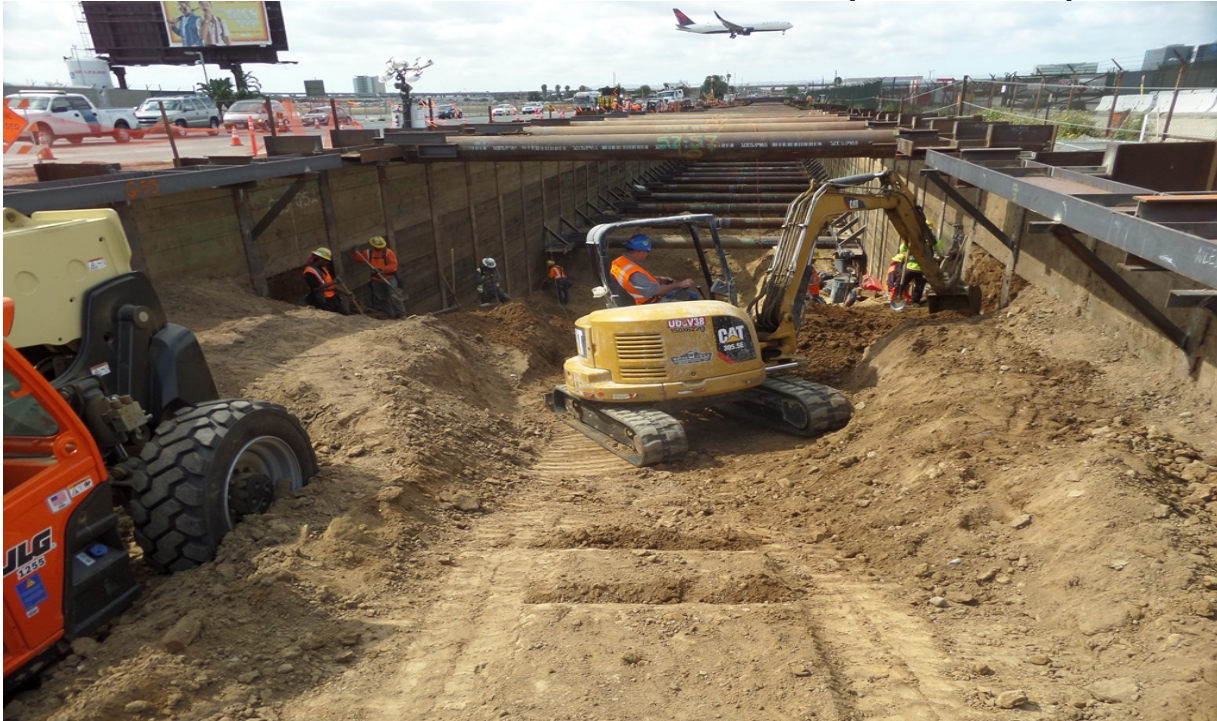
UNDERGROUND GUIDEWAY 1 – Excavation bracing and lagging installation continues at the north end.
