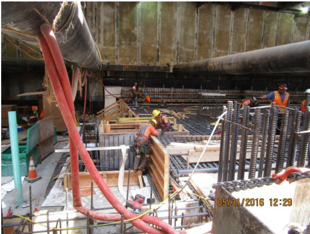
MARTIN LUTHER KING JR. STATION – Installation of electrical conduits, plumbing, and rebar at north end of station.
