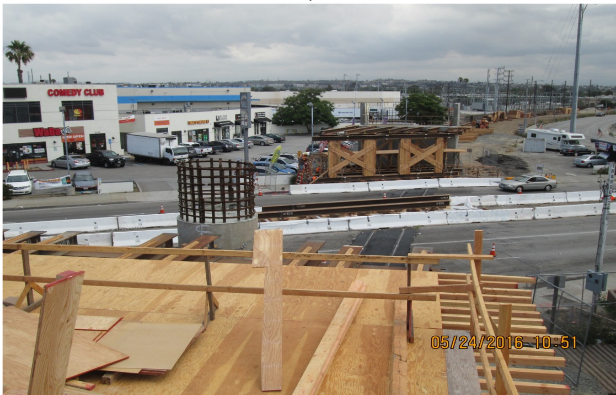
MANCHESTER BRIDGE UNDERPASS – Looking up the station.
