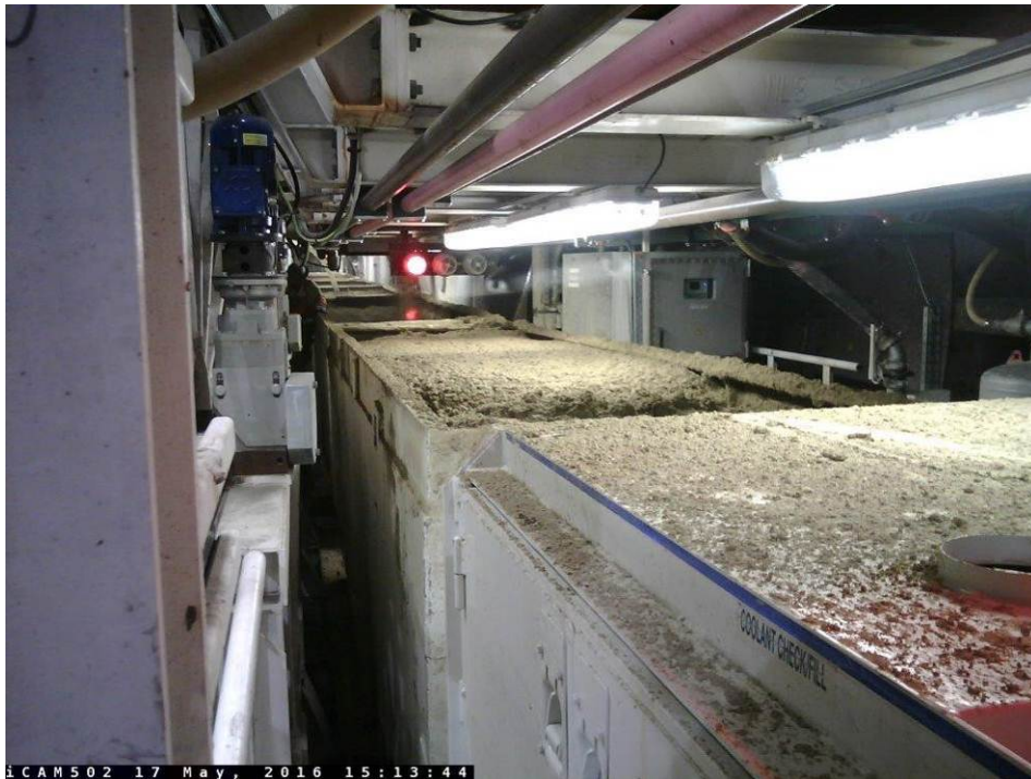
TUNNELING – Removing muck from TBM advance.
