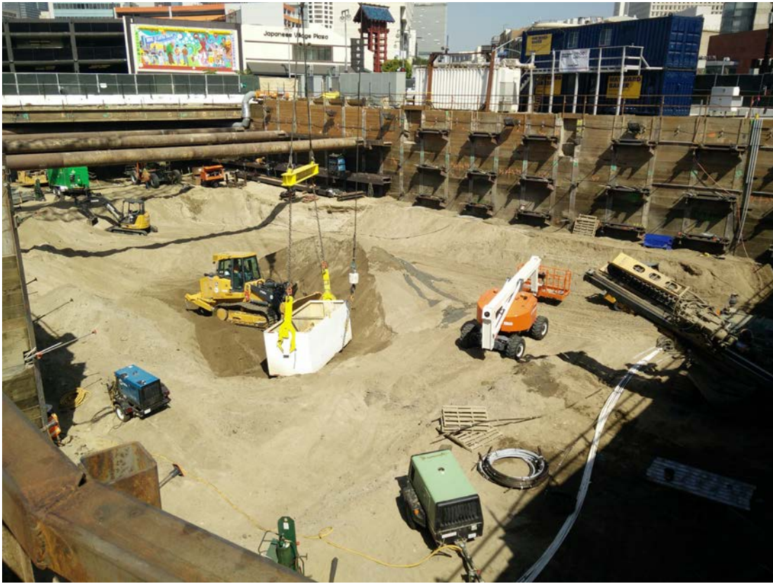
Tieback installation and bracing struts at 1 st /Central Station
