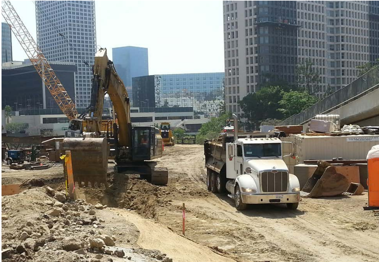
2 nd /Hope construction activities
