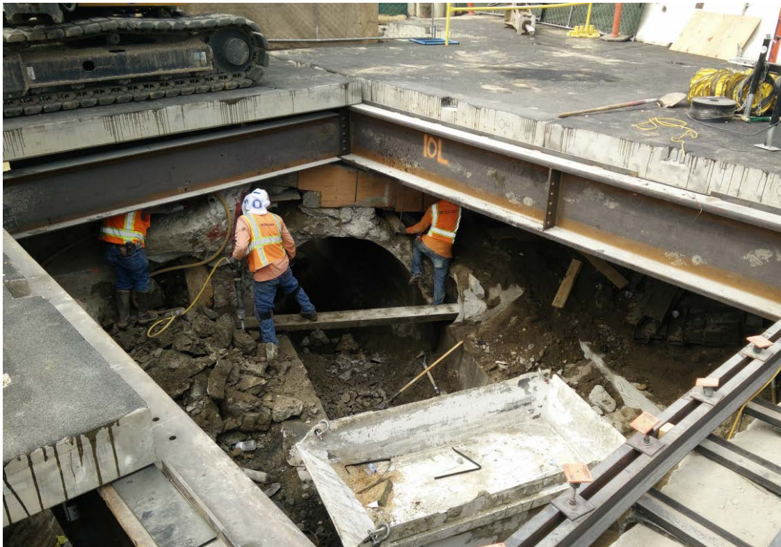
Utility hanging and preparatory work for 69" Hobas storm drain installation
