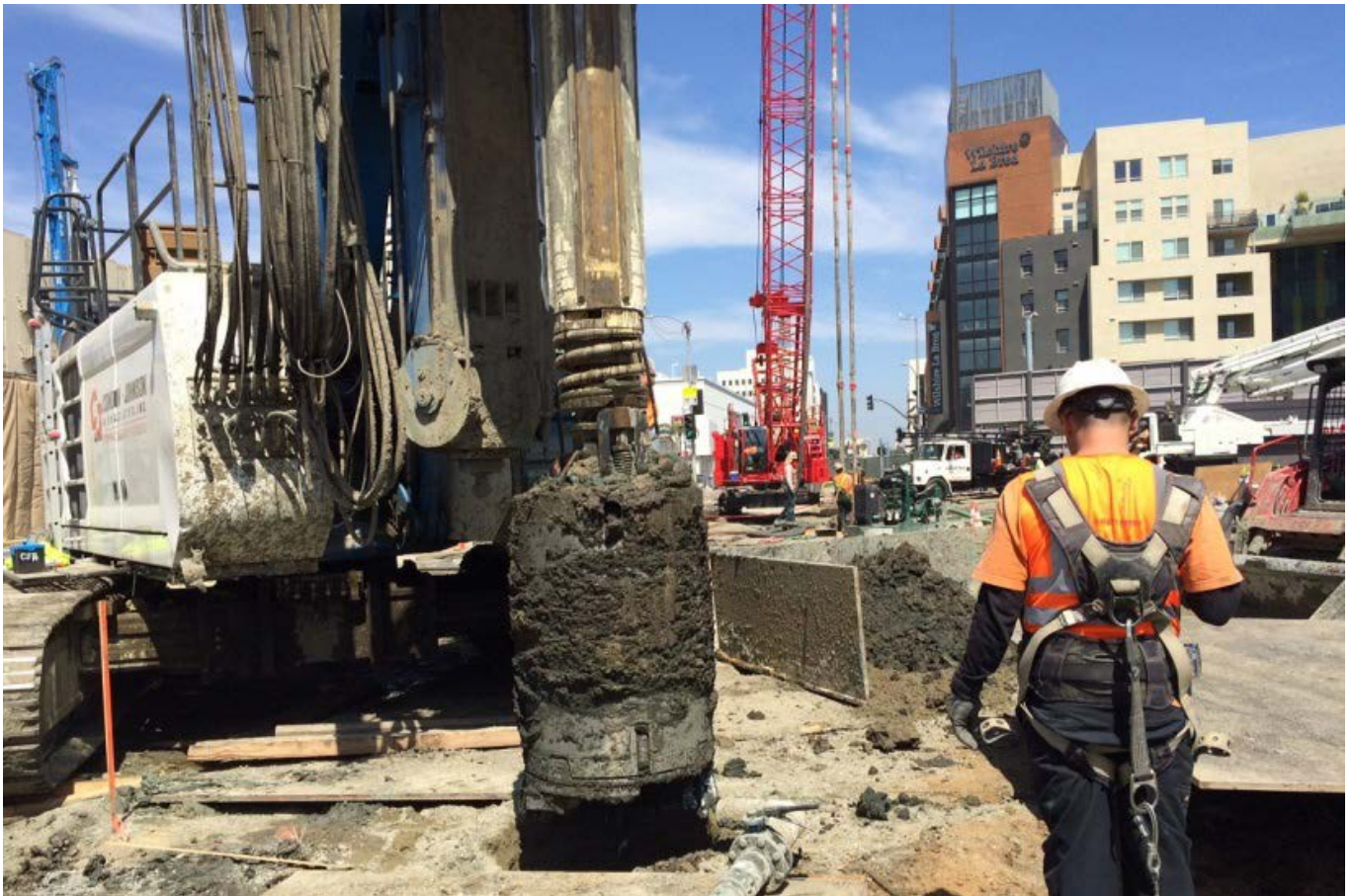
C1045 Contractor Installing Piles South Side Wilshire/La Brea Station
