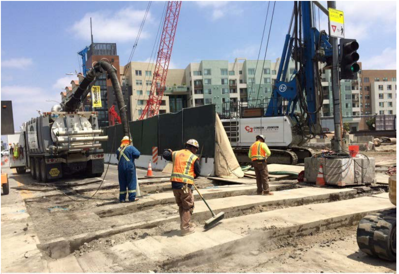
C1045 Contractor Preparation for Jet Grouting Activities at Wilshire/Detroit
