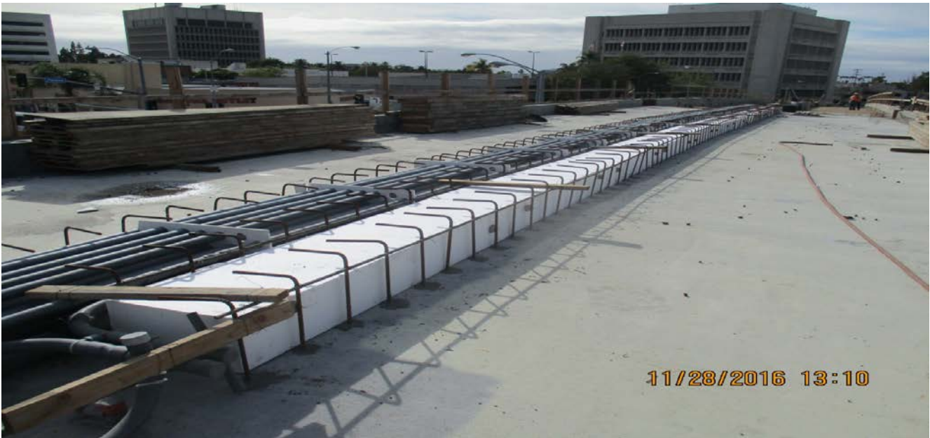
(AG-6) LA BREA BRIDGE – Crews continued to drill and bond the Emergency walkway/ CS ductbank.
