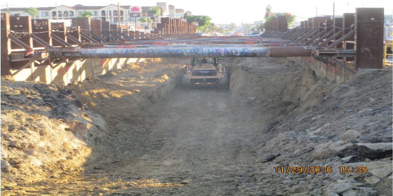
UG#3- Excavating beneath struts at north portal.
