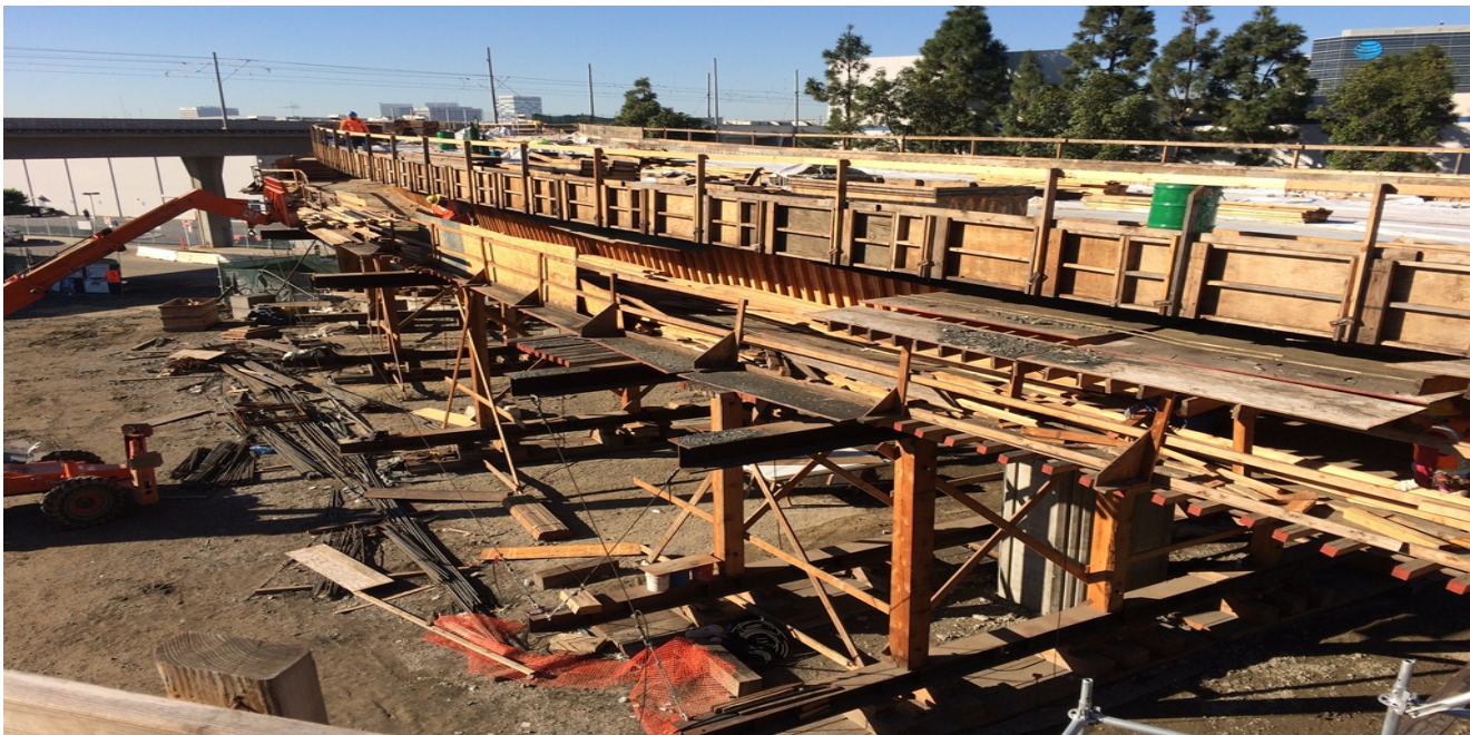
GREENLINE UNDERPASS – Frame A: overhang formwork removed and PT tendons installed by DSI.
