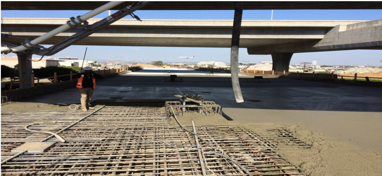
GREENLINE UNDERPASS – Frame 2: Deck concrete placement.
