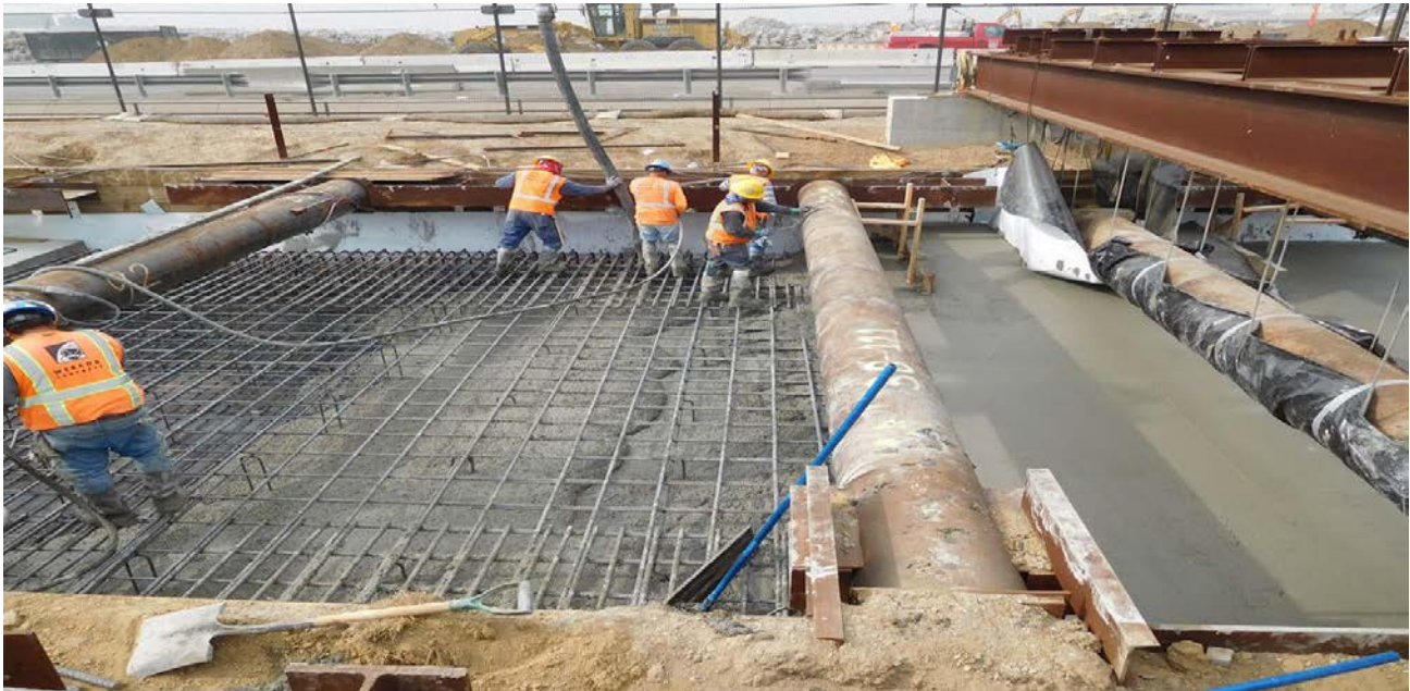
UG#1 – Crews continue with sequential construction at Underground Guideway 1 progressing from south to north.
