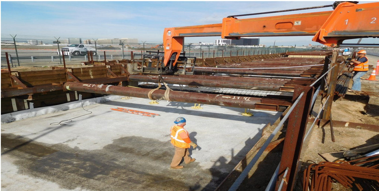
UG#1 Tier 1 SOE strut removals ongoing.
