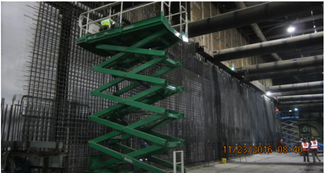
LEIMERT PARK STATION – Installation of rebar along the lower west walls.
