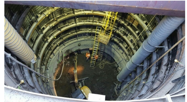
Tie-back removal shaft excavation
