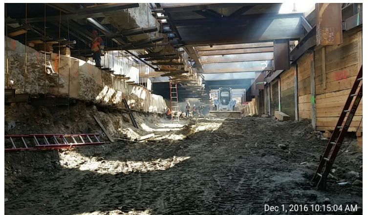
Utility hanging under 2 nd Street decking
