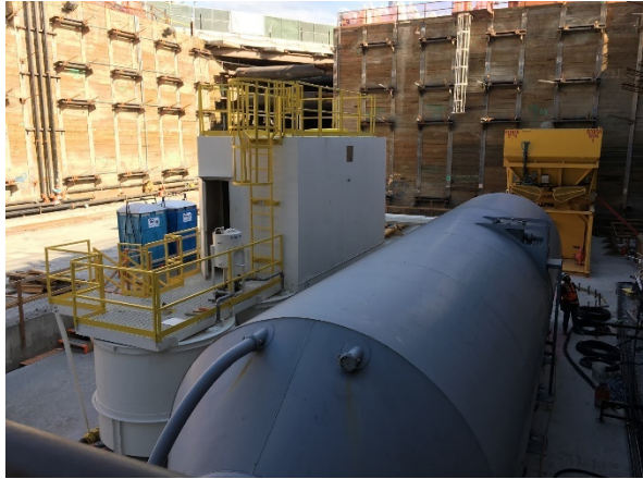
TBM assembly in launch pit (left) Installation of foam and grout plant equipment at 1st/Central Station (right)
