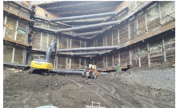
Drilling for Tiebacks Level 5 (top) Assembling Level 4 diagonal struts (bottom)
