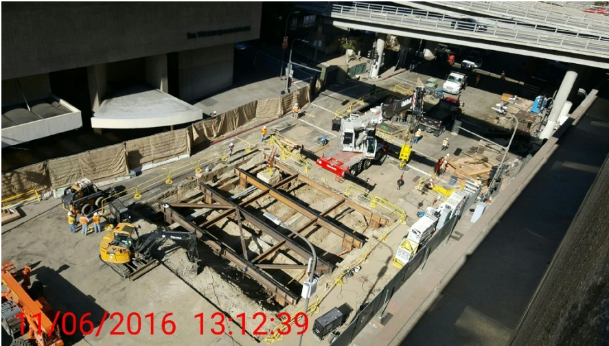
Deck beam installation on 4 th /Flower, during weekend closures
