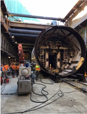
TBM assembly in launch pit (left) Installation of foam and grout plant equipment at 1st/Central Station (right)
