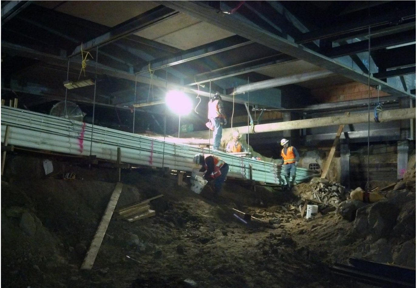
Hanging of Telecom Ductbank under Wilshire/La Brea Station Decking
