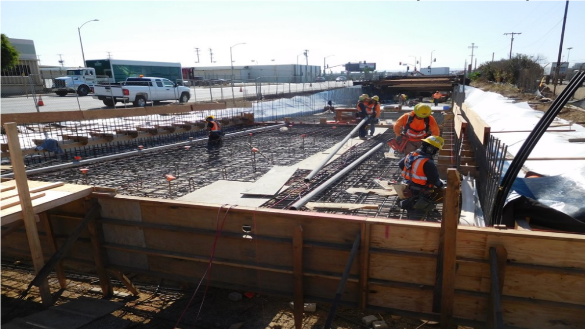
UG#1 -Invert rebar installations at the north end.
