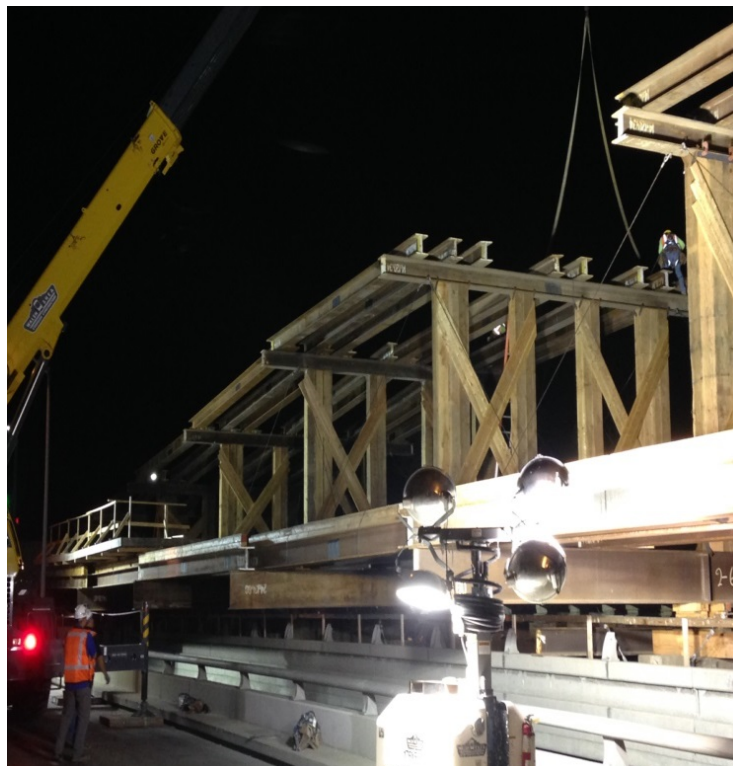
I-405 Bridge –. Bridge superstructure falsework erection ongoing.
