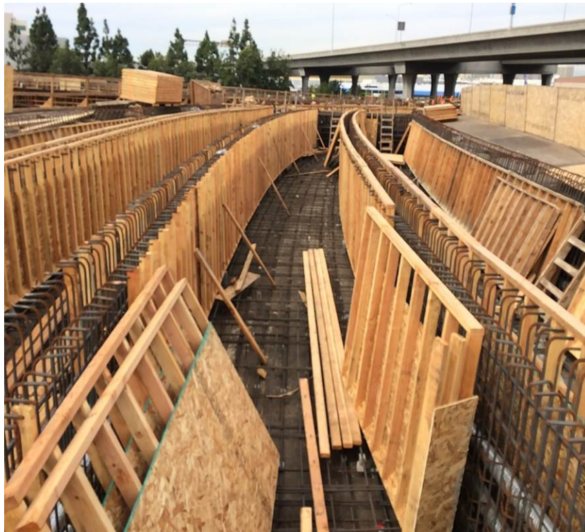
GREENLINE UNDERPASS – Deck rebar installation ongoing/girder-stem formwork installation ongoing.
