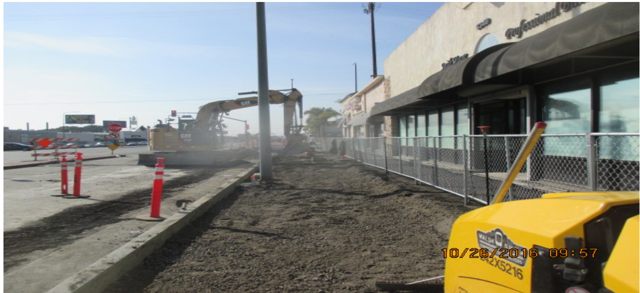
PARK MESA – Placing CMB base section north of 54 th .
