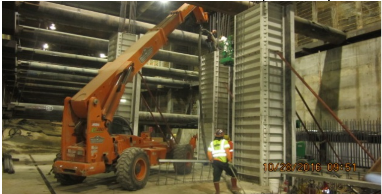
LEIMERT PARK STATION – Installation of invert column shear cap.
