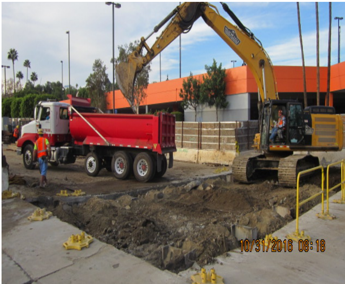
MARTIN LUTHER KING JR. STATION – Start of excavation for side structure.
