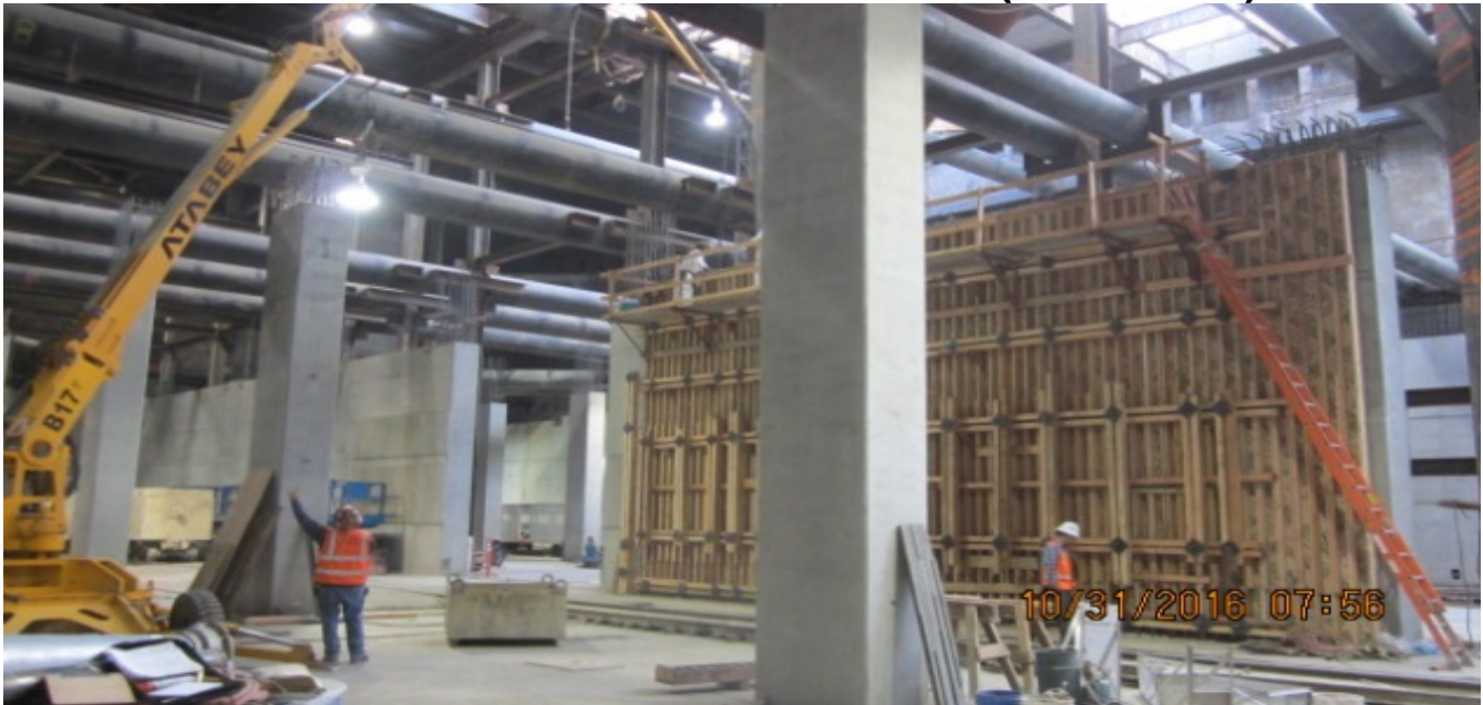
EXPOSITION/CRENSHAW STATION – Placing concrete for interior wall.
