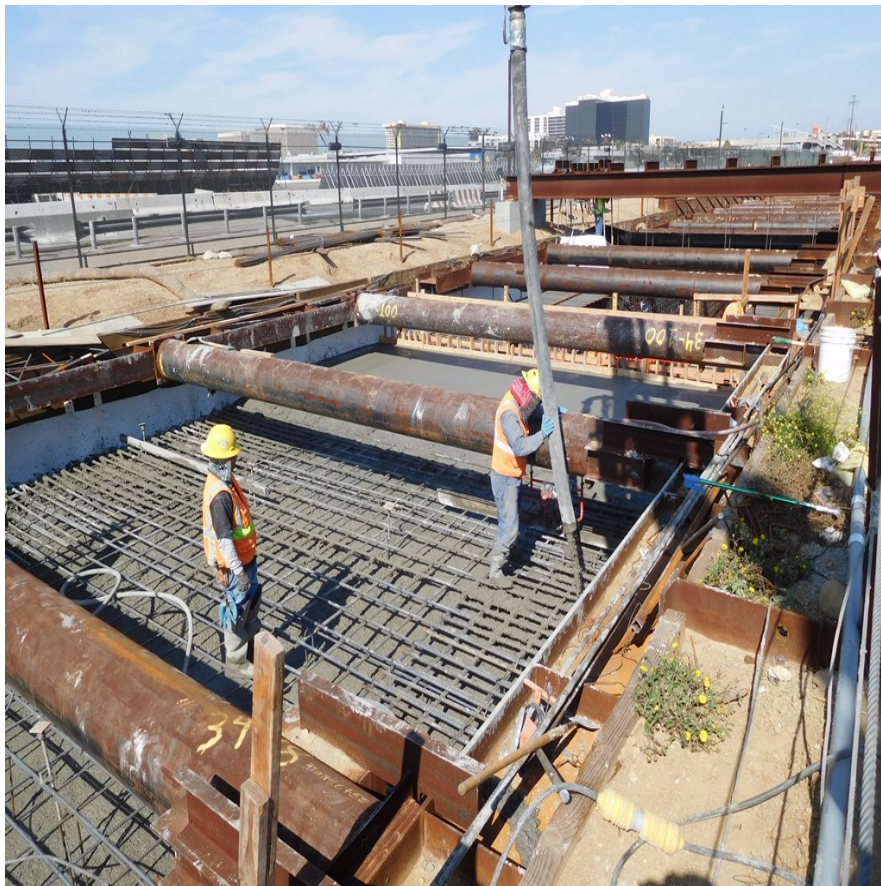
UG#1 - Concrete placement for cut-and-cover tunnel segment.
