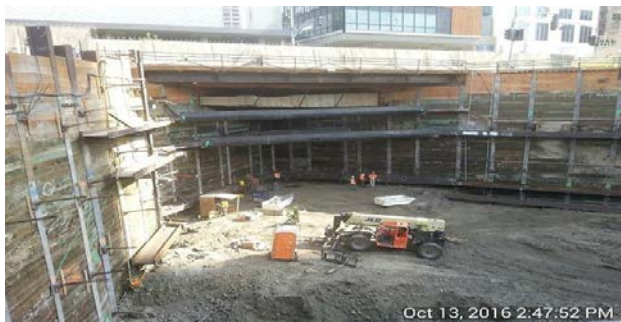
Installation of 3 rd Level walers below Hope Street decking
