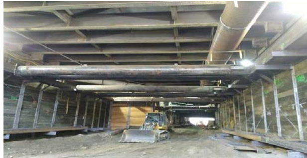
Continued excavation at Wye
