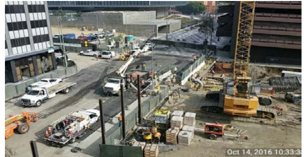
2 nd /Broadway restoration in preparation for street re-opening
