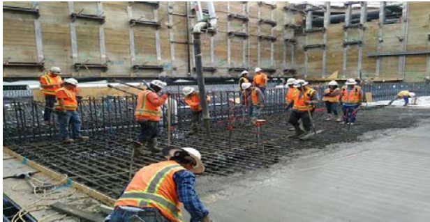
Concrete pours of invert slab
