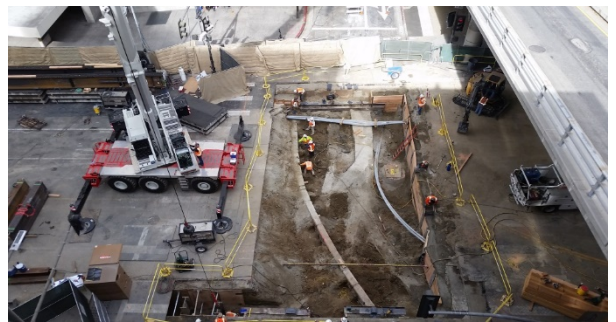
Decking preparations at 4 th /Flower Intersection
