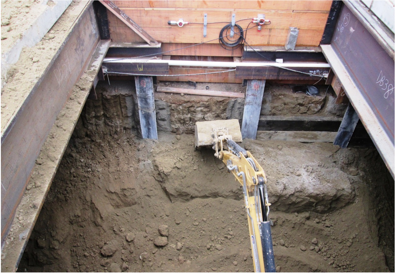
Wilshire/La Brea Station Excavation
