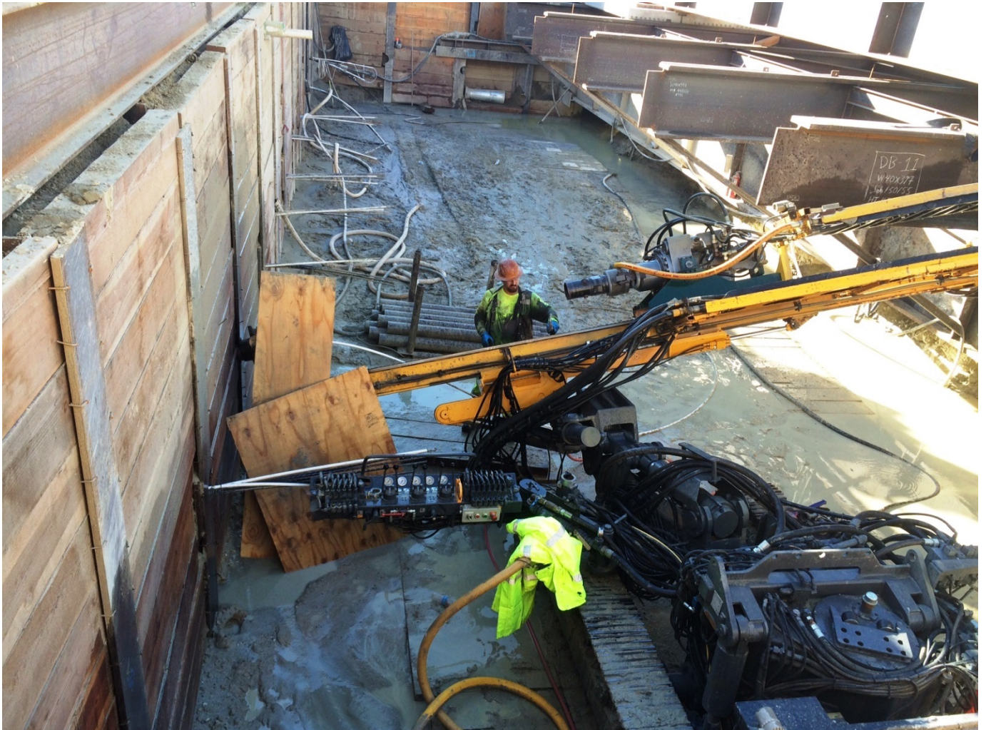
Wilshire/La Brea South Muck Shaft Tieback Grouting
