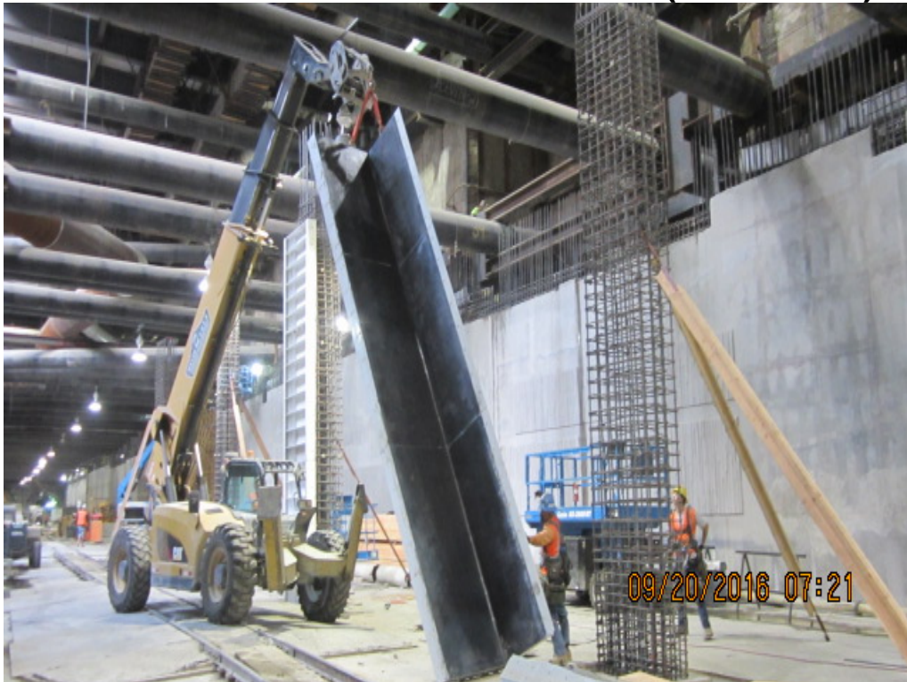
EXPOSITION/CRENSHAW STATION – Installation of rebar and formwork for Invert level column.
