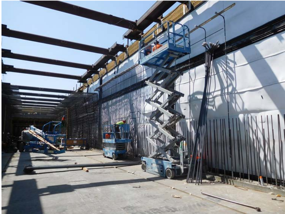
UG#1 – Type 2 strutted U-wall rebar installation.
