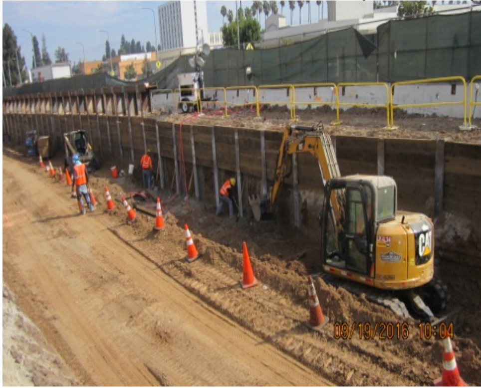
UG#4 –Lagging and excavation activities along the east wall.
