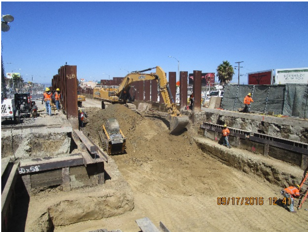
UG#3 – Excavation activities at north portal.
