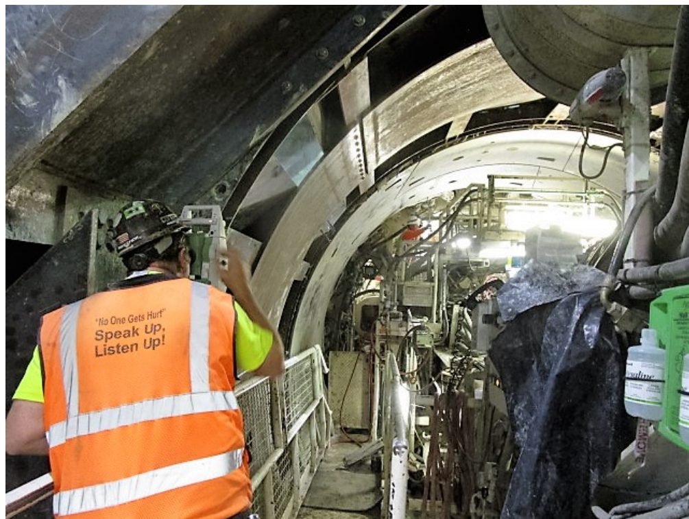
TUNNELING – Installation of ring #693.
