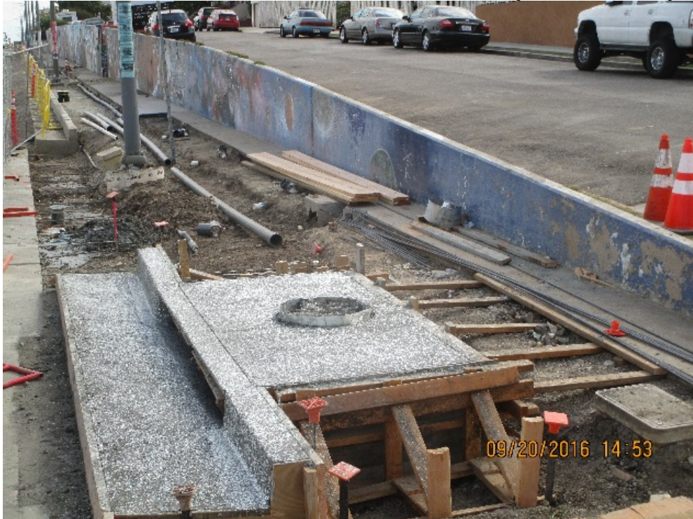
PARK MESA HEIGHTS – Placement of catch basin #25.
