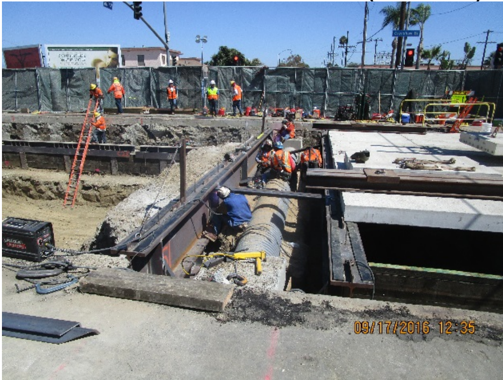
UG#3 – Setting deck beam and deck panels.
