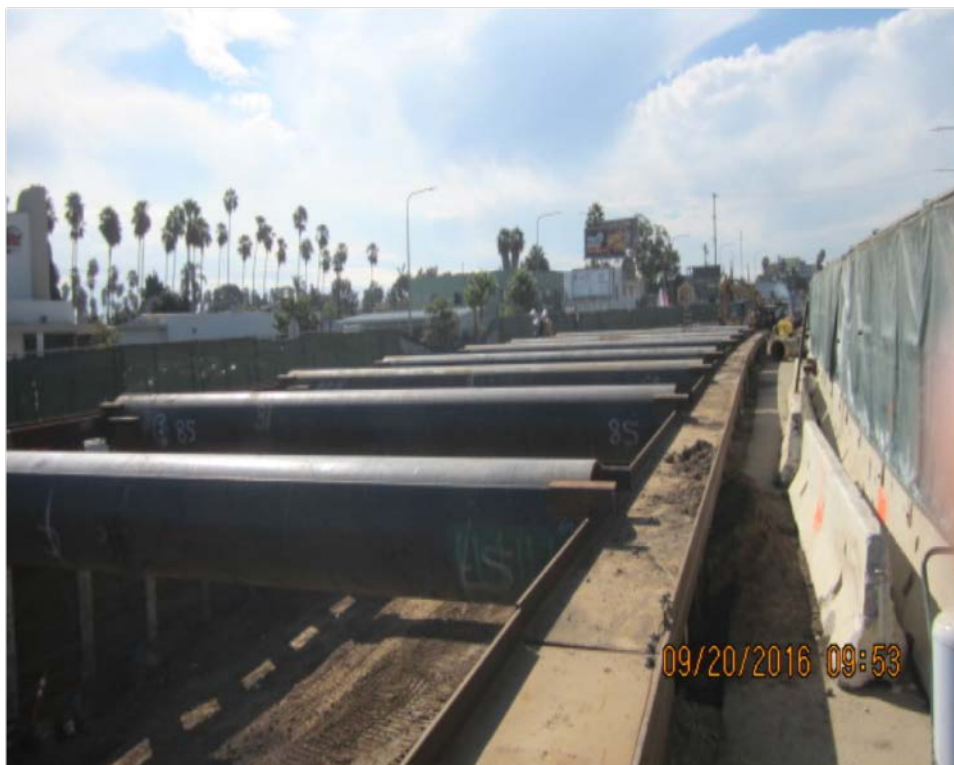
UG#4 – Staging struts at south end of cut and cover.
