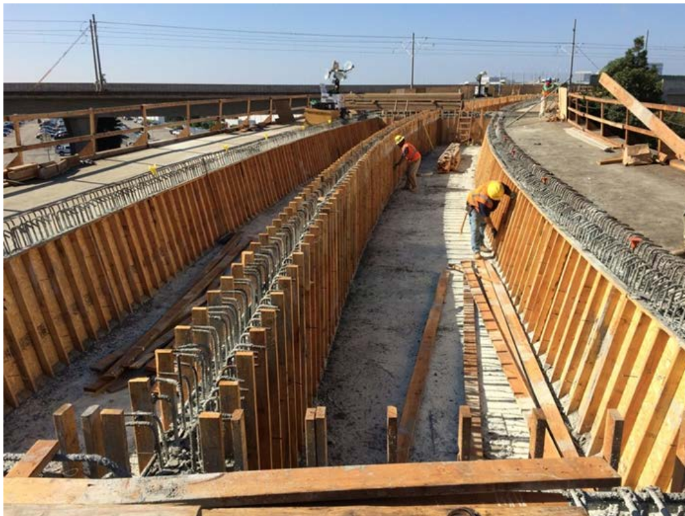
GREENLINE UNDERPASS – Continued with deck formwork at Frame 2.
