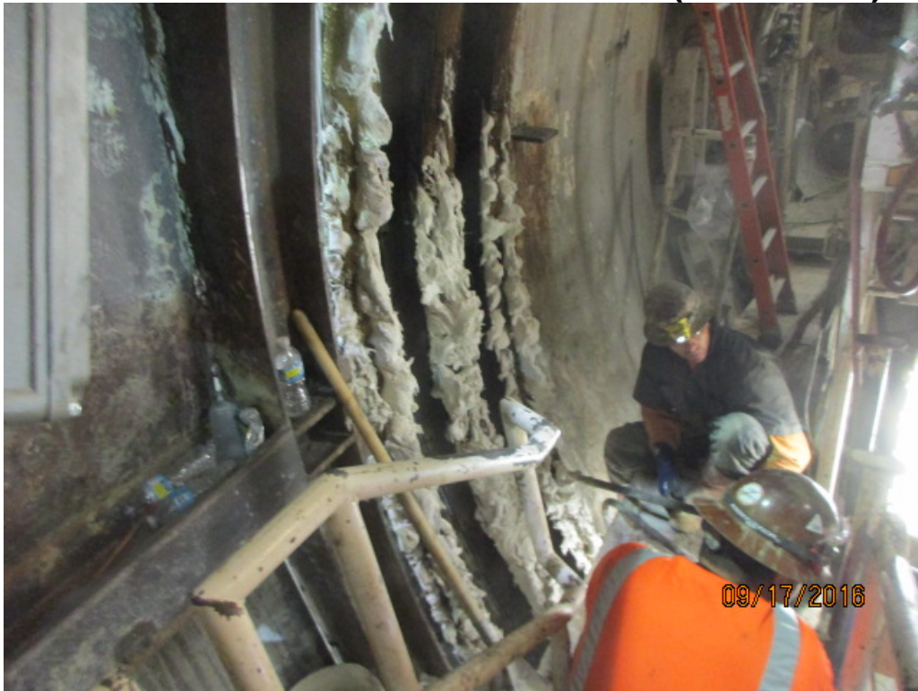
TUNNELING – Greasing tail seal brushes in preparation for continued mining.
