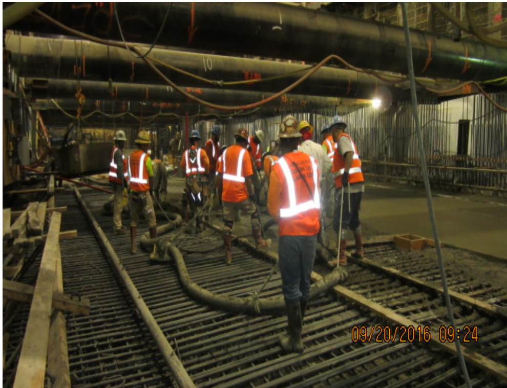
LEIMERT PARK STATION – Placement of invert section C-4.
