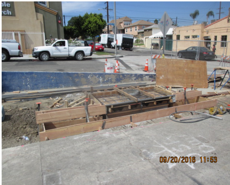
PARK MESA HEIGHTS – Installing formwork for catch basin at Westmount.
