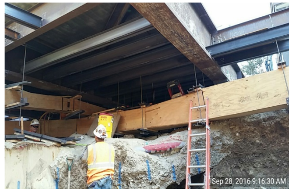
Utility hanging at 2 nd /Broadway
