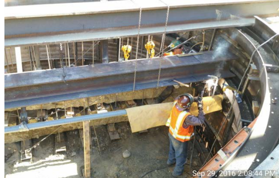
Excavation and utility hanging at Tie-back Removal Pit
