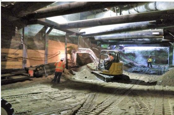
Excavation at Wye
