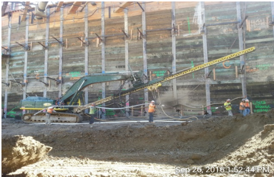
Tie-back installation at 2 nd /Hope
