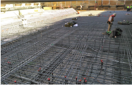
Installation of top map of rebar for 1 st /Central station invert
