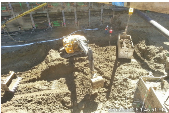
Removing spoils from 2 nd /Hope with muck bin
