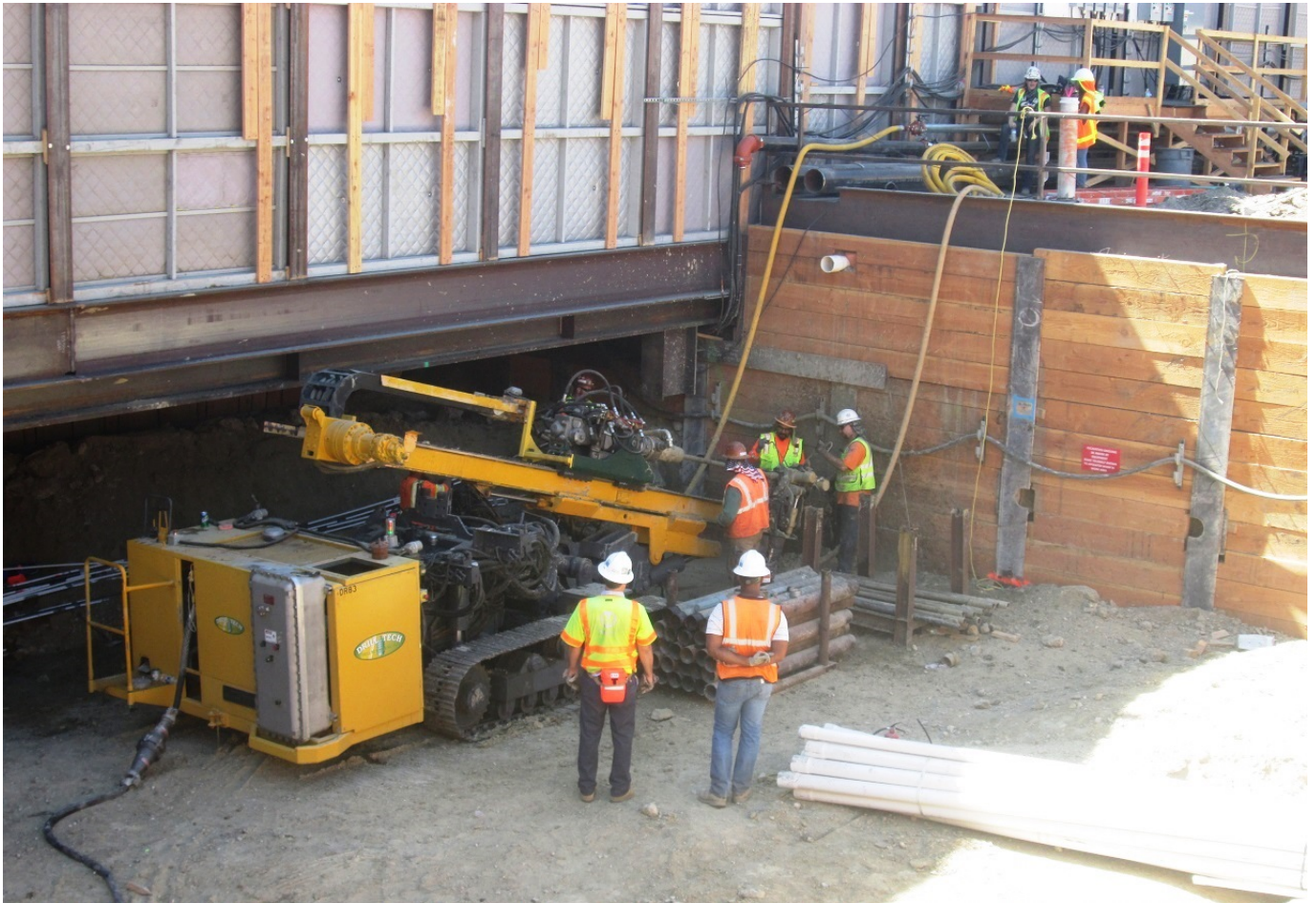
Wilshire/La Brea North Muck Shaft Tieback Installation
