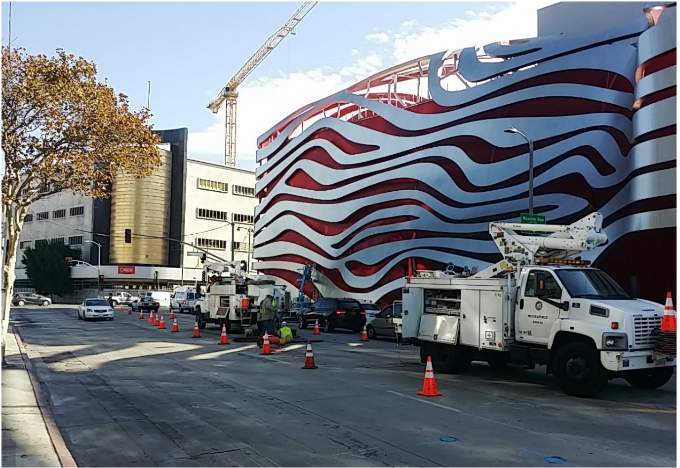
LADWP Performing Power Cutover on Fairfax south of Wilshire Blvd.
