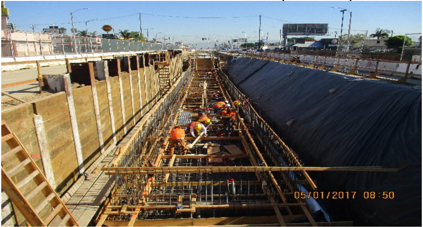
HYDE PARK STATION- Installation of formwork for TC&C room.
