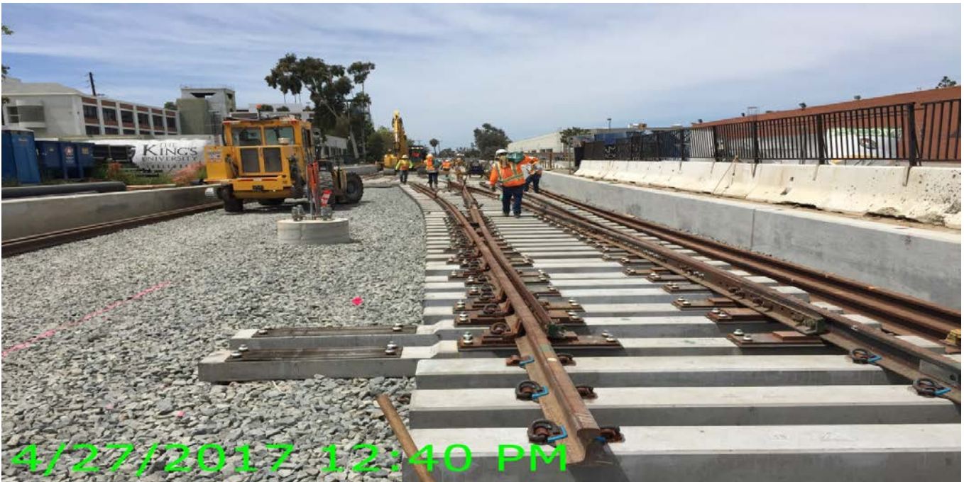
Special ballasted trackwork installation.
