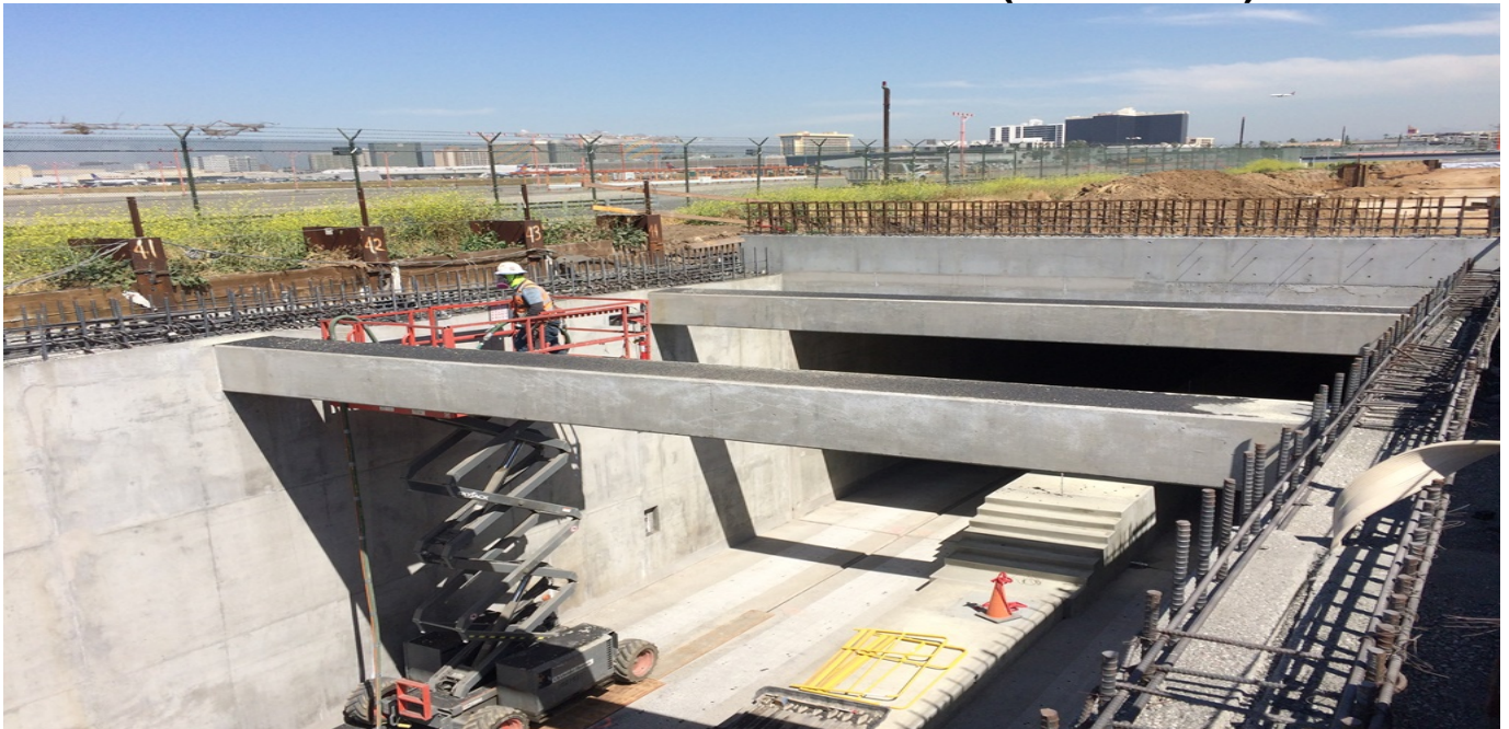
UG1 - Sandblasting underway along the barrier wall construction joint.
