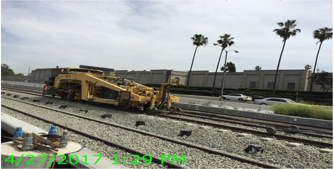
Ballast tamping ongoing.
