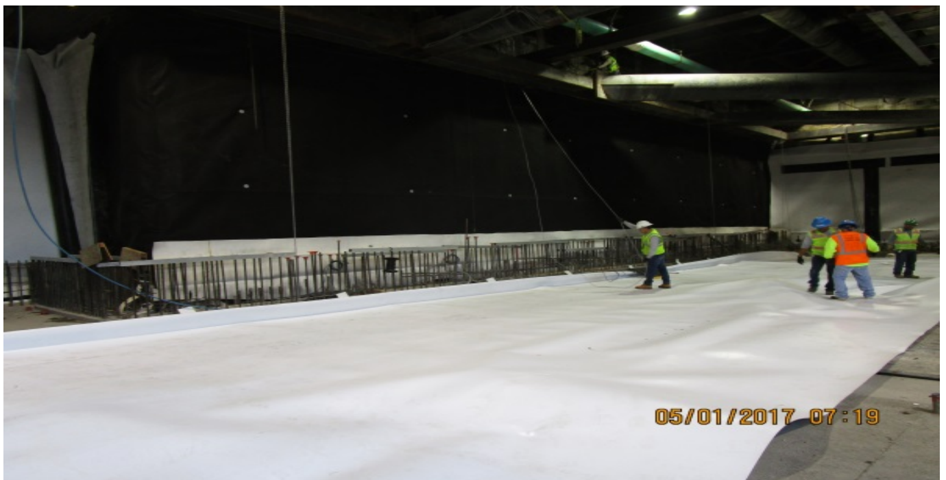
EXPOSITION/CRENSHAW STATION– Preparing to install waterproofing for concourse level walls.
