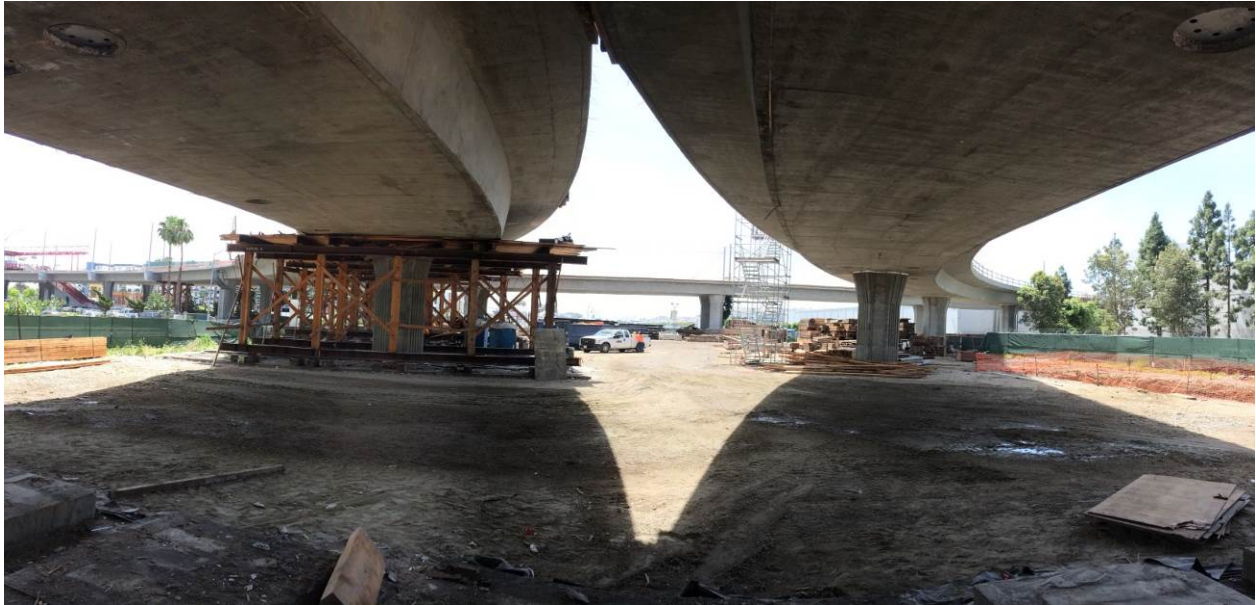
GREENLINE UNDERPASS – Falsework removal underway at frame 1 & frame A (right).
