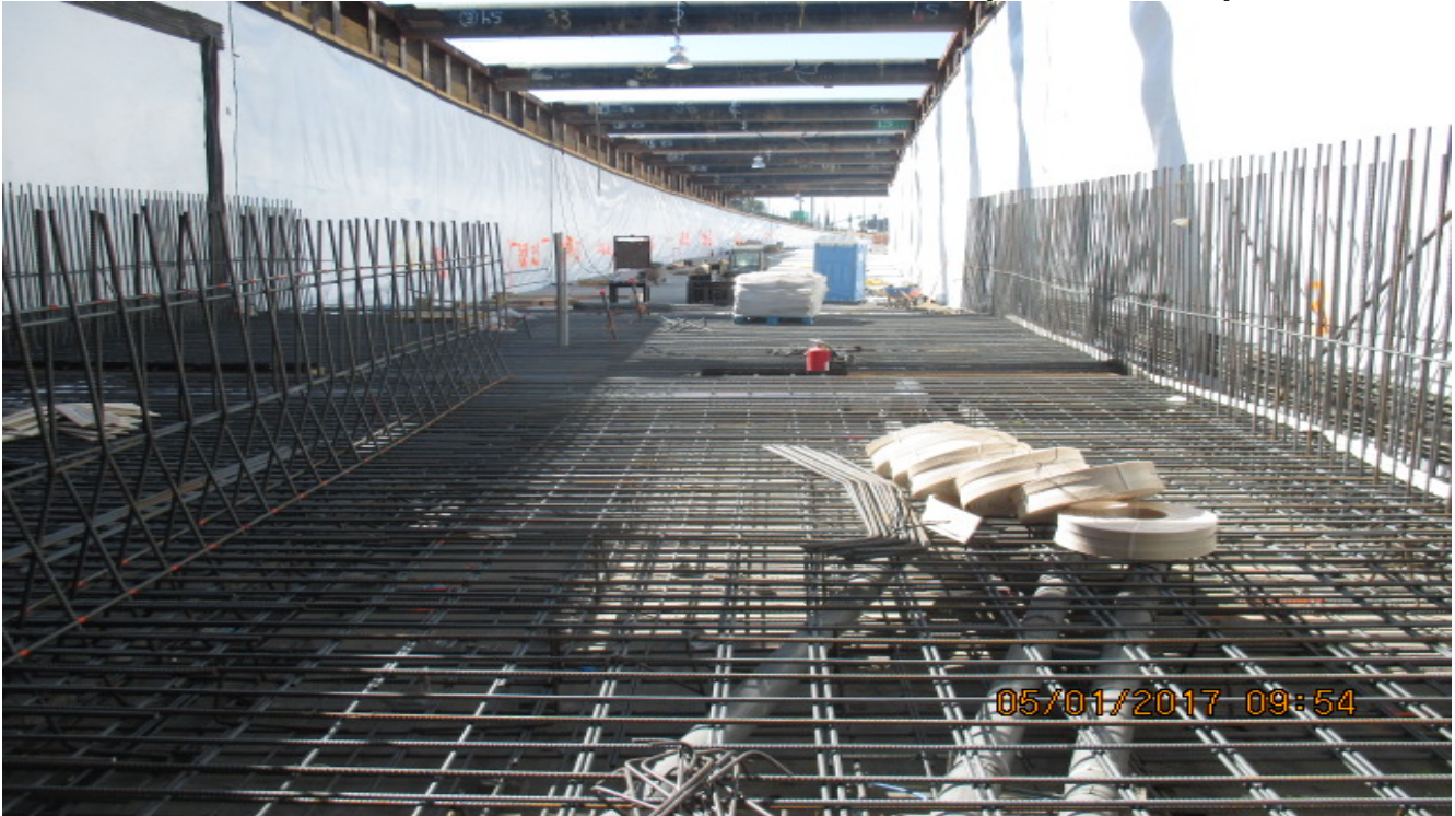
UG4 – Installation of rebar for invert section I-16.
