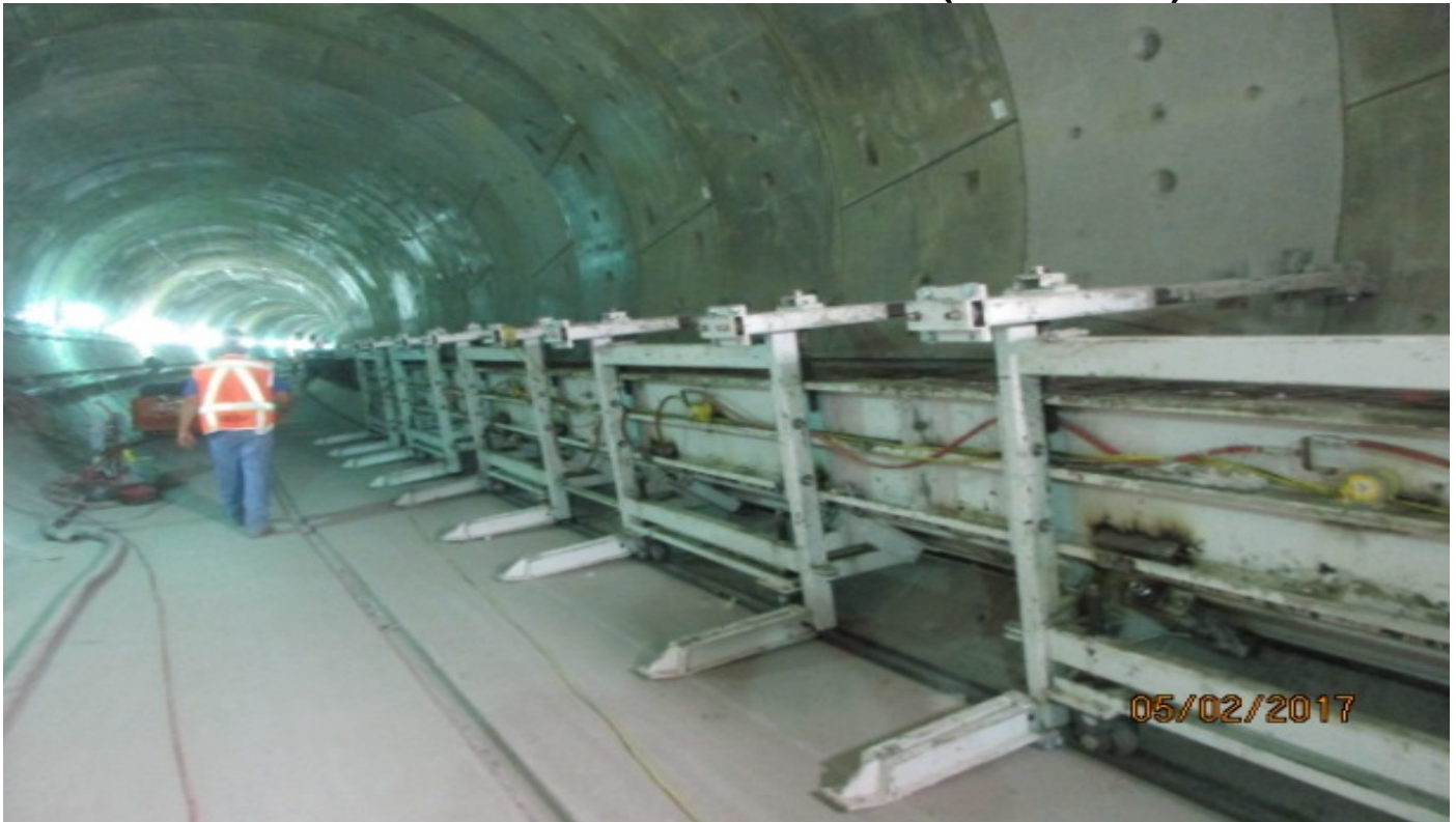
TUNNELING – Installation of SB Tunnel Walkway formwork.
