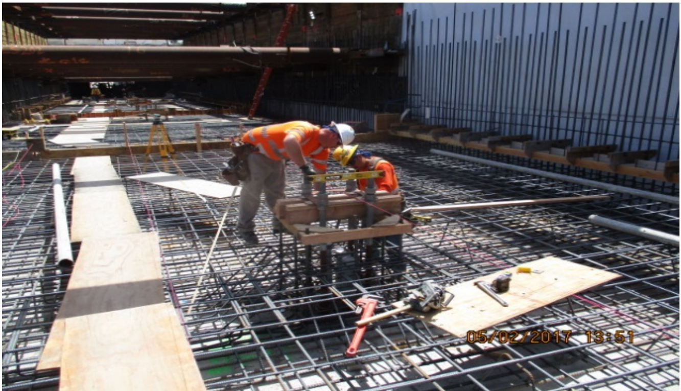
UG#3 Installation of rebar and OCS foundation north of 60th St.
