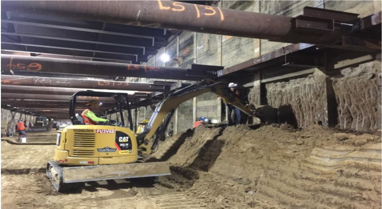
UG#3 – Excavating and lagging activities near Hyde Park Blvd.
