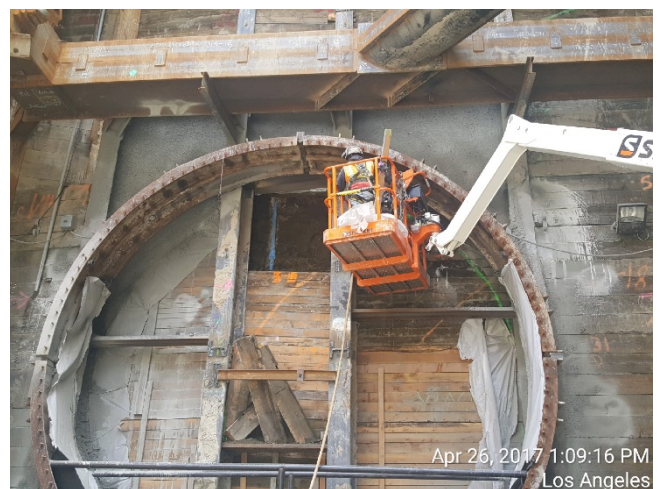
Applying Shotcrete at Left Track at Hope Station
