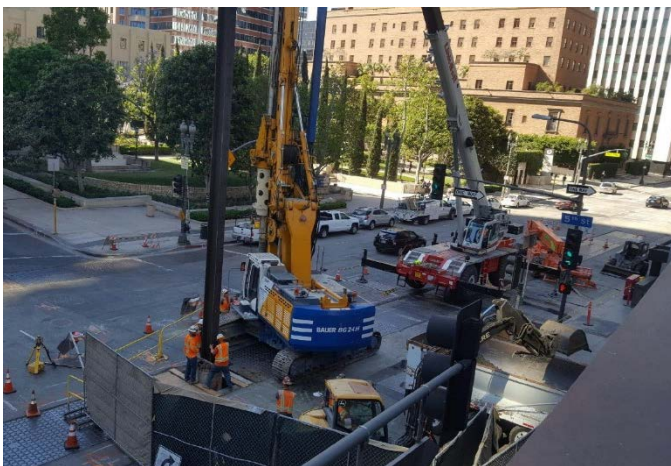
Piling at SW corner of 5th & Flower St.
