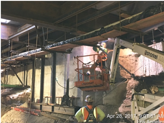
Utility Hanging along north side of Broadway SOE
