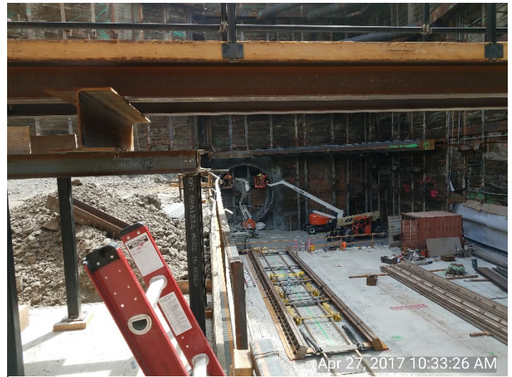
Installed Temporary Rail for TBM at Hope Station
