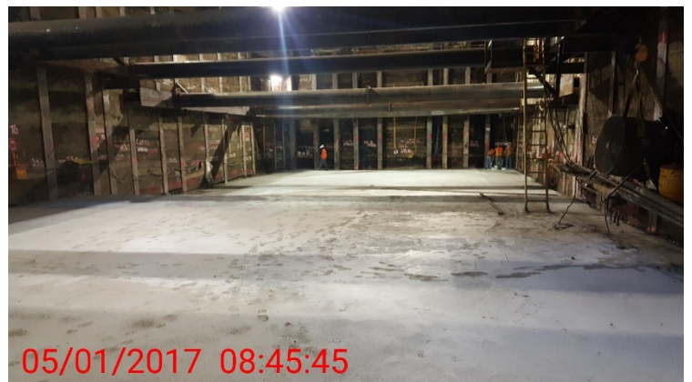
Finished Sub-Invert slab at TBM Retrieval Shaft
