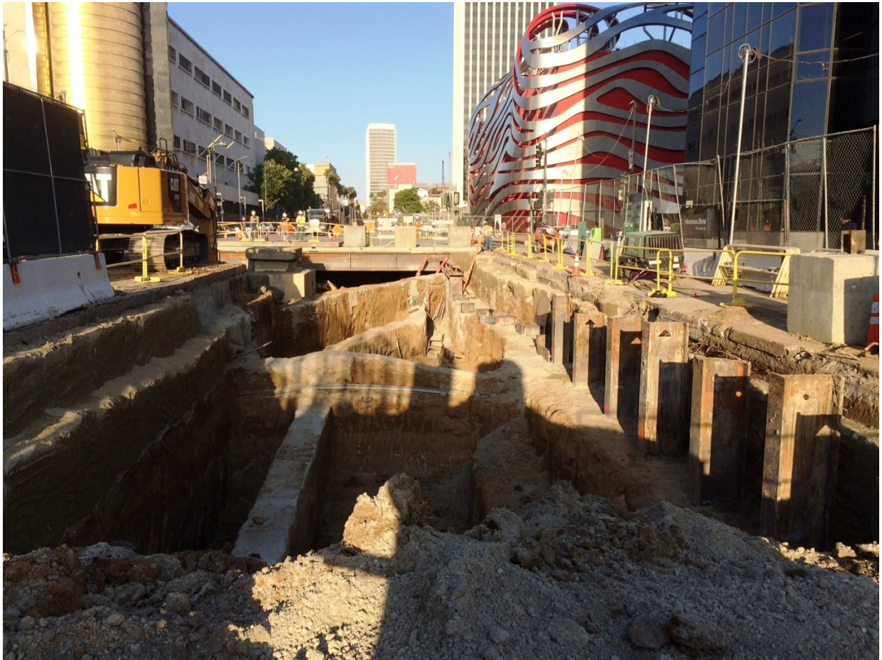
Wilshire/Fairfax Decking Operation in Progress
