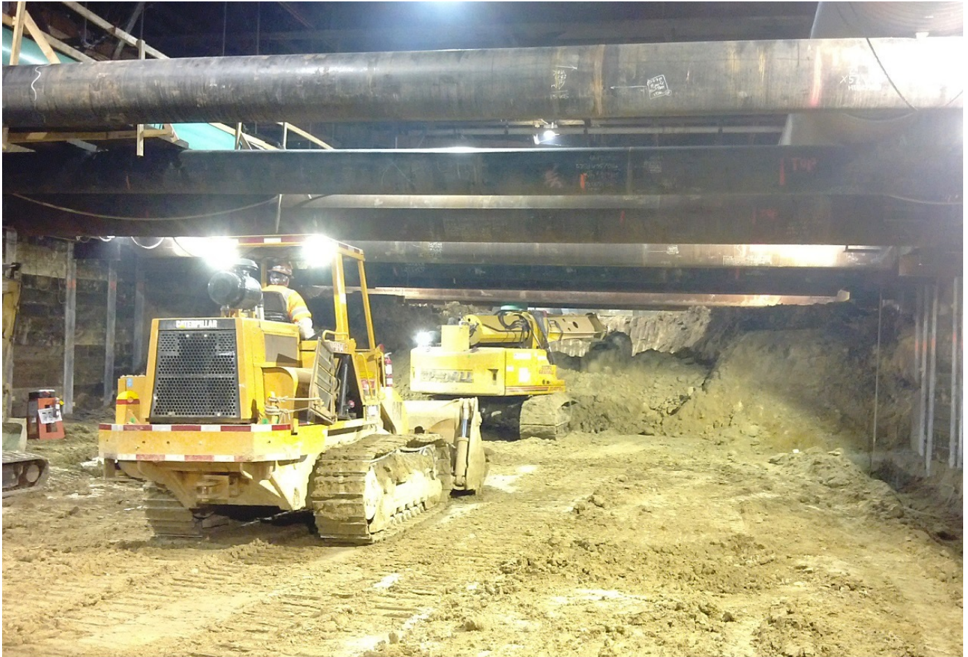
Under Deck Excavation at Wilshire/La Brea Station
