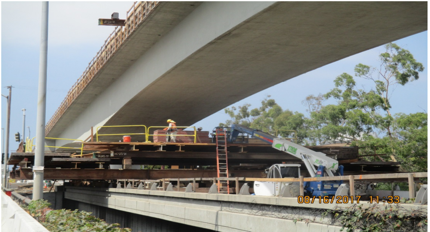
(AG-5) I-405 BRIDGE – Falsework removal complete.
