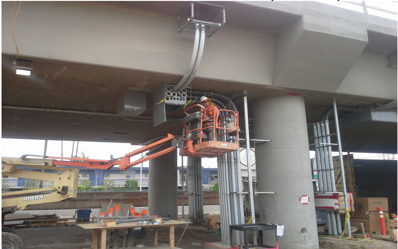
AVIATION/CENTURY BRIDGE – TPSS #2 and TC&C #3: Site work underway.
