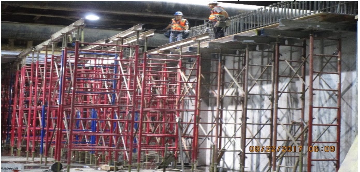
EXPOSITION/CRENSHAW STATION – Installing roof support falsework at Roof Slab Phase 1.
