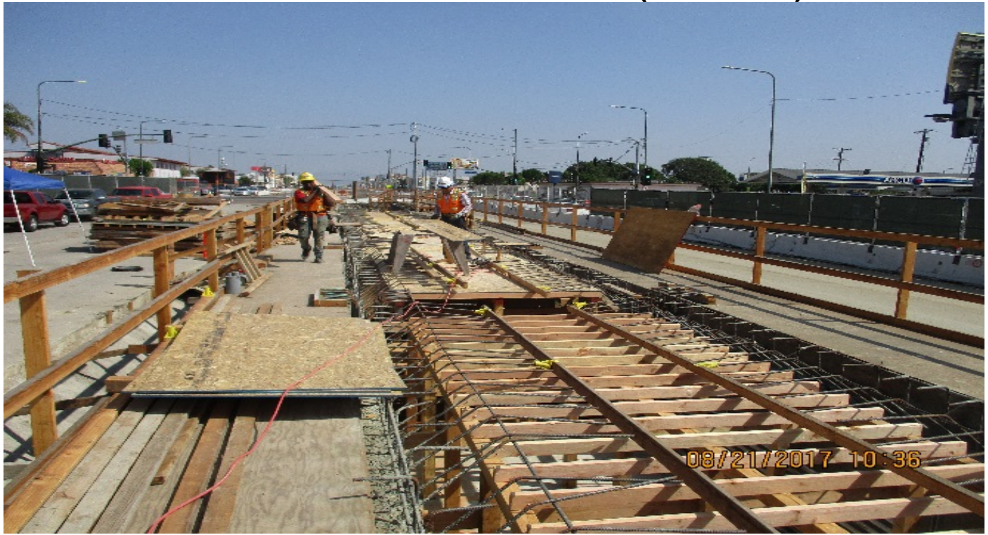
HYDE PARK STATION- Installation of formwork for platform deck.
