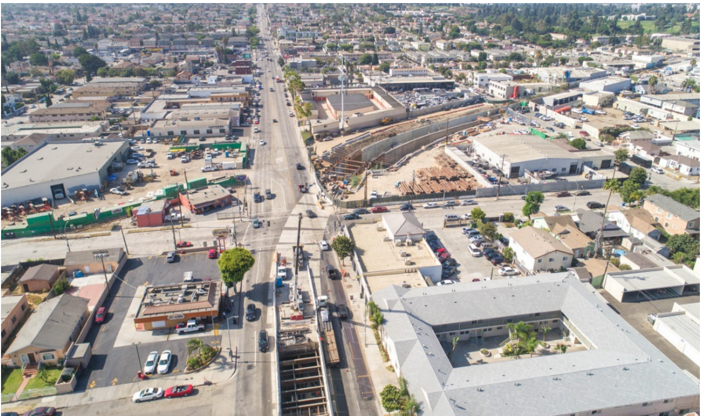
UG#3 - Aerial view of the south end of UG-3.
