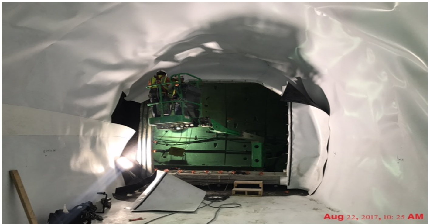
TUNNELING – Installation of waterproofing at CP-2.
