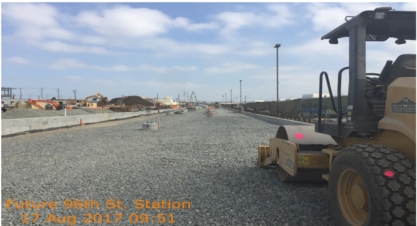
ACCOMODATIONS FOR 96TH STREET STATION AREA – Bottom ballast placement complete.
