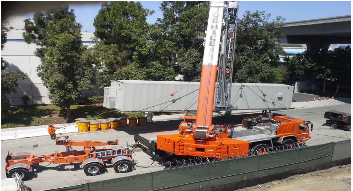
GREENLINE UNDERPASS TC&C #1 building set.
