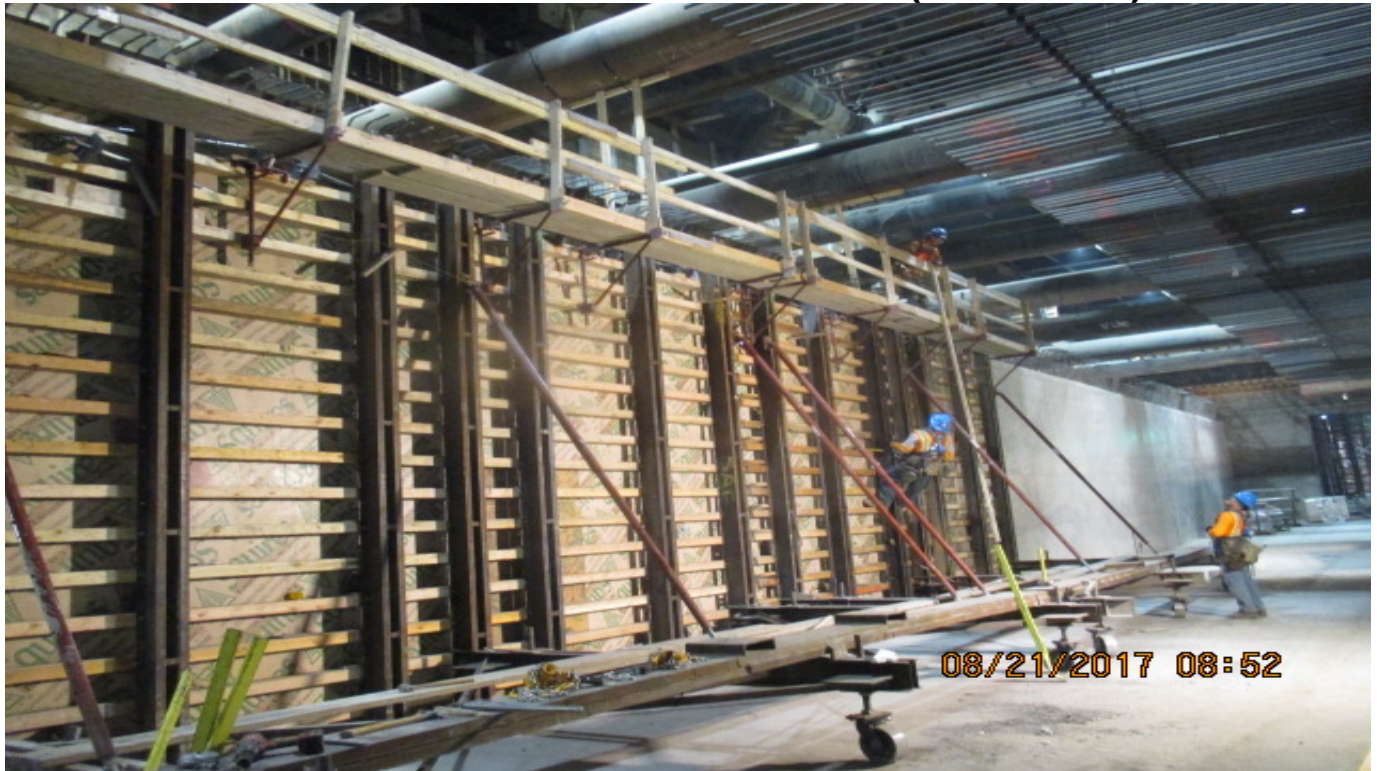
UG4 – Removing formwork for completed wall section CW-26.
