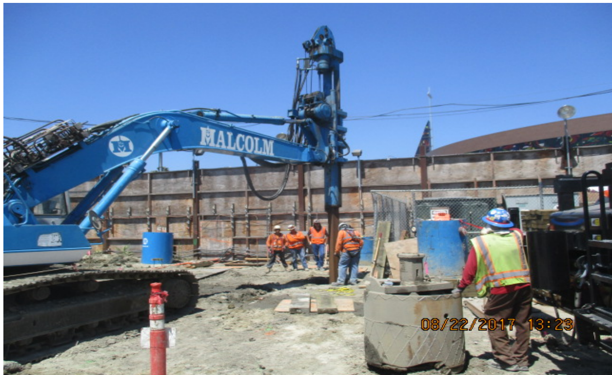
EXPOSITION/CRENSHAW STATION – Drilling for piles at side structure “Q”.
