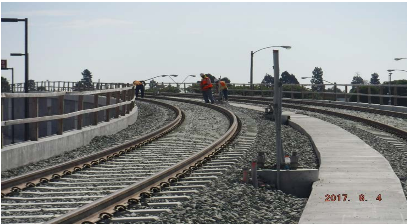
MSE 192 - Wall complete, ballasted trackwork in-place (surface & line and de-stressing complete).
