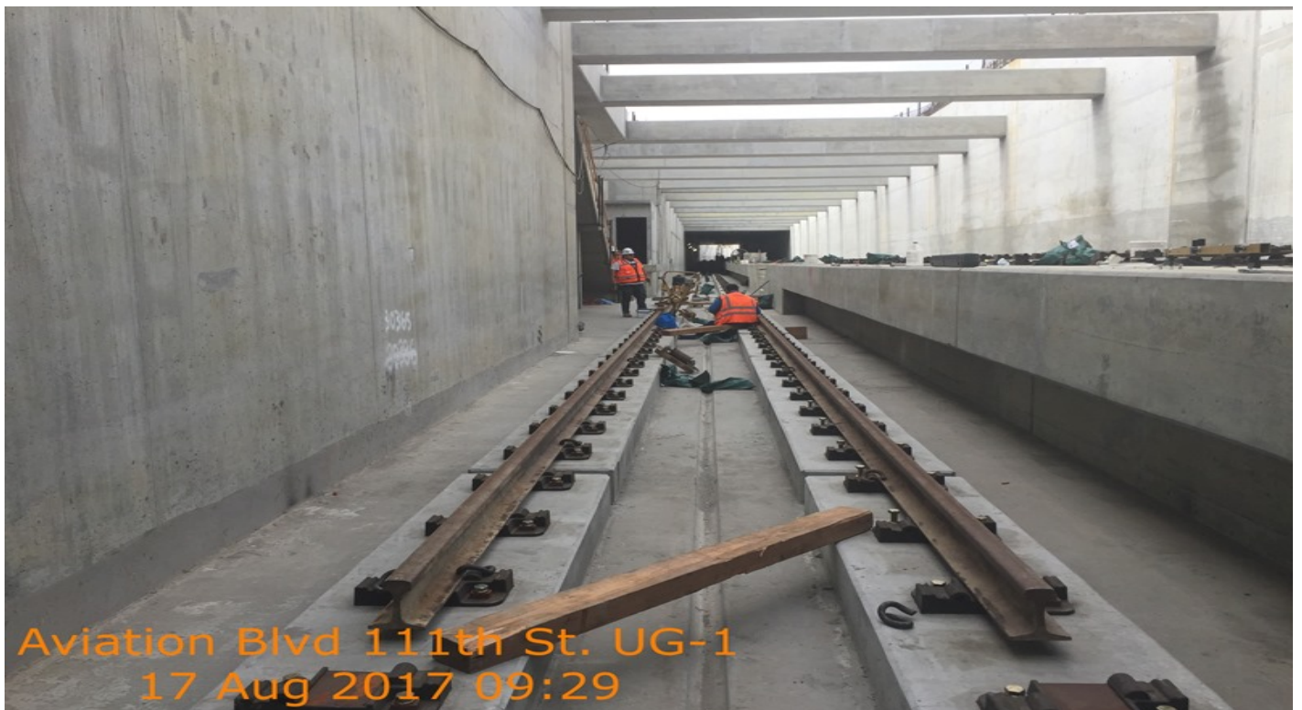
UG#1 - Rail fastener lining and gauging underway.
