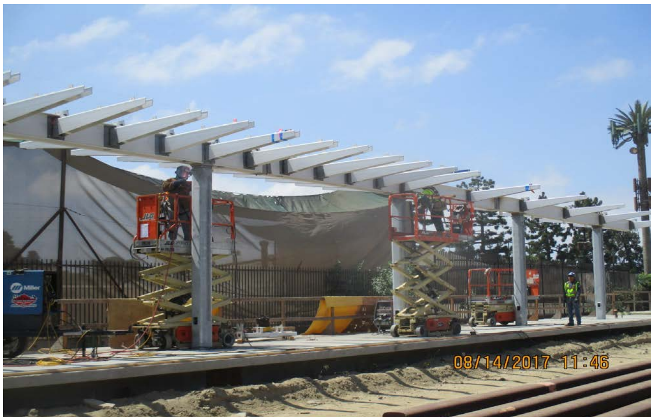
WEST STATION - Canopy erection underway. MEP installation and painting to follow.
