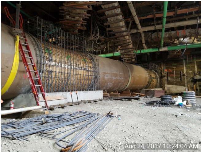
Hobas east bend rebar cage forming at Historic Broadway Station
