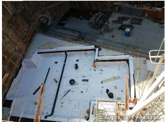
HDPE and waterbar installation at Grand Av Art/Bunker Hill Station
