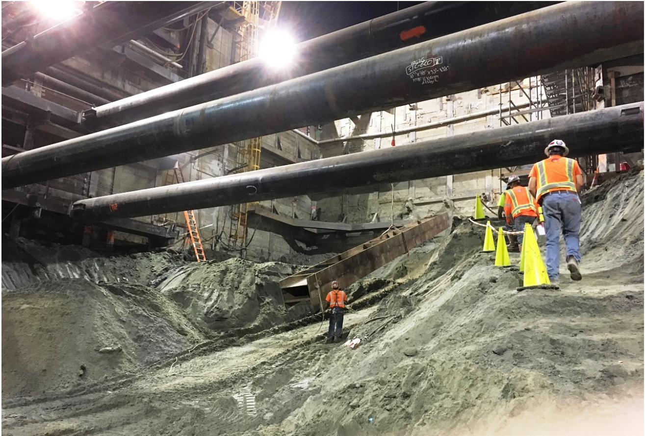
Under Deck Excavation at Wilshire/La Brea Station
