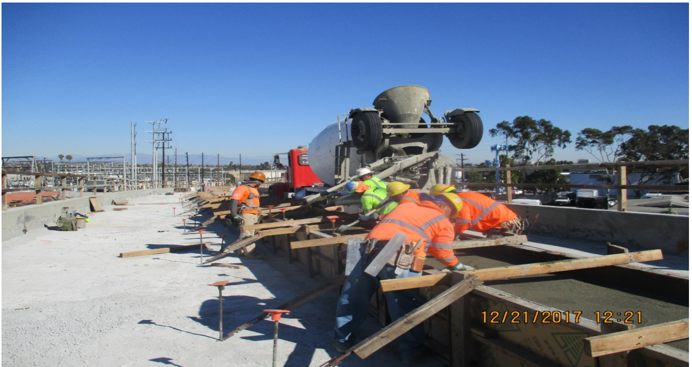
MSE 122 L&R - Electrical ductbank forming over lightweight cellular concrete fill.
