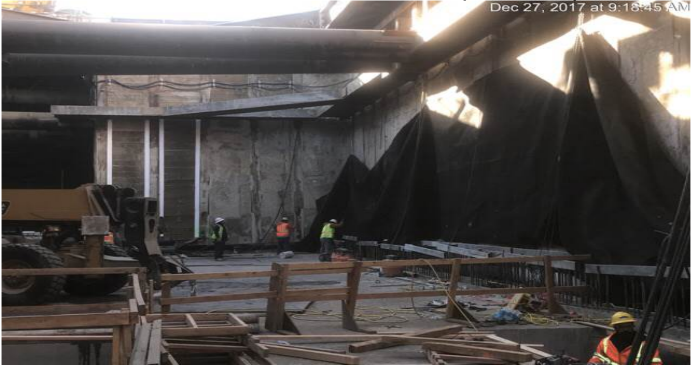
MARTIN LUTHER KING JR. STATION – Installing waterproofing along the west concourse level walls.
