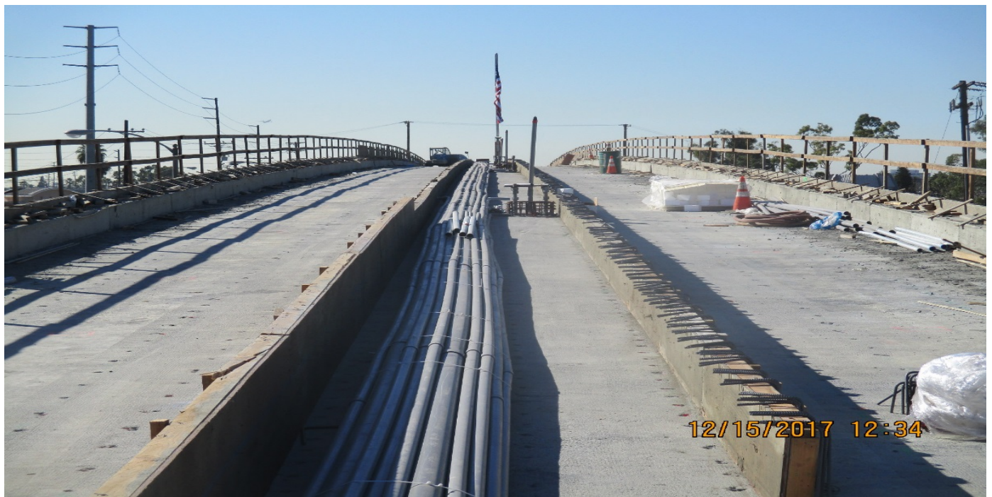
(AG-5) I-405 - Overview of electrical ductbank forming.
