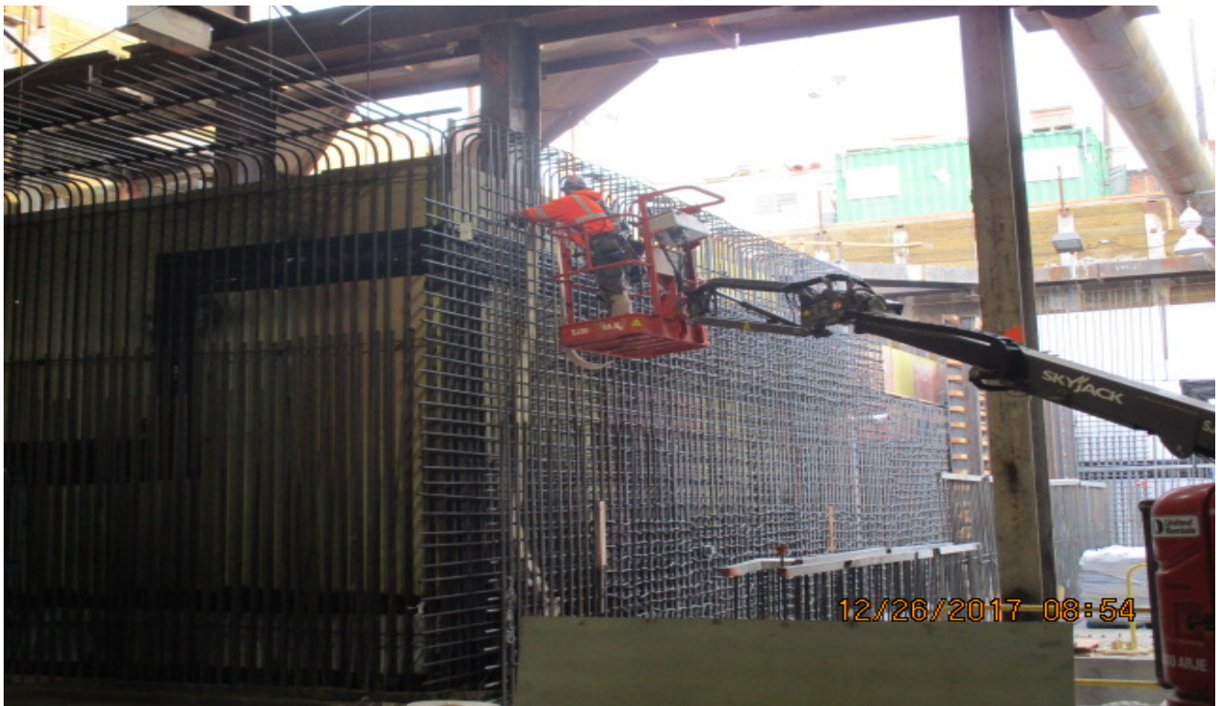
LEIMERT PARK STATION – Installation of rebar at concourse level walls.
