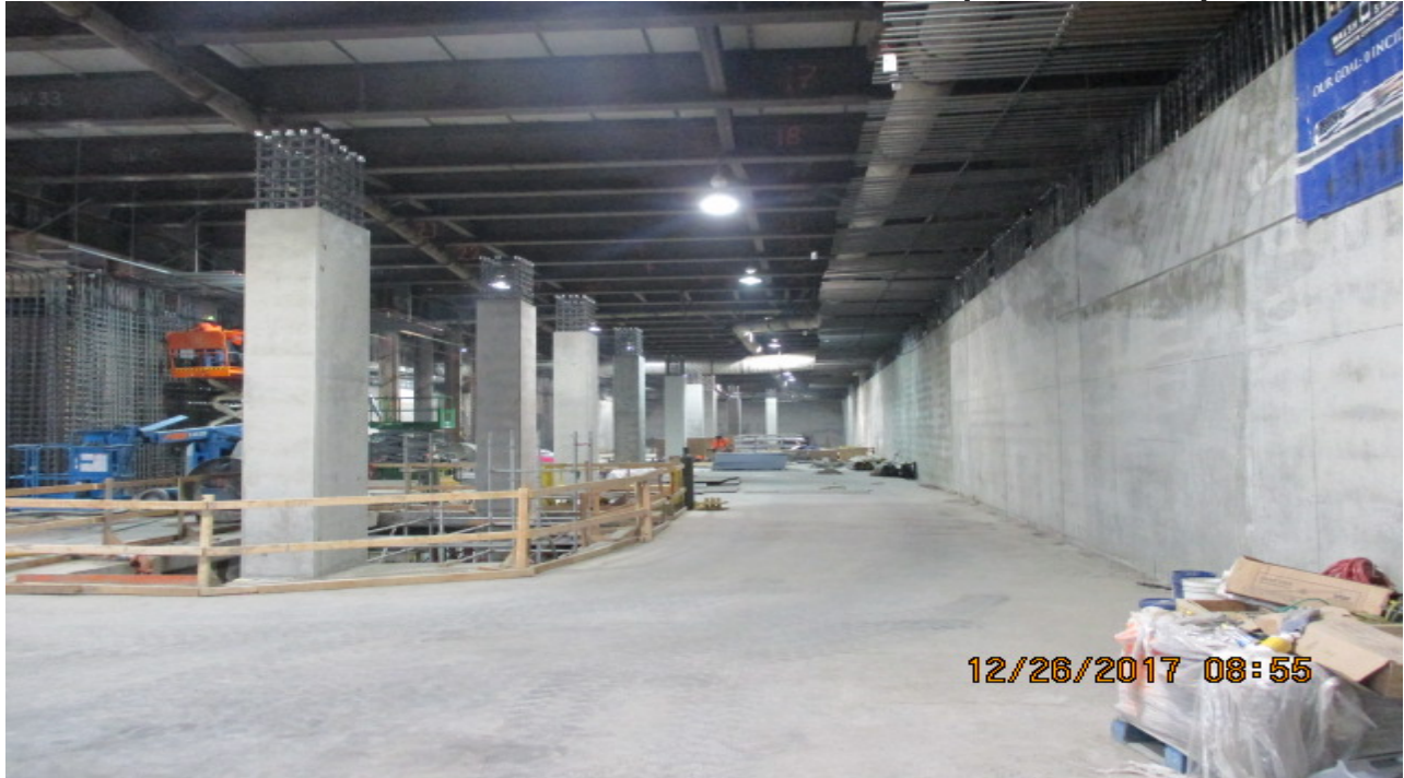
LEIMERT PARK STATION - Previously placed concourse level columns and walls.
